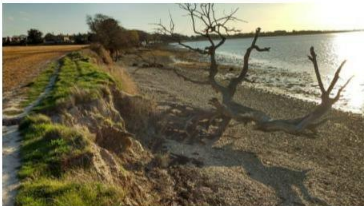
Photo f: Active coastal erosion along the coastal footpath at northern end of H34C facing south on the west shoreline (24 th March 2019)
