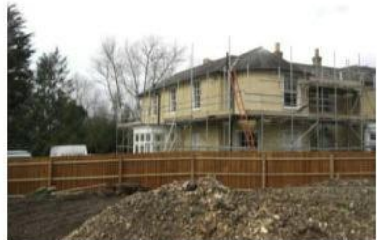
The spoil towards the east elevation
