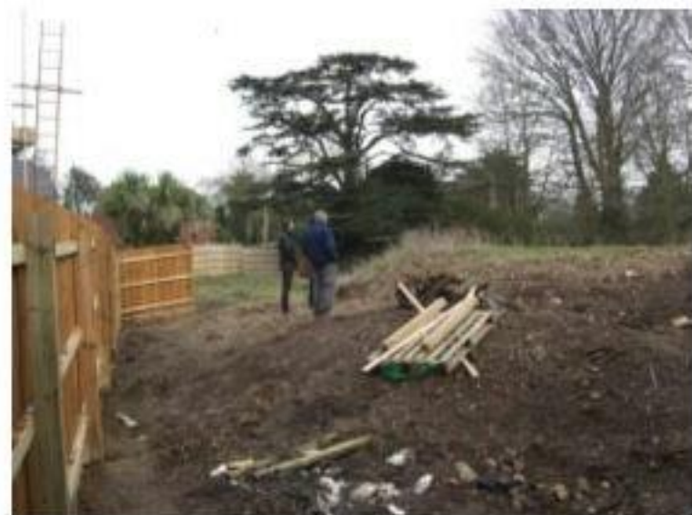
Behind the fence – the southeast site portion
