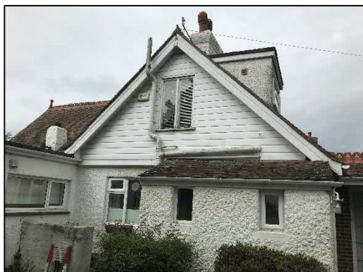
Figure 5: Main residential property with pitched roof
