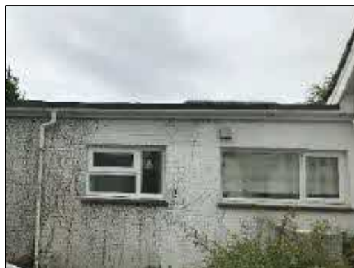
Figure 6: Flat roof section of the property
