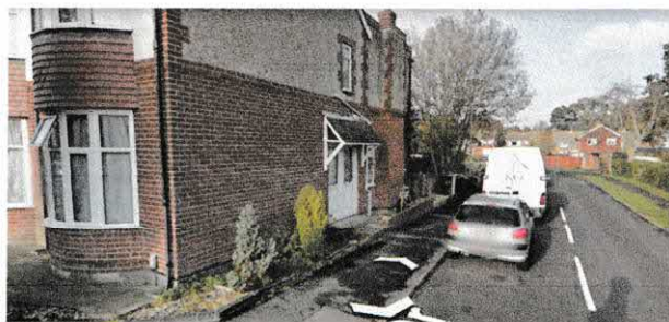
17A/B AVONDALE ROAD - East elevation looking North
