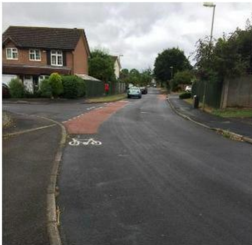
Photograph 2: Westbourne Avenue Existing Conditions
