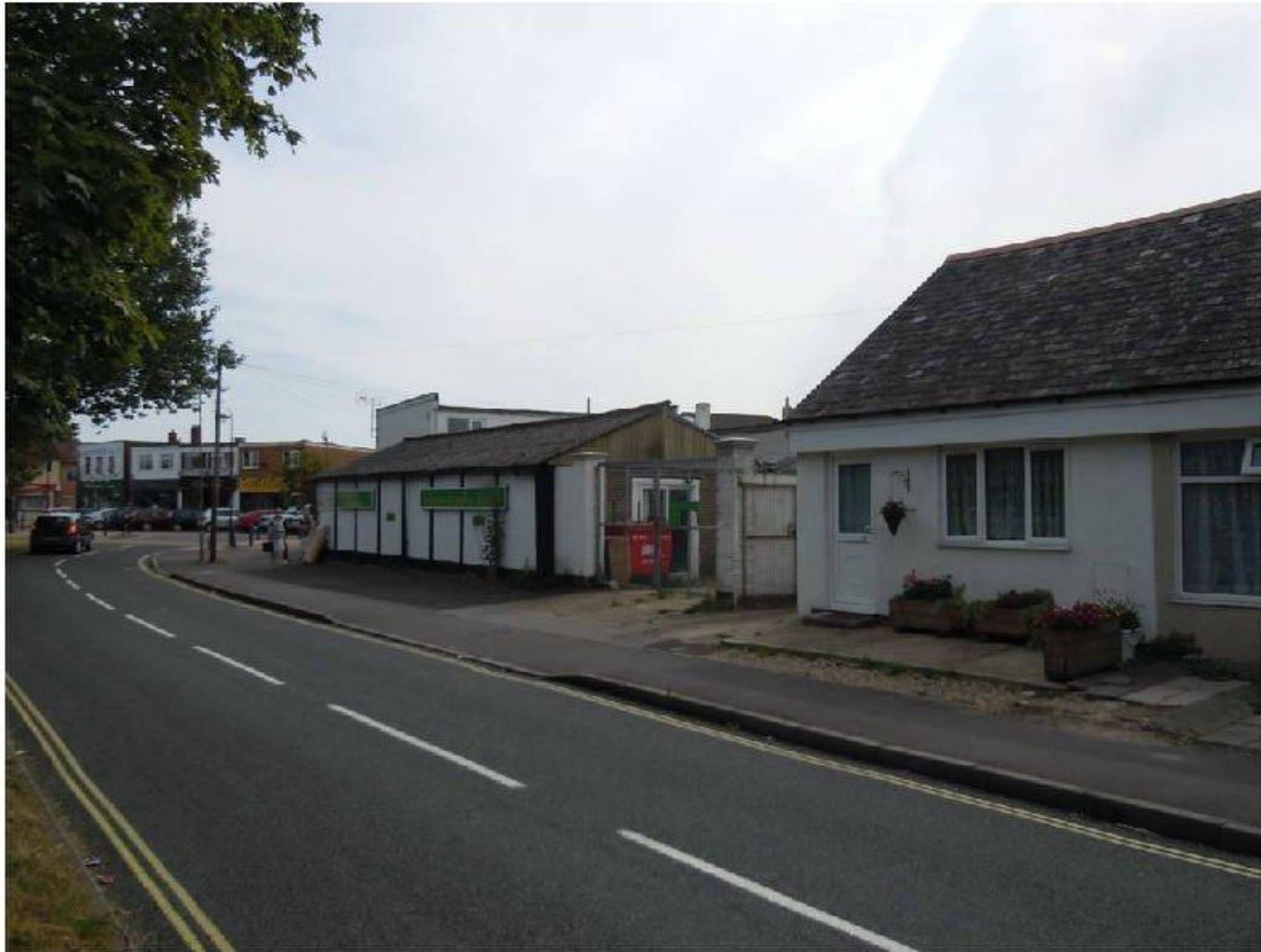
Side workshop from West Lane looking southwest
