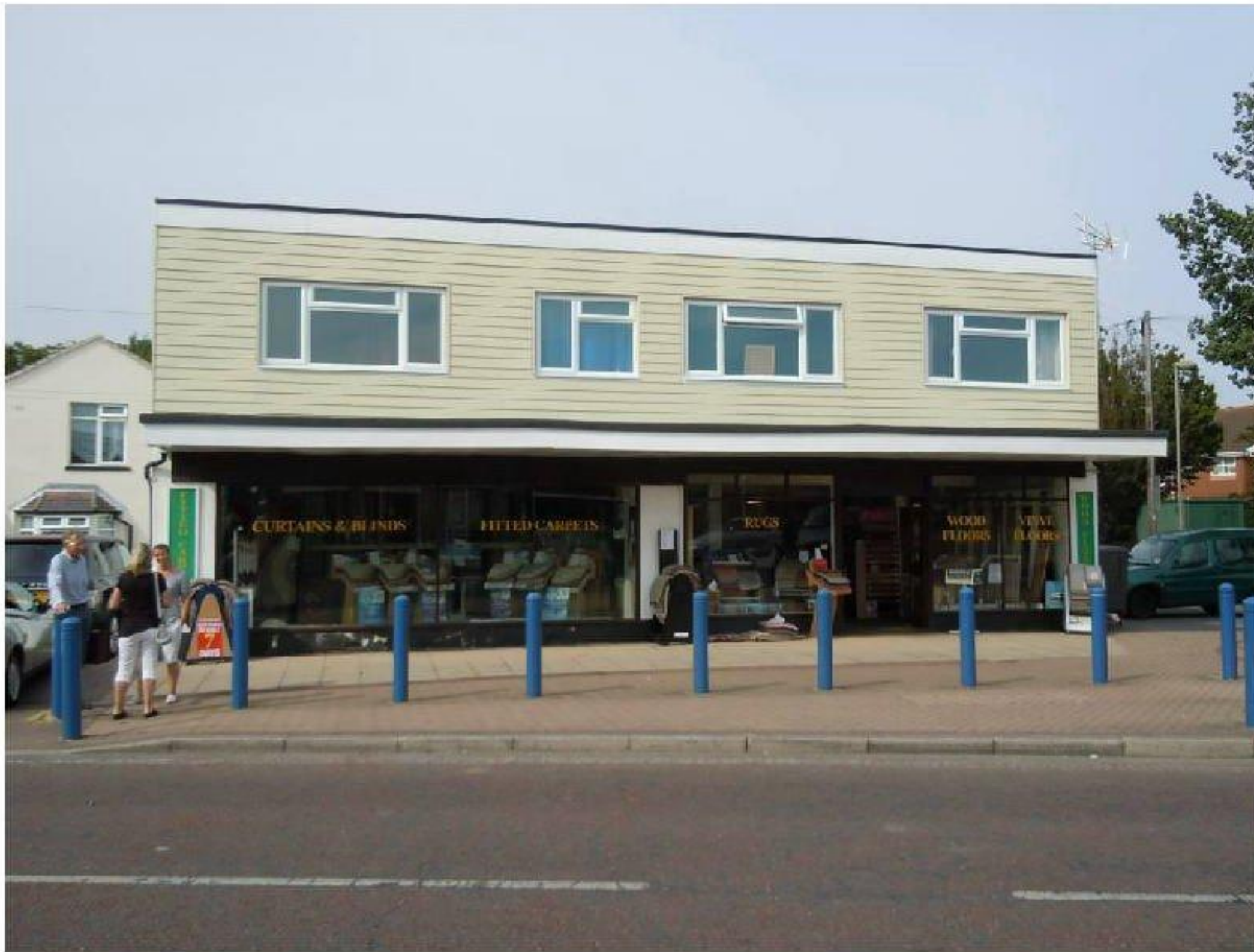
Shop frontage facing Station Road
