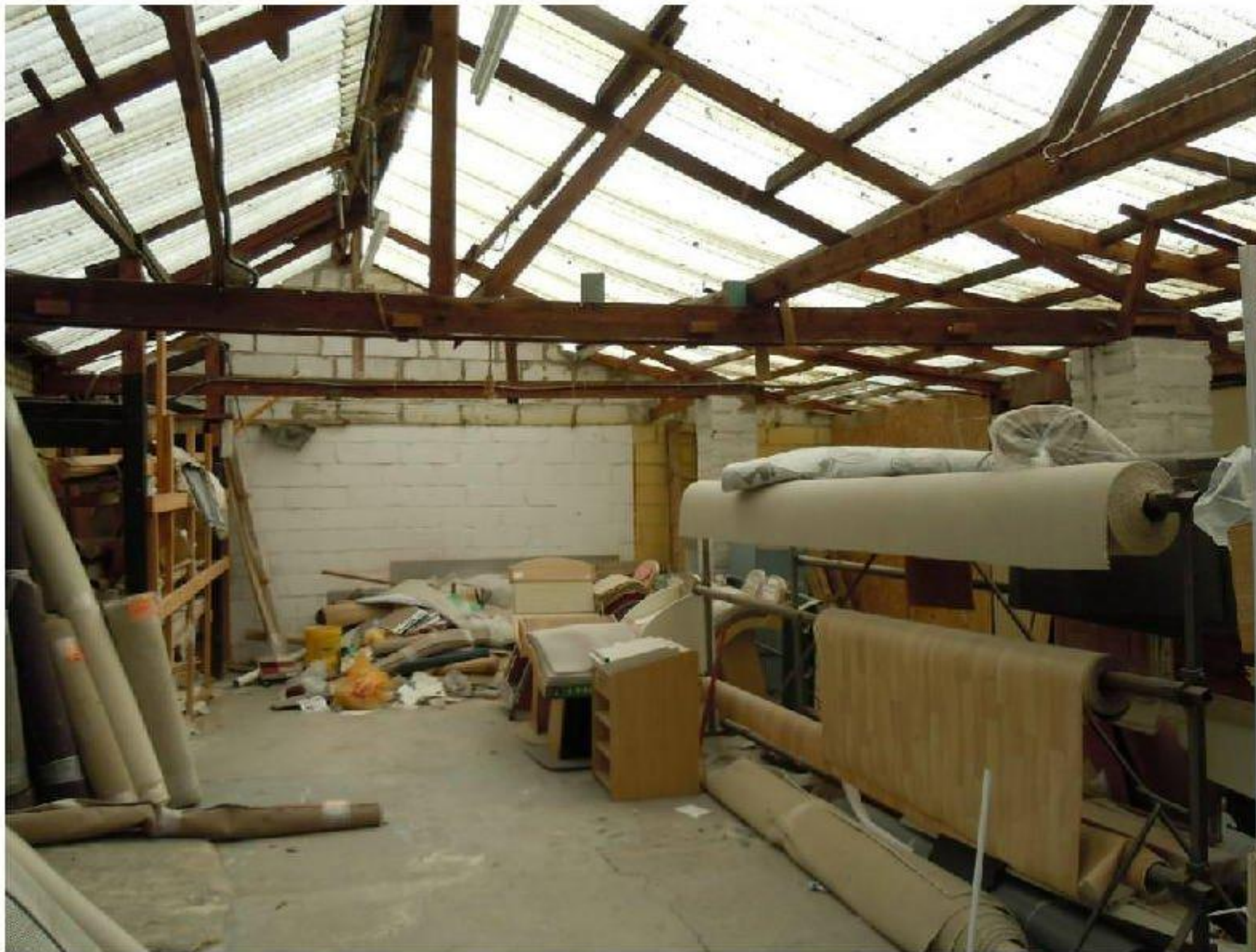
Inside rear workshop
