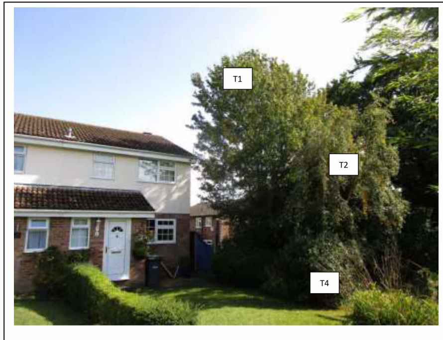
View of property from front left
