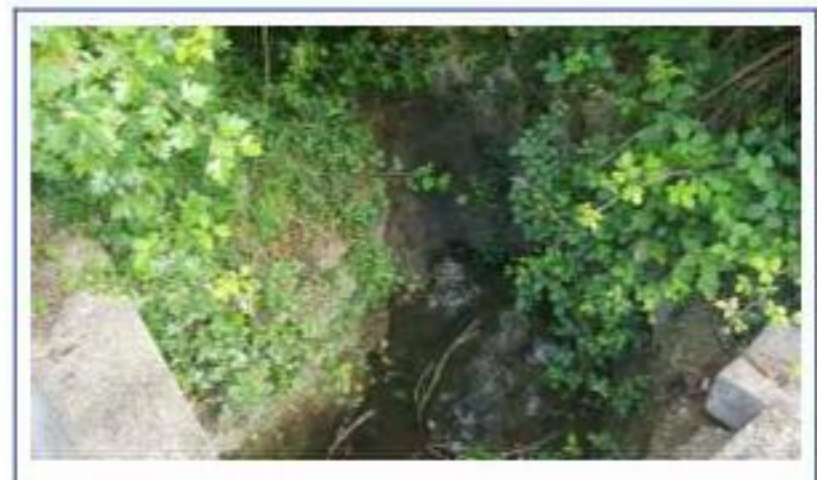
Southleigh Stream at culvert
