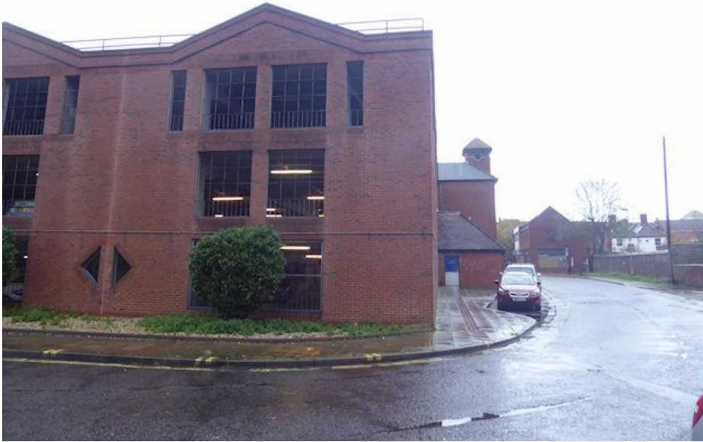
Photograph 9 – General view of the southeast corner of the building.
