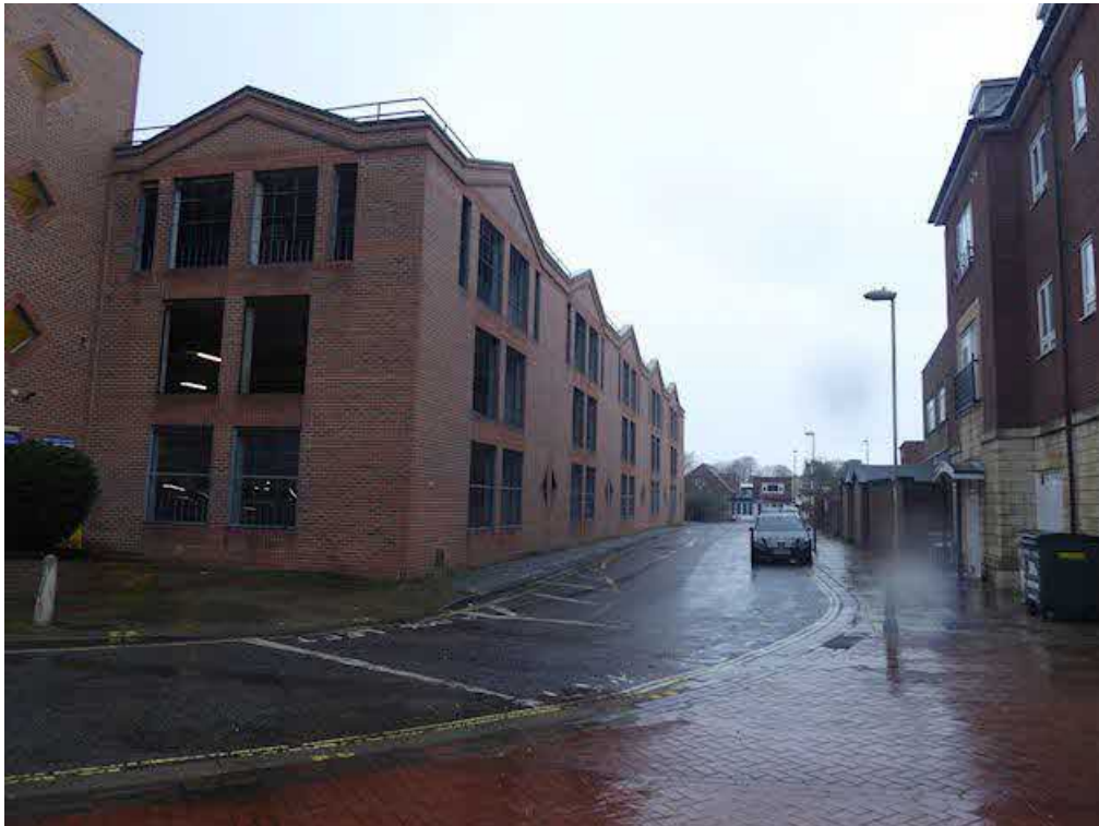
Photograph 19 – General view looking west along Bulbeck Road, noting the north elevation.
