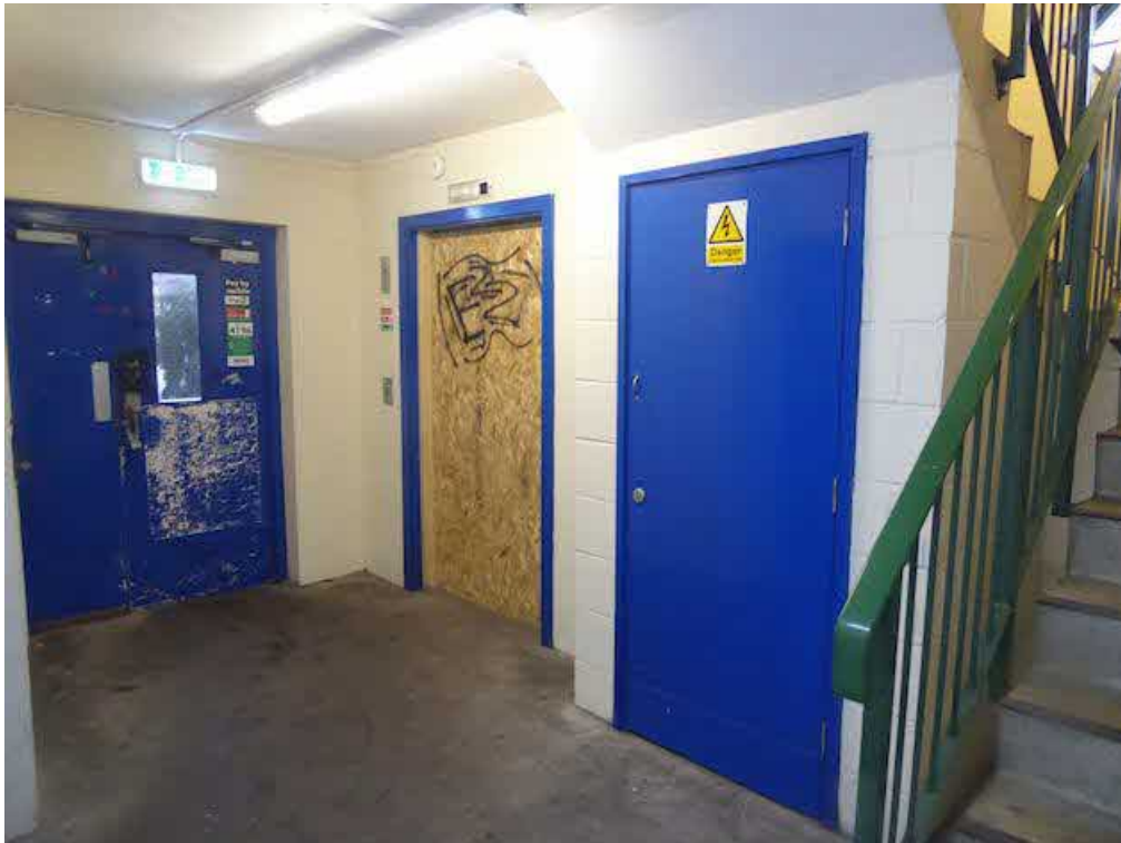
Photograph 27 – General view of the northeast core.
