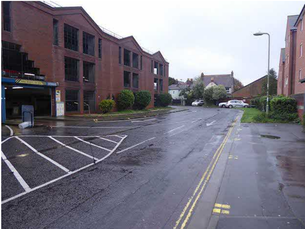
Photograph 5 – General view looking east up Bulbeck Road, with the south elevation.
