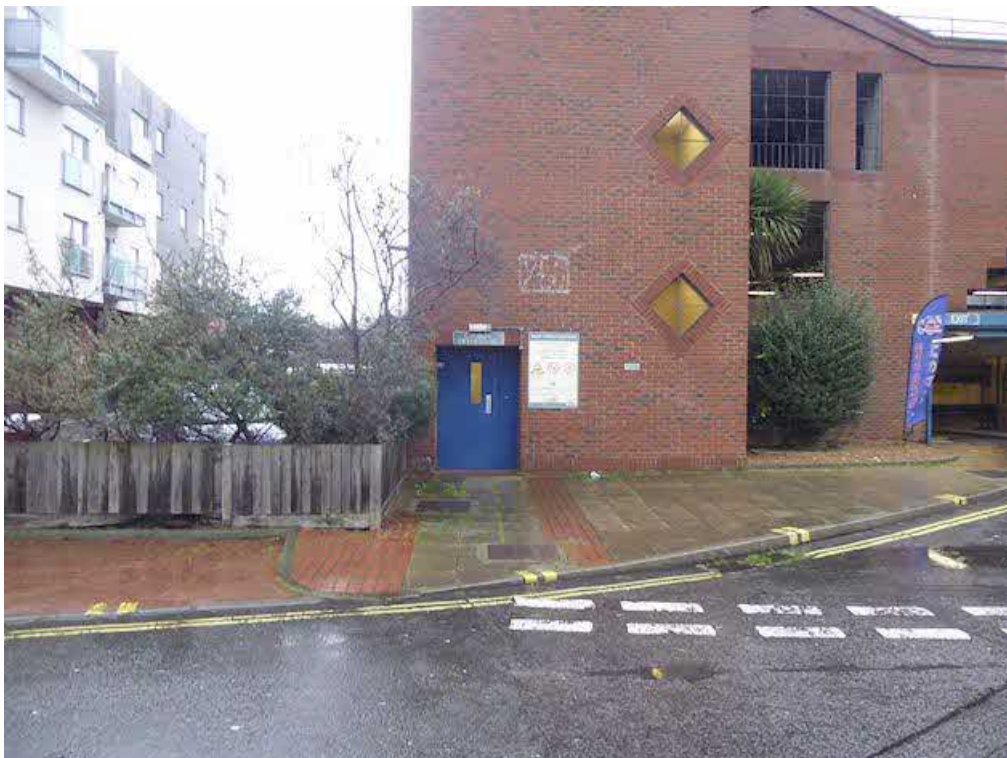
Photograph 4 – General view of the door into the southwest stair tower.
