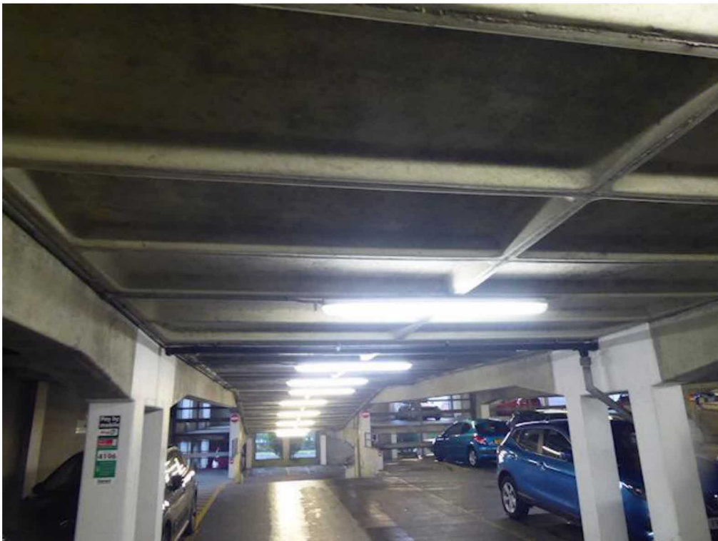
Photograph 32 – View of the structure on the lower decks.
