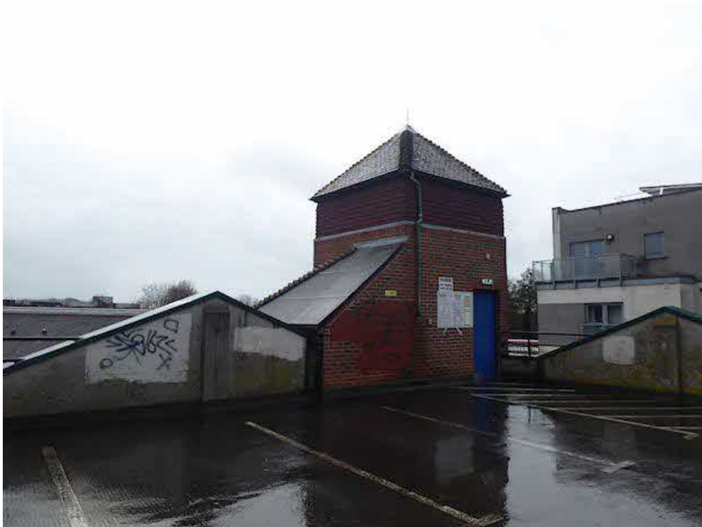
Photograph 49 – View of the southwest stair tower from the top deck.
