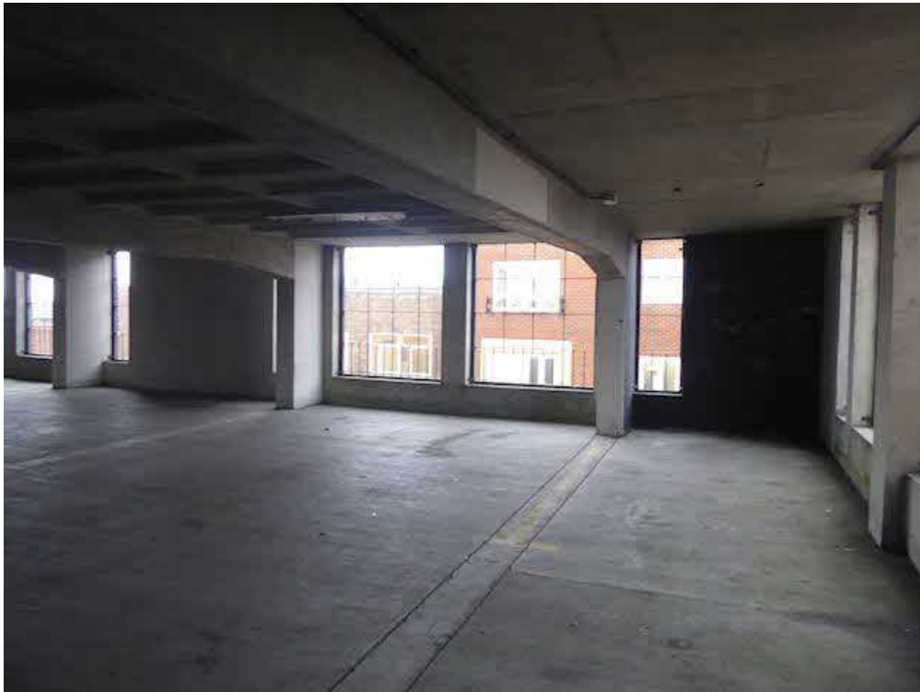
Photograph 41 – Further view of the structure on the top deck, adjacent to the external wall.
