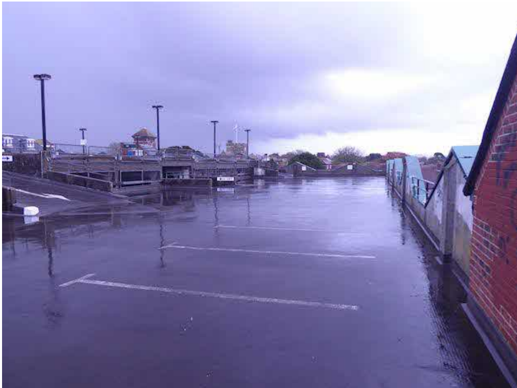
Photograph 47 – Further view of the lower section of the top deck, looking north.
