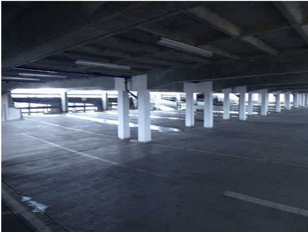
Photograph 39 – Further view of structure on the floors adjacent to the top deck.
