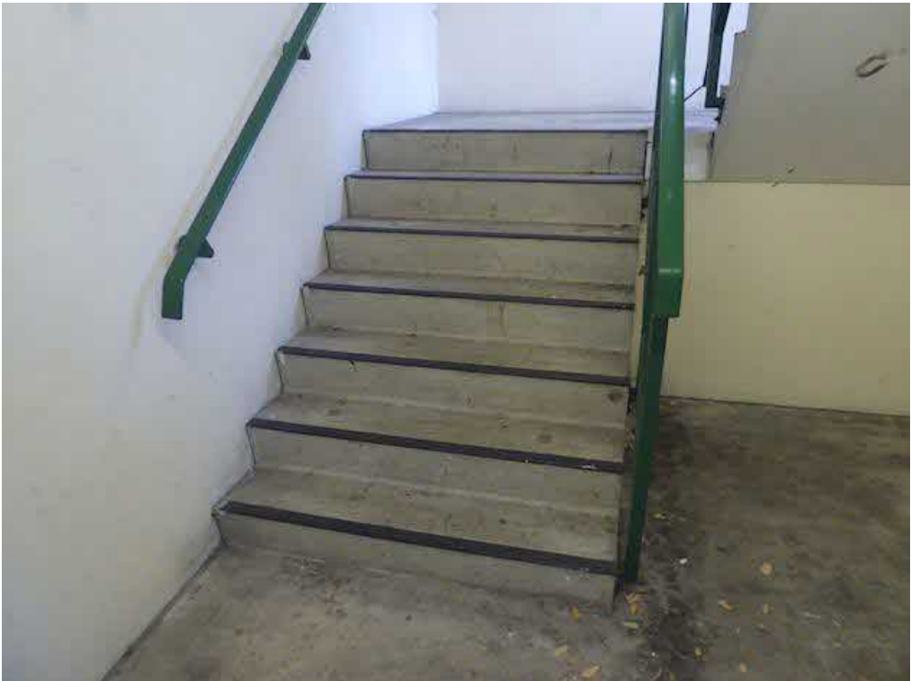
Photograph 45 – View of staircases within the southwest core.
