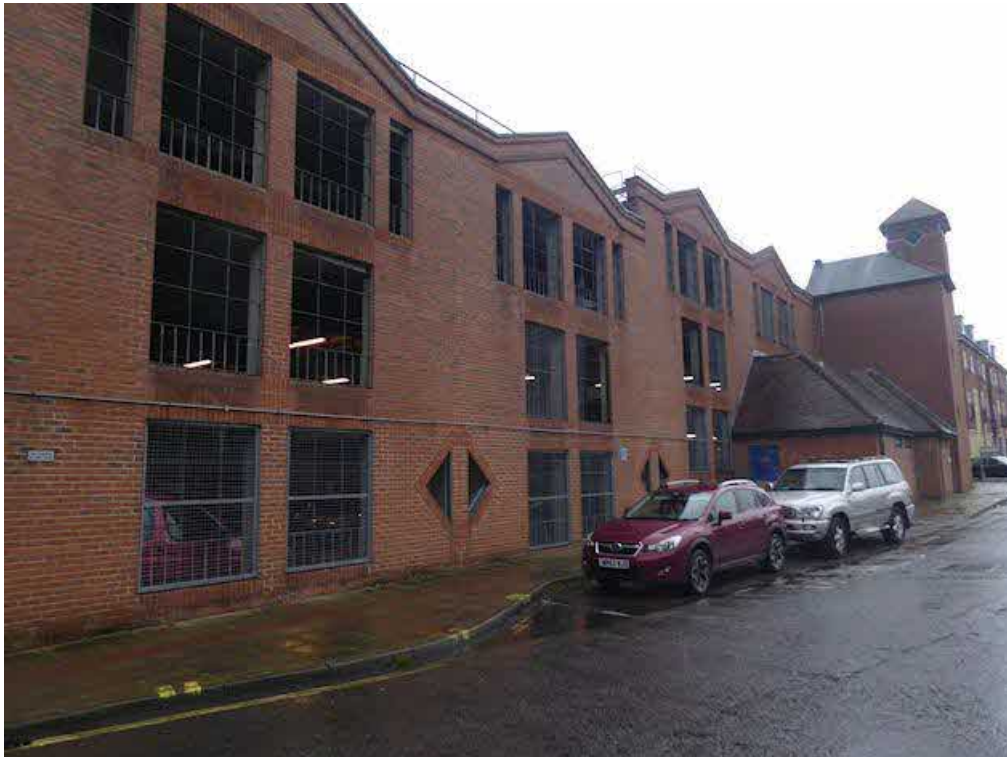
Photograph 13 – General view of the east elevation.
