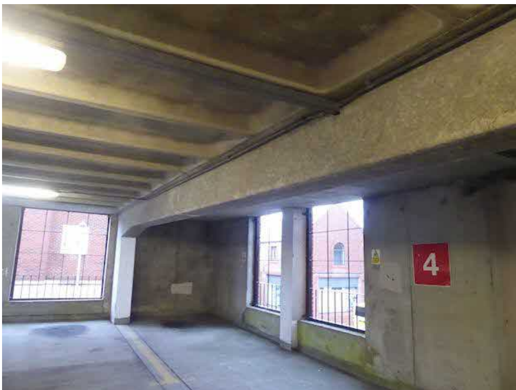
Photograph 37 – View of the structure adjacent to the external wall on the upper floors.
