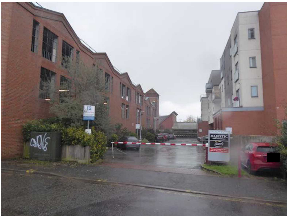
Photograph 24 – Further view of the car park sitting towards the west of the building.
