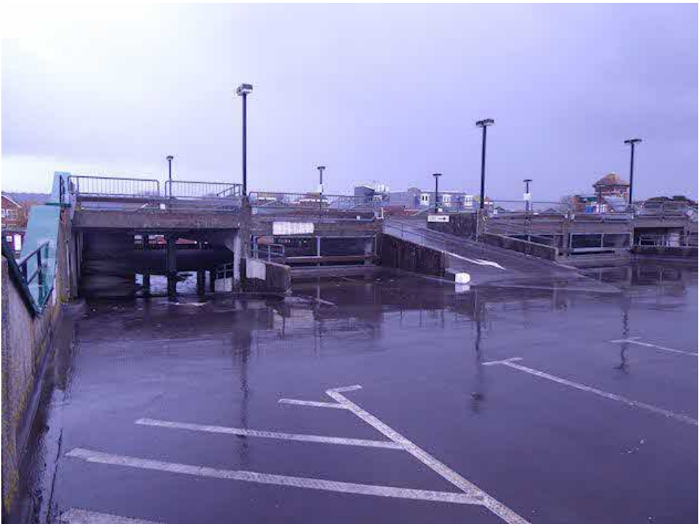
Photograph 46 – General view of the lower section of the top deck.
