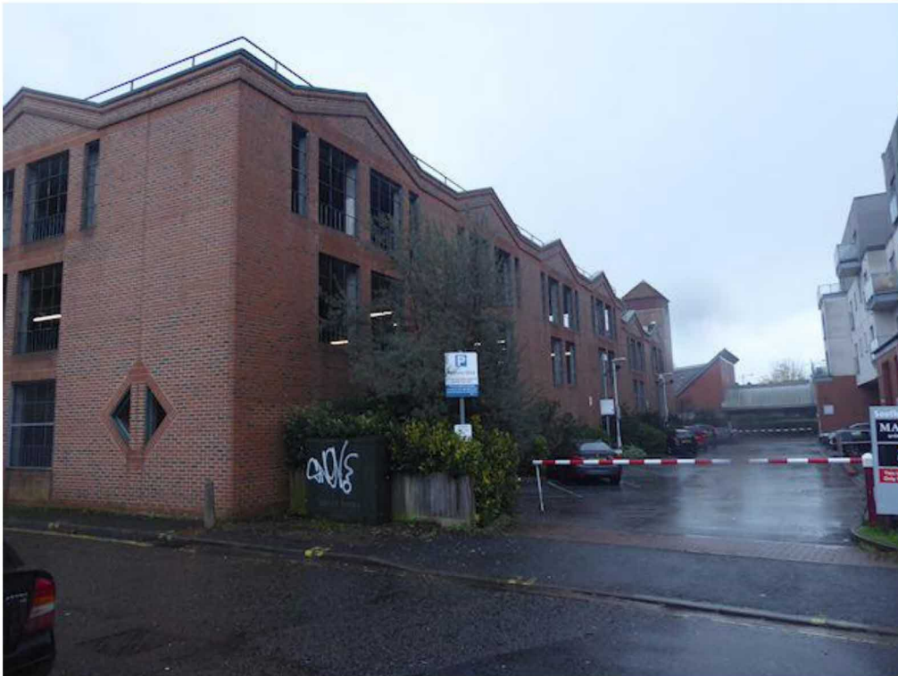
Photograph 23 – General view of the west elevation overlooking the adjacent car park.
