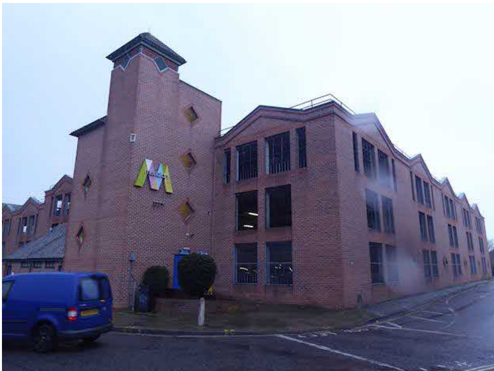
Photograph 18 – Further view of the northeast corner of the building.
