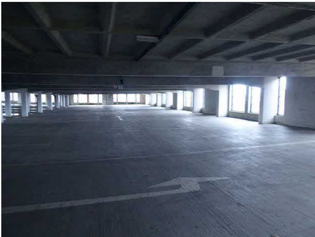
Photograph 40 – Further view of the structure adjacent to the top deck.
