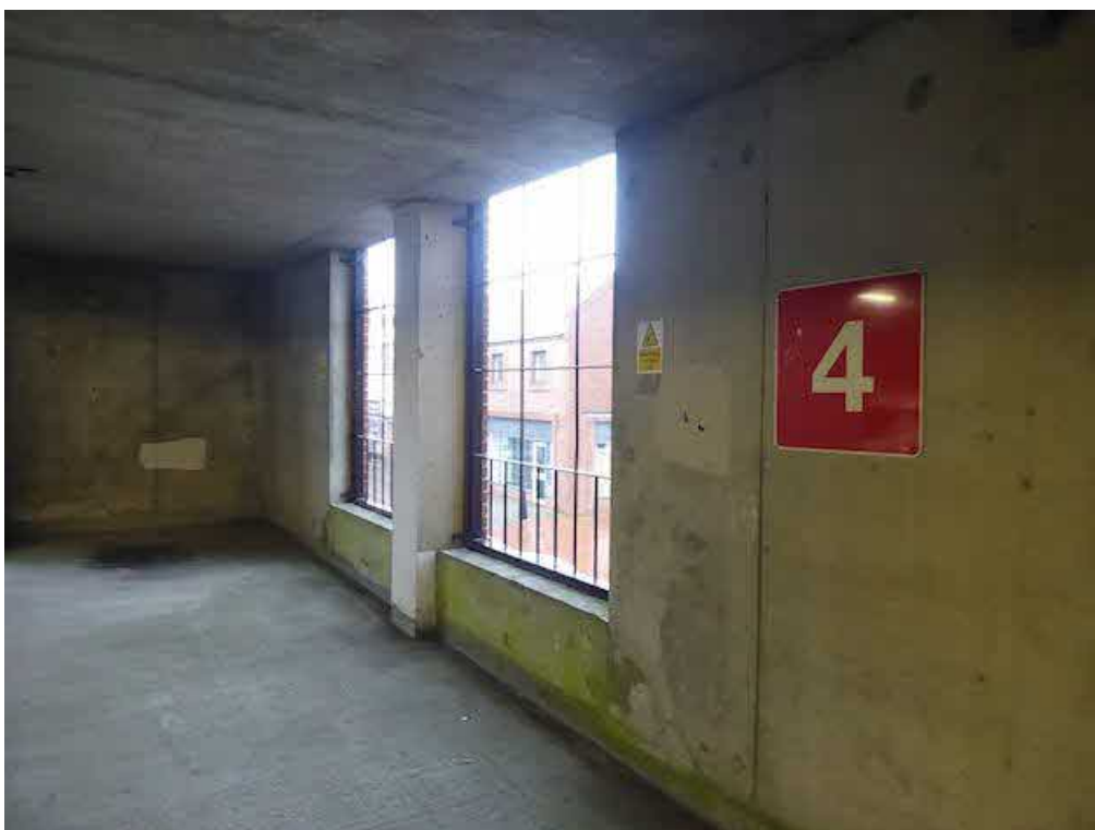
Photograph 38 – View of the external finishes to the upper floor.
