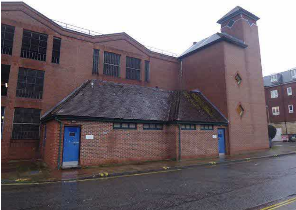
Photograph 15 – General view of the public toilets and the northeast stair tower.
