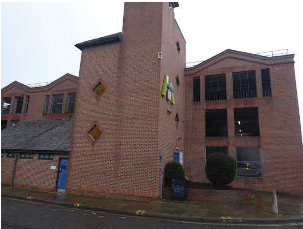
Photograph 17 – General view of the northeast corner of the building, including the stair tower.
