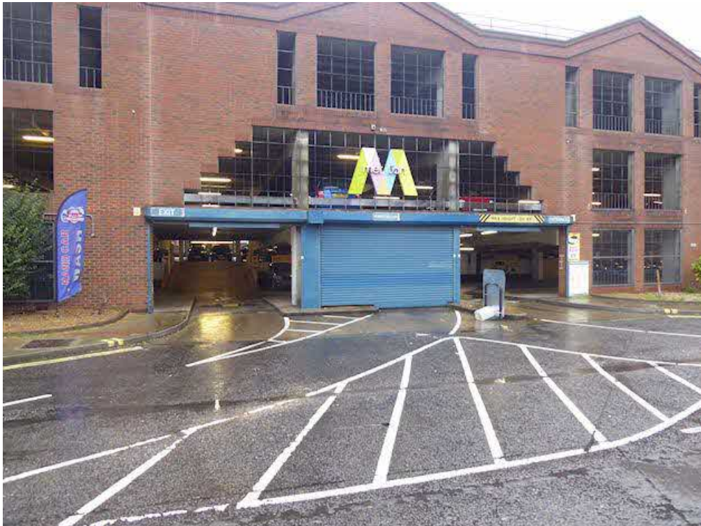
Photograph 7 – General view of the entrance into the car park along the south elevation.
