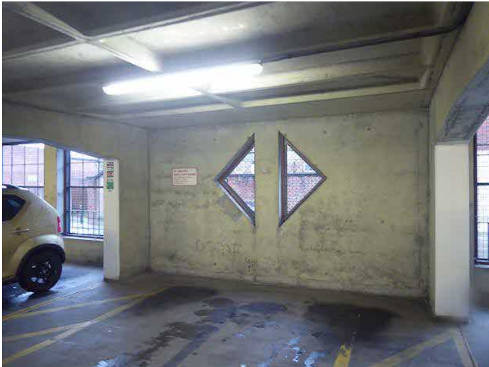
Photograph 33 – General view of the external wall finishes to the lower deck.
