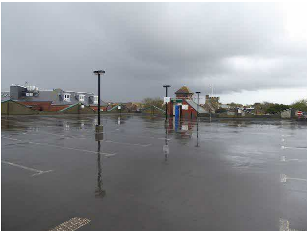
Photograph 52 – General view of the top deck, looking north.
