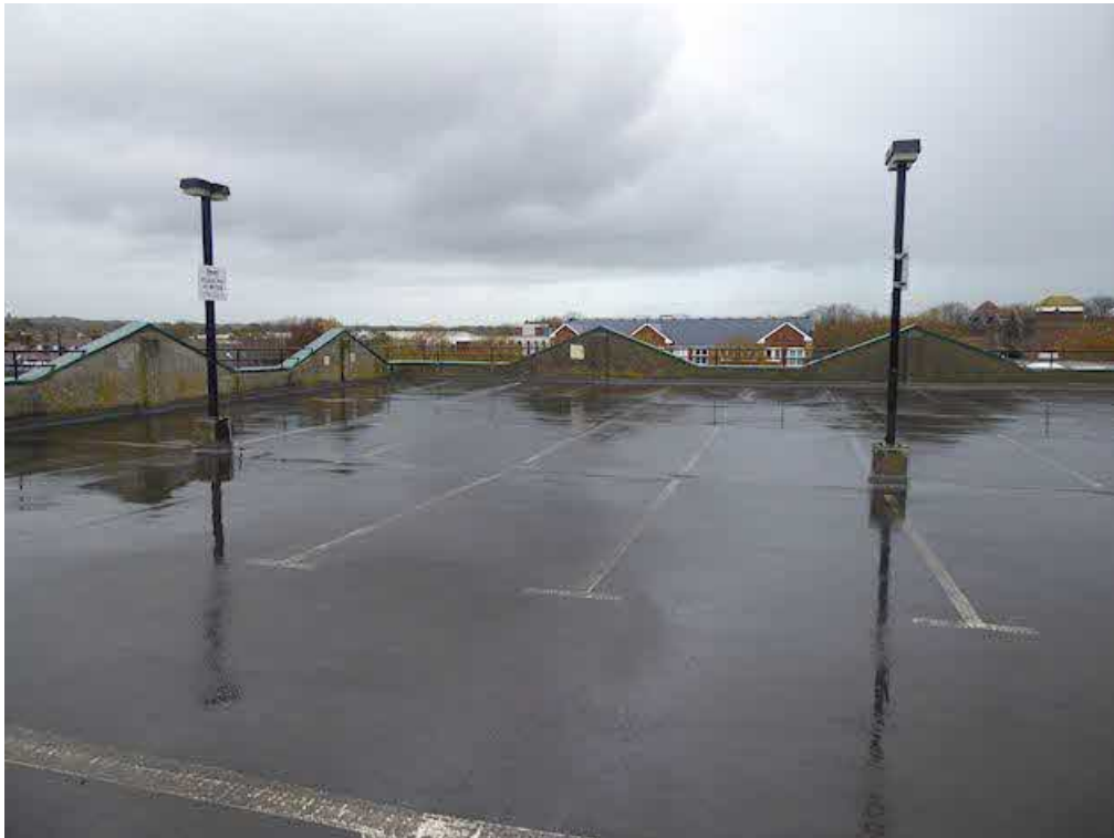
Photograph 51 – General view of the top deck, looking west.
