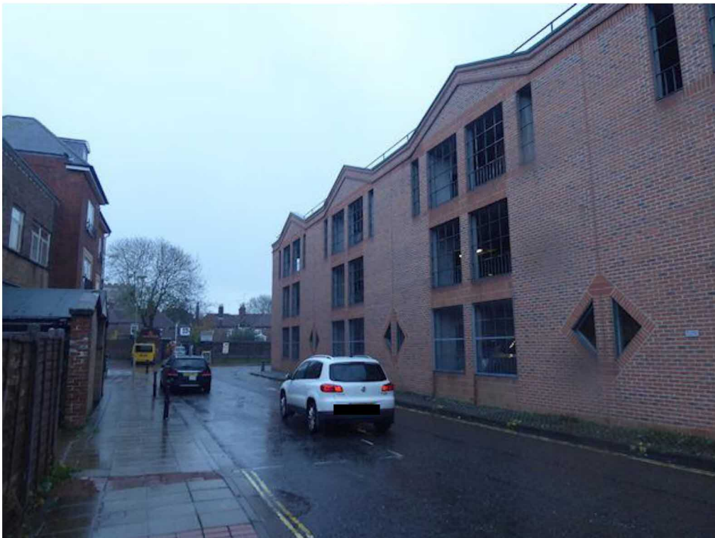
Photograph 22 – General view of the north elevation looking east.
