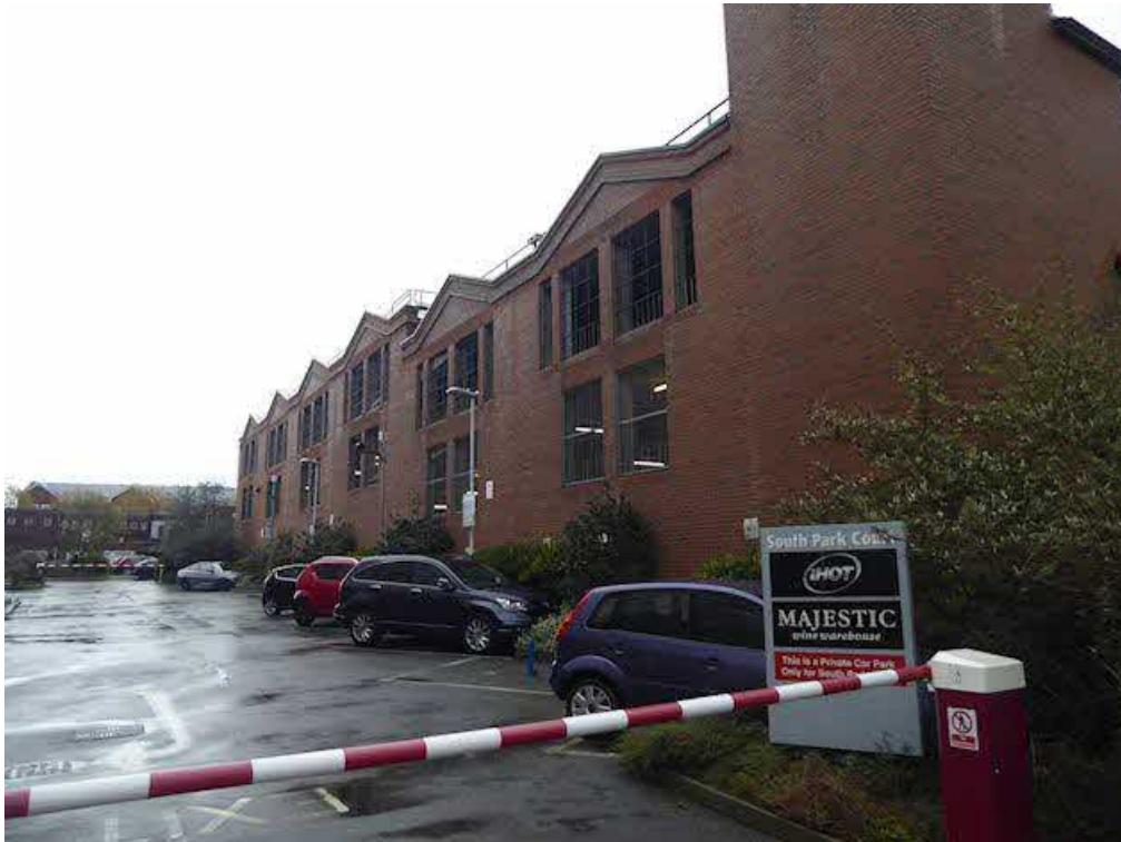
Photograph 1 – General view of the west elevation overlooking the adjacent car park.
