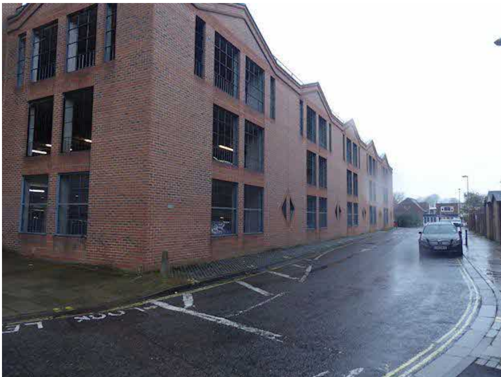
Photograph 20 – Further view of the north elevation.
