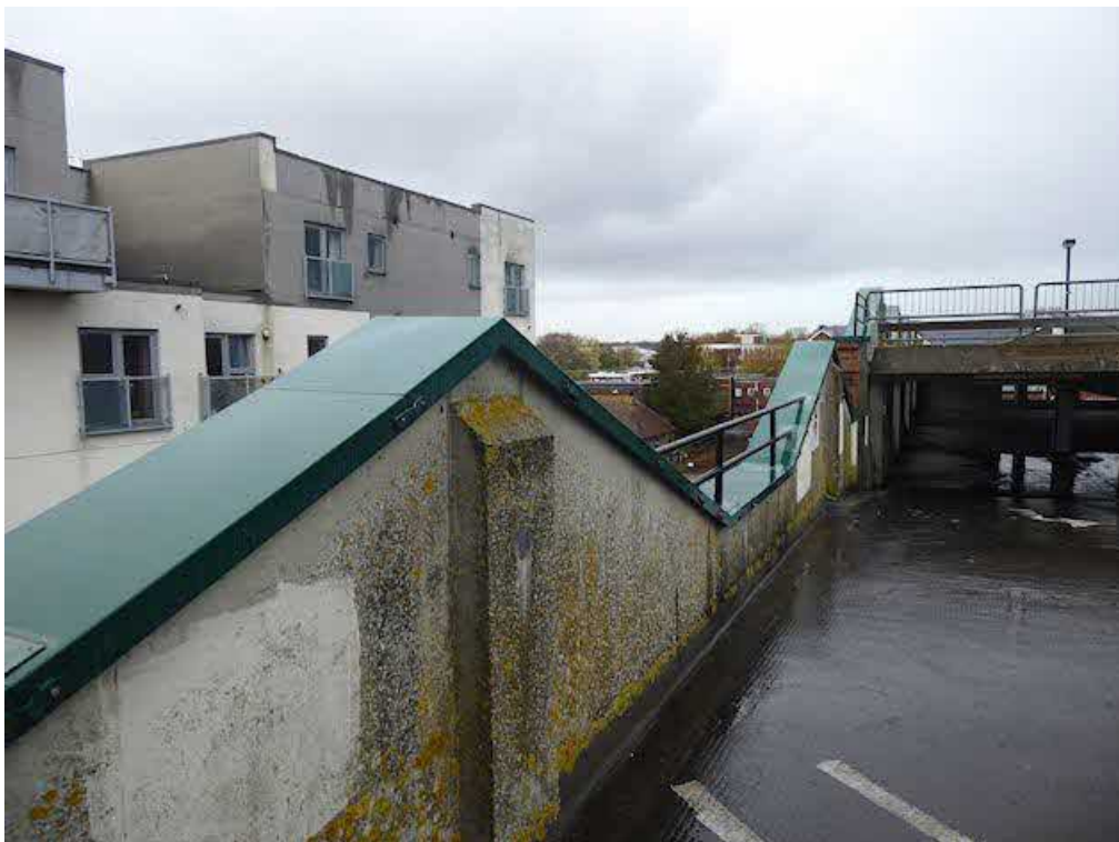
Photograph 48 – General view of the finishes around the perimeter of the lower top deck.
