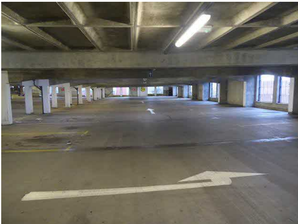
Photograph 36 – Further view of the structure of the building on upper floors.
