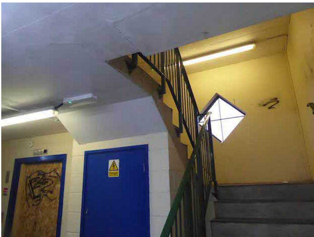
Photograph 29 – Further view of the northeast core.
