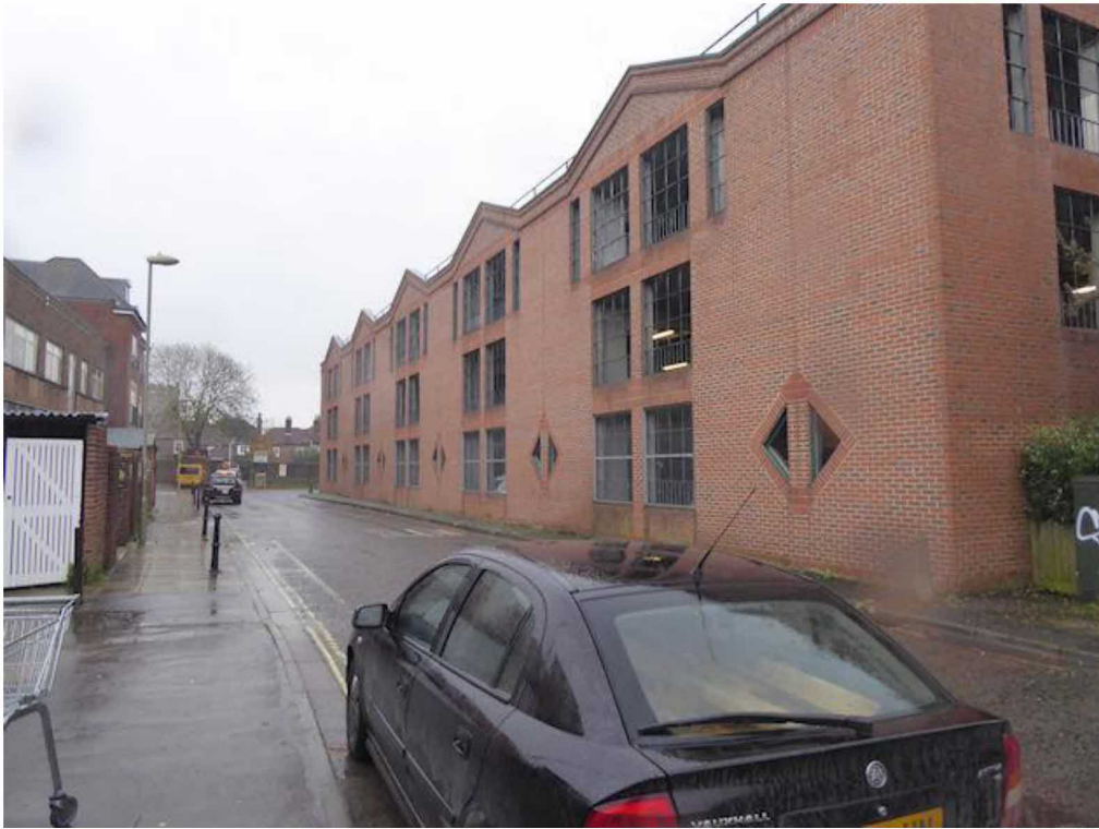
Photograph 25 – View looking east up Bulbeck Road, noting the north elevation.
