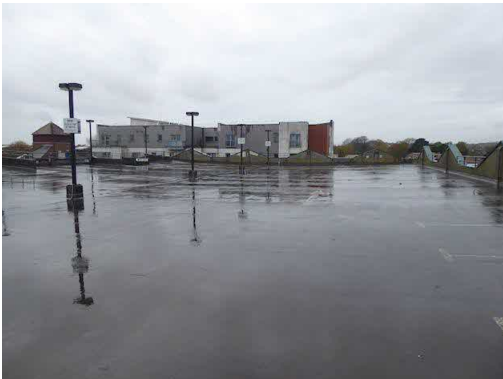
Photograph 54 – Further view looking west on the top deck.
