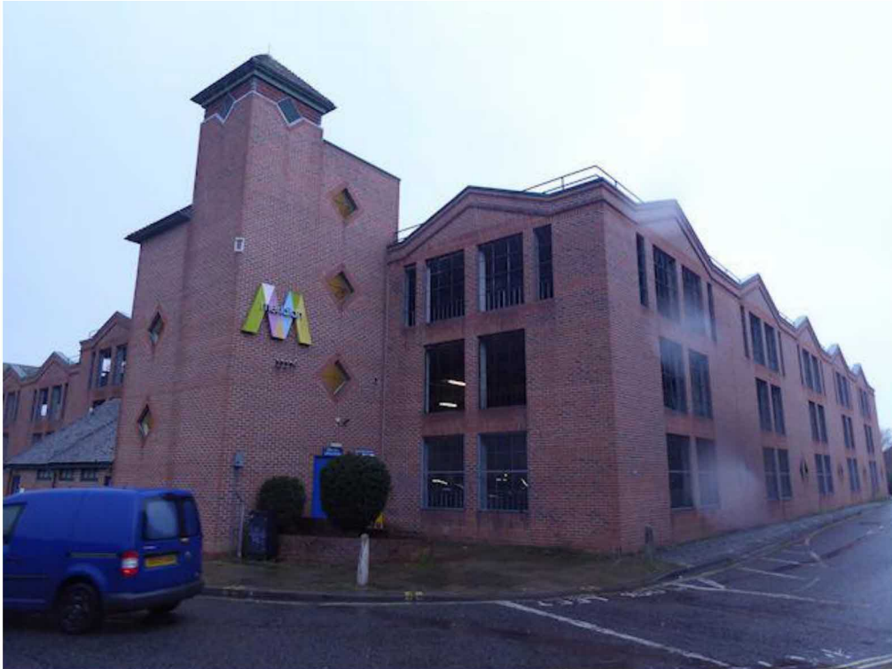
Bulbeck Road Car Park, Havant, Hampshire, PO9 1HN
