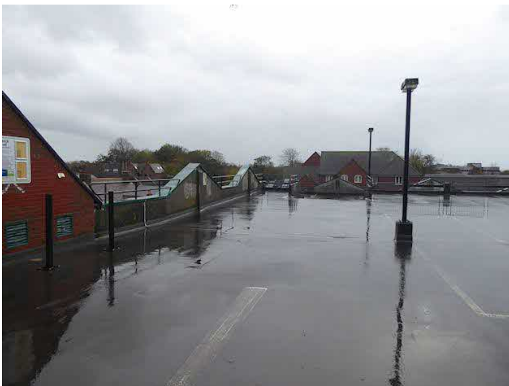
Photograph 56 – General view of finishes to the top deck, including around the perimeter.
