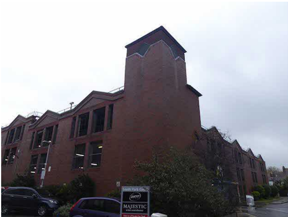
Photograph 2 – General view of the southwest corner and stair tower.
