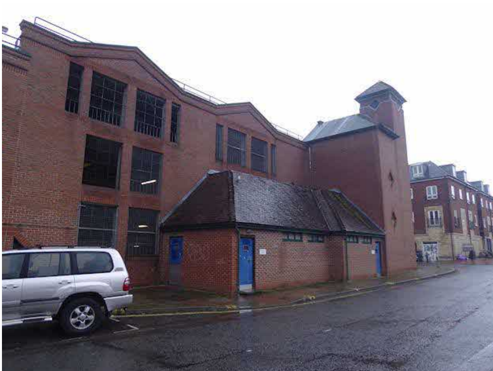
Photograph 14 – Further view of the east elevation, noting the public toilets and northeast stair tower.
