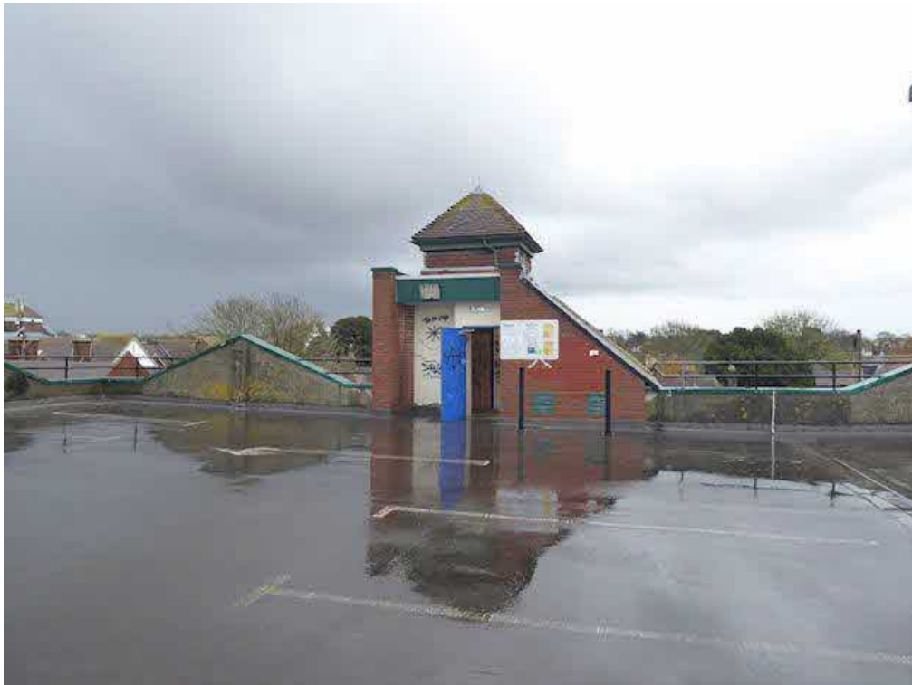
Photograph 53 – General view of the northeast stair tower on the top deck.
