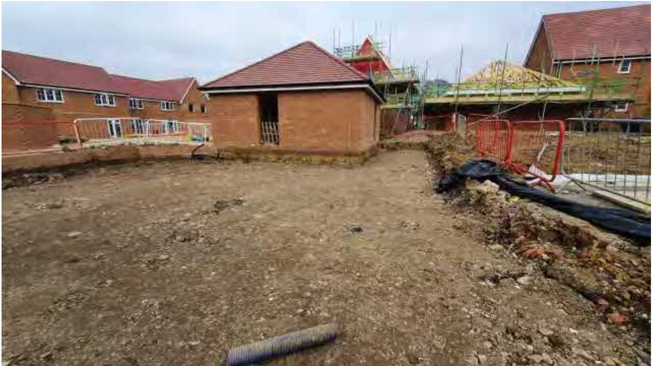
Plate 1 – View of crushed concrete installed across Plots 117-118
