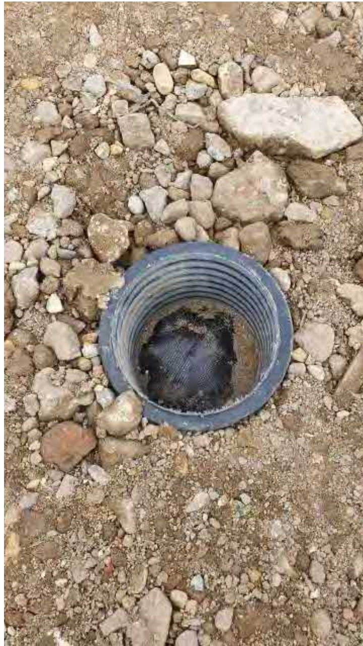
Plate 2 – View of geotextile membrane installed beneath the crushed concrete in Plot 117
