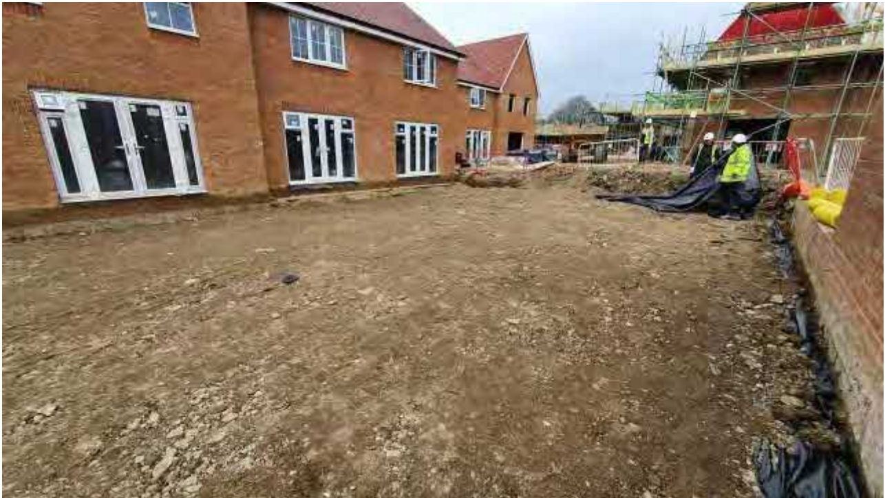
Plate 3 – Crushed concrete installed across Plots 136-138
