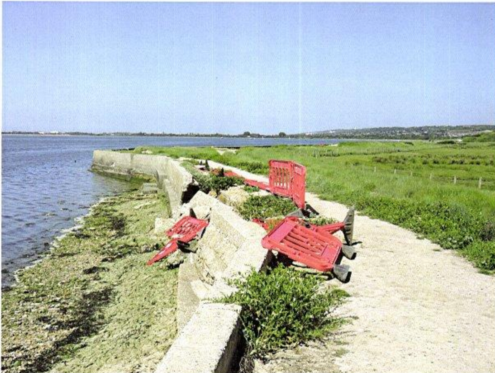
Image 1. Deteriorating seawall at proposed breach location
