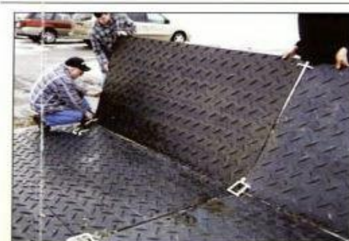
DOUBLE LINK JOINERS - lock Ground-Guards into one large working platform.
