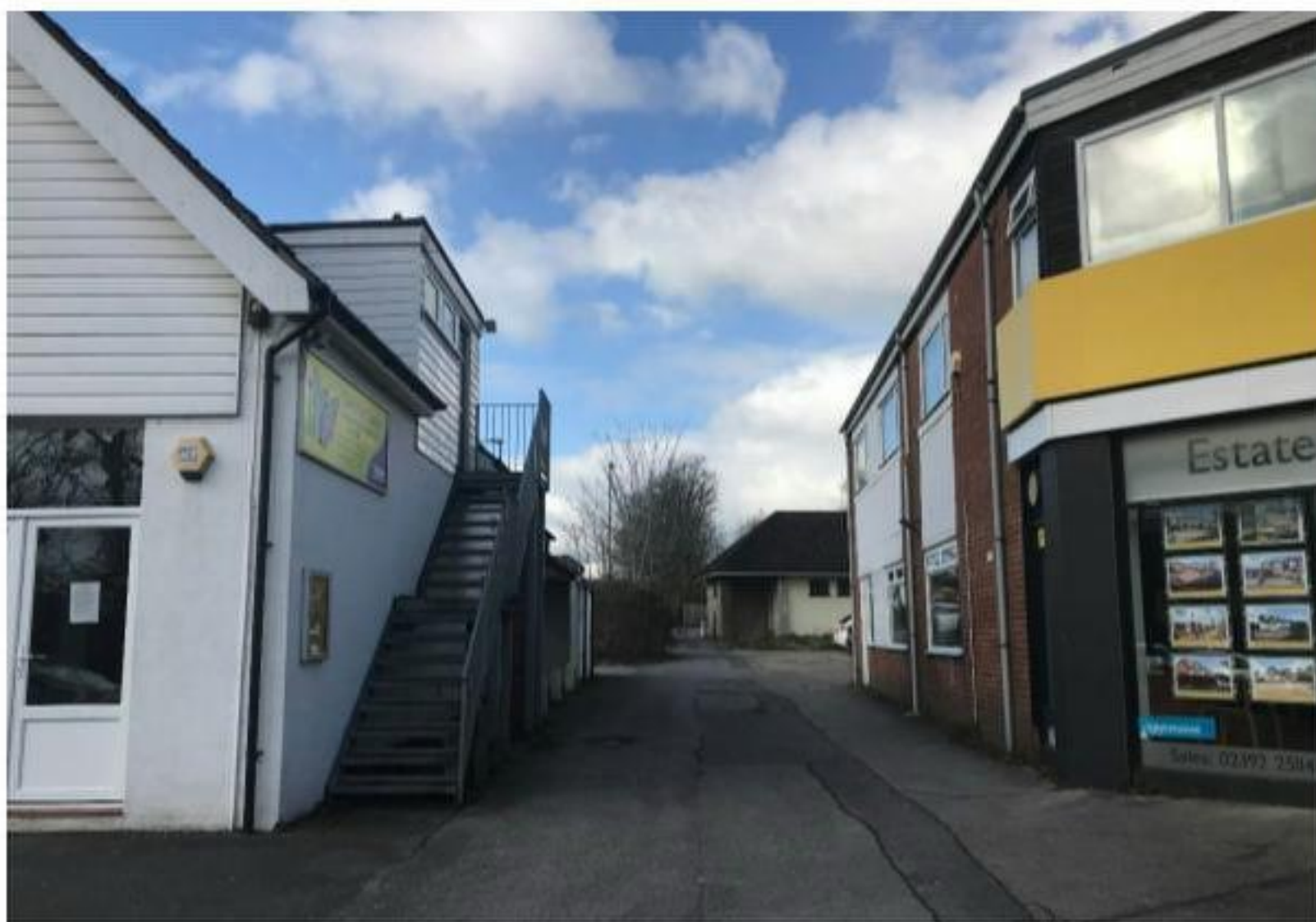
Existing access to the site from London Road
