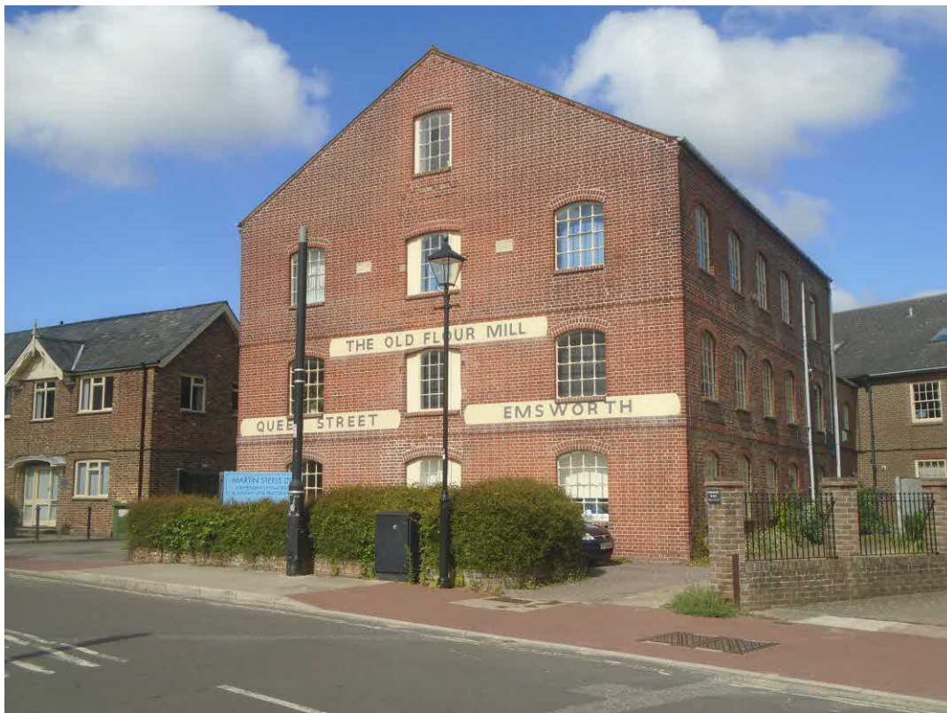
Figure 6. The Old Flour Mill (listed building) opposite application site in Queen Street.
