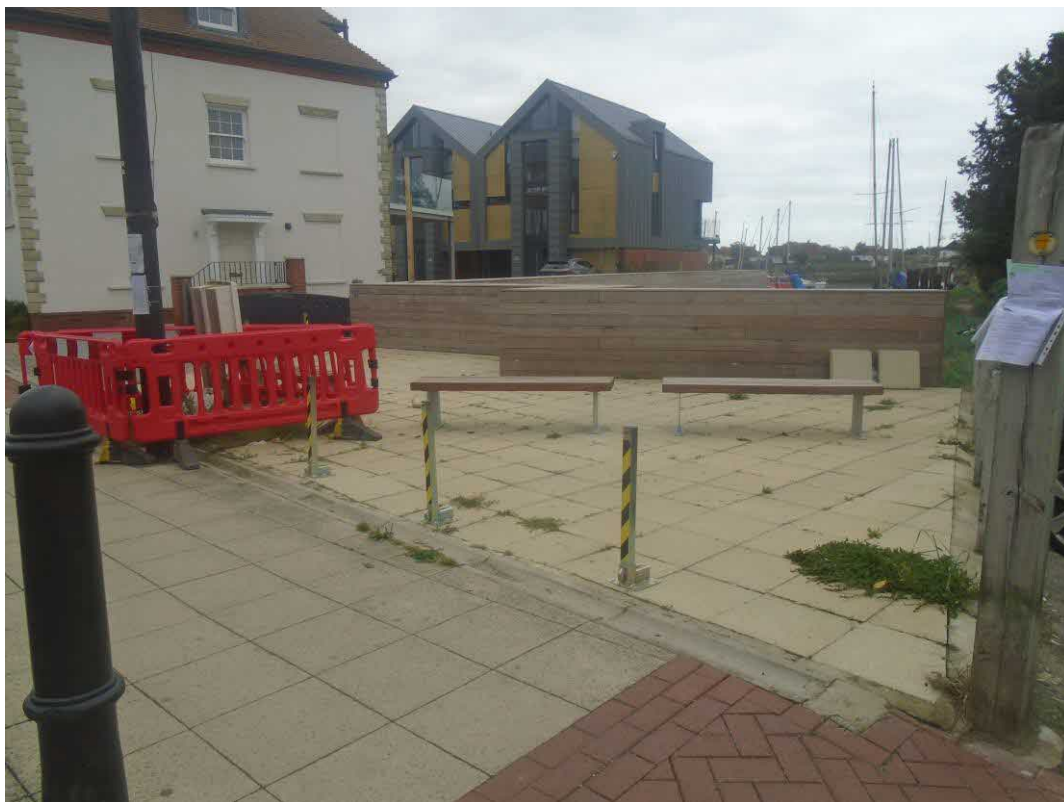
Figure 1. The application site
