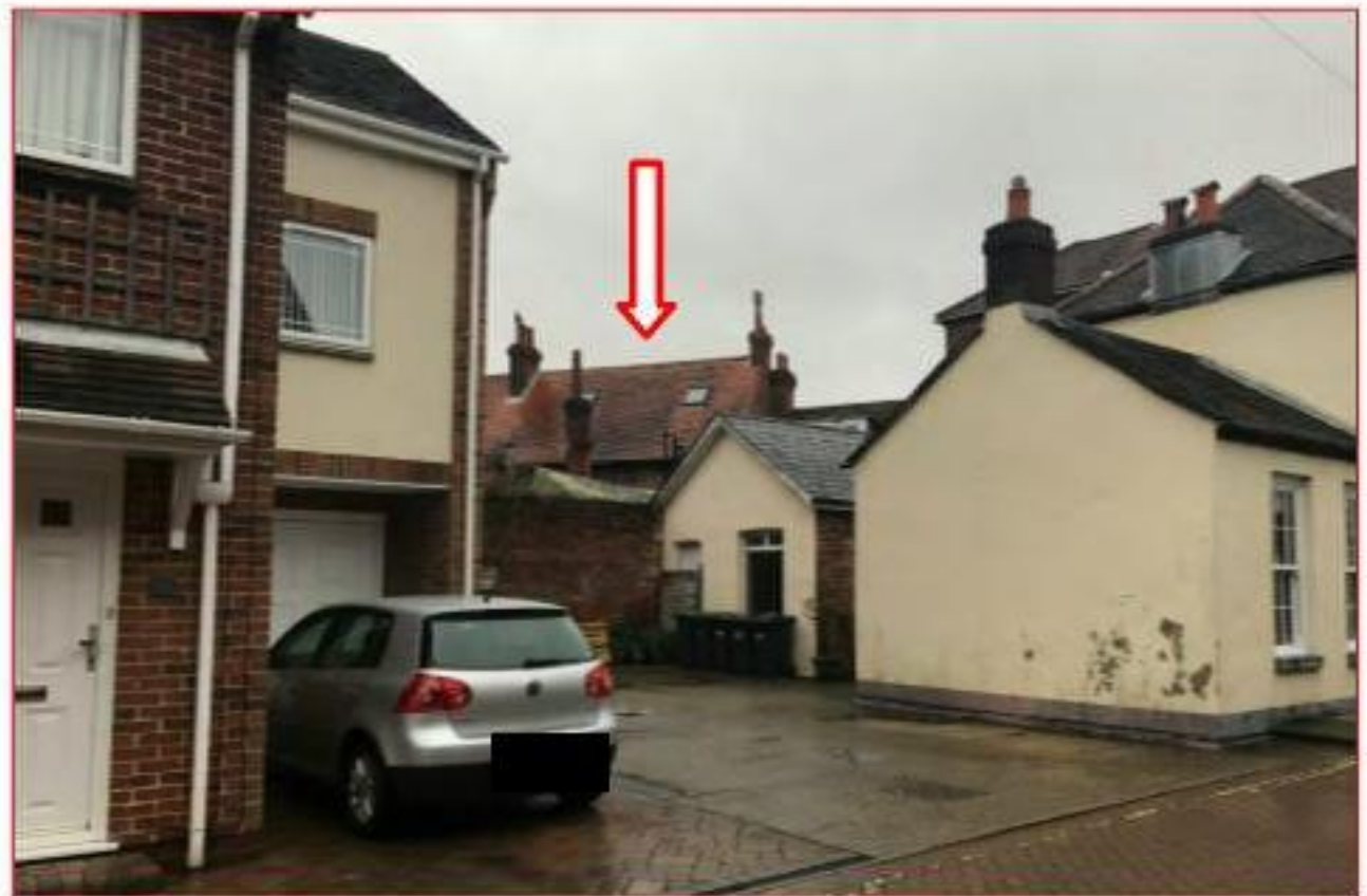
Plate 14 View of part of rear roof slope to subject building (arrowed) taken from School Lane. Note that the two-storey addition will be partially visible in this view.
