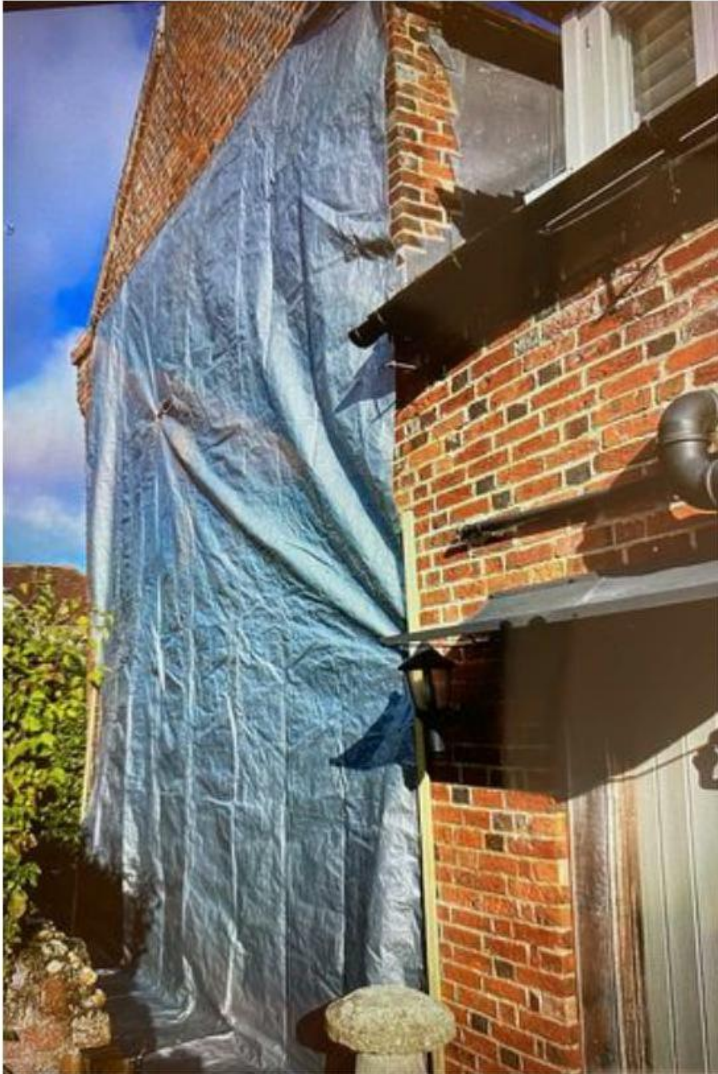
Image 7 – an emergency effort made to prevent further moisture penetration
