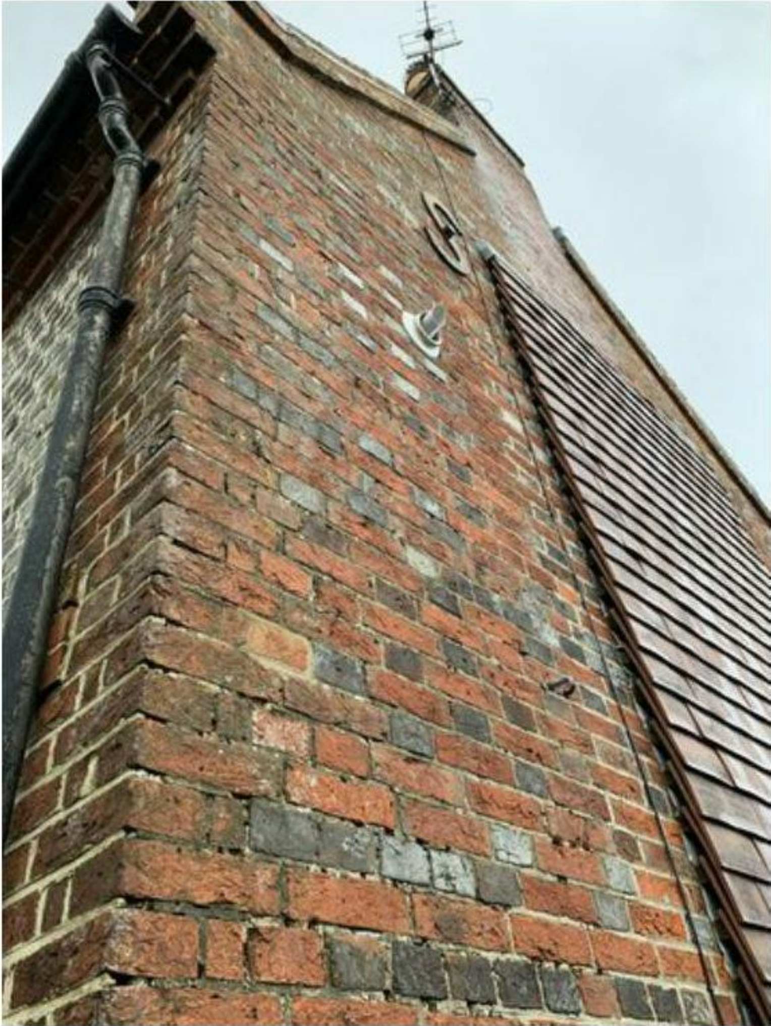
Image 6 – existing gable wall, showing the modern tile-hanging and some repointing
