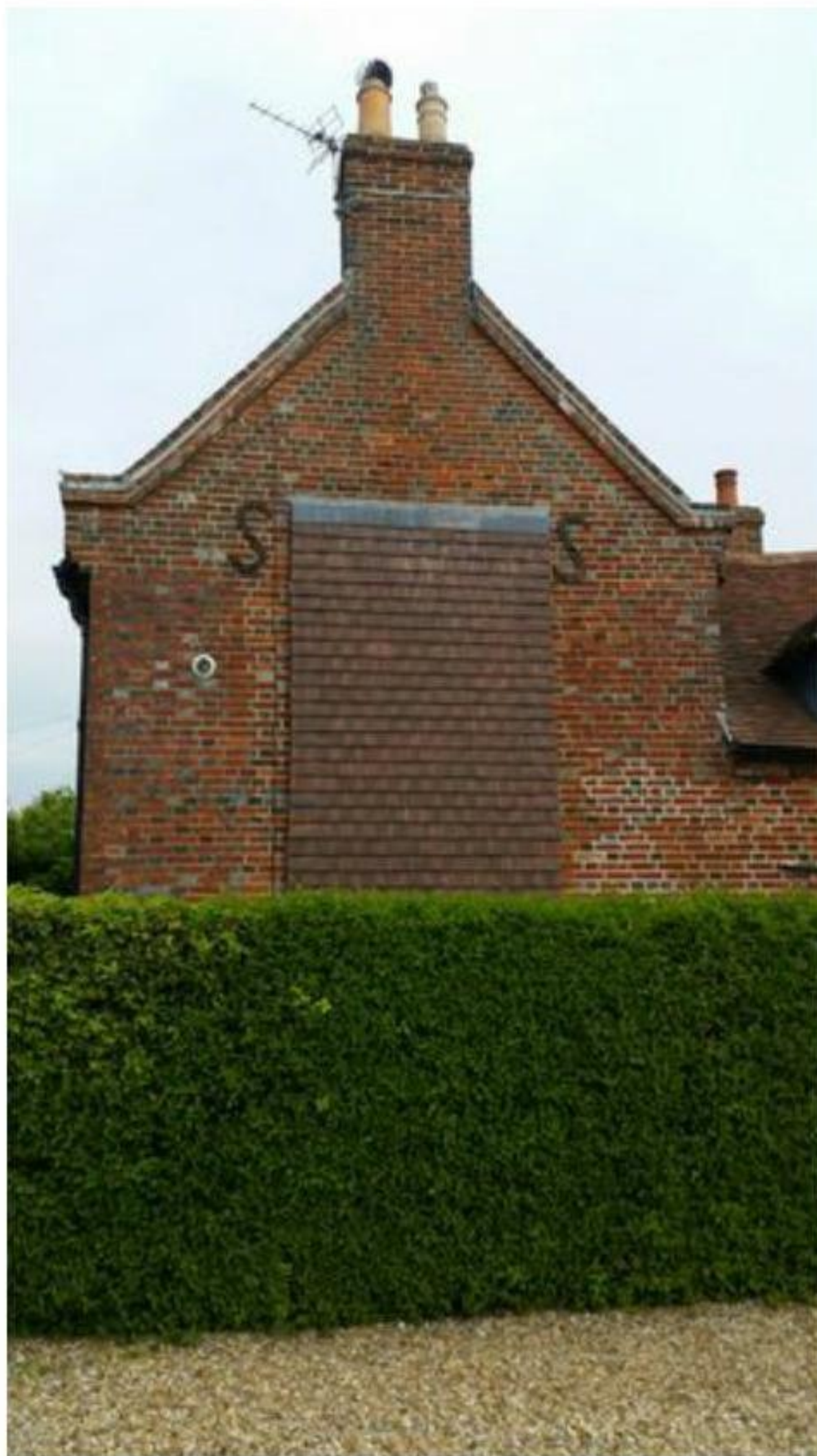
Image 10 – existing gable wall
