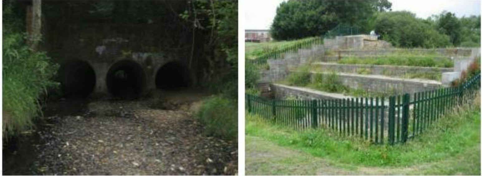
Photo 4: Major culvert & weir on Park Lane Stream
