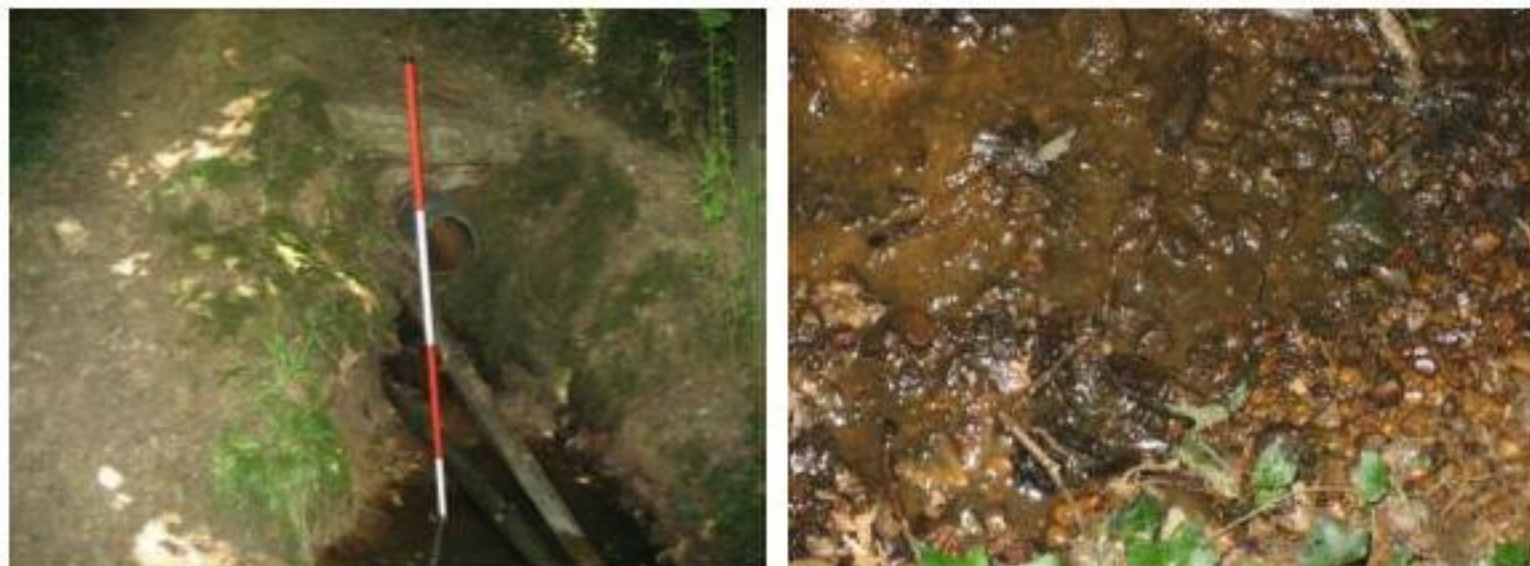
Photo 6: Outfall pipe from Upper Lake & gravel / pebble substrate
