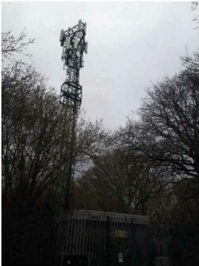
Plate 14: Vodafone telecommunications mast and associated electrical substation.
