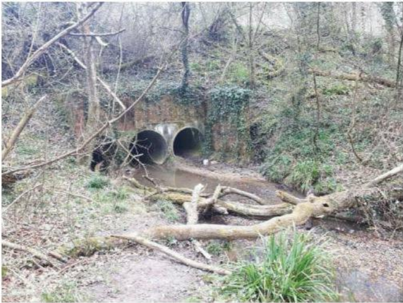
Plate 28: Looking at culvert for Park Lane Stream located south of the site.
