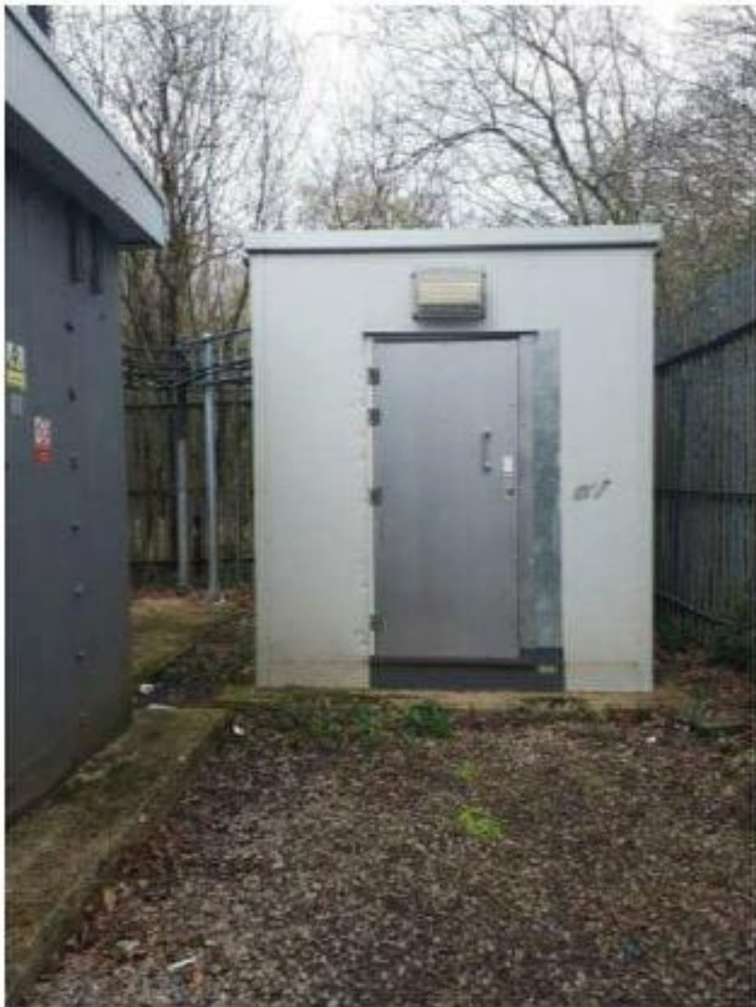
Plate 16: Building units associated with telecommunications mast.
