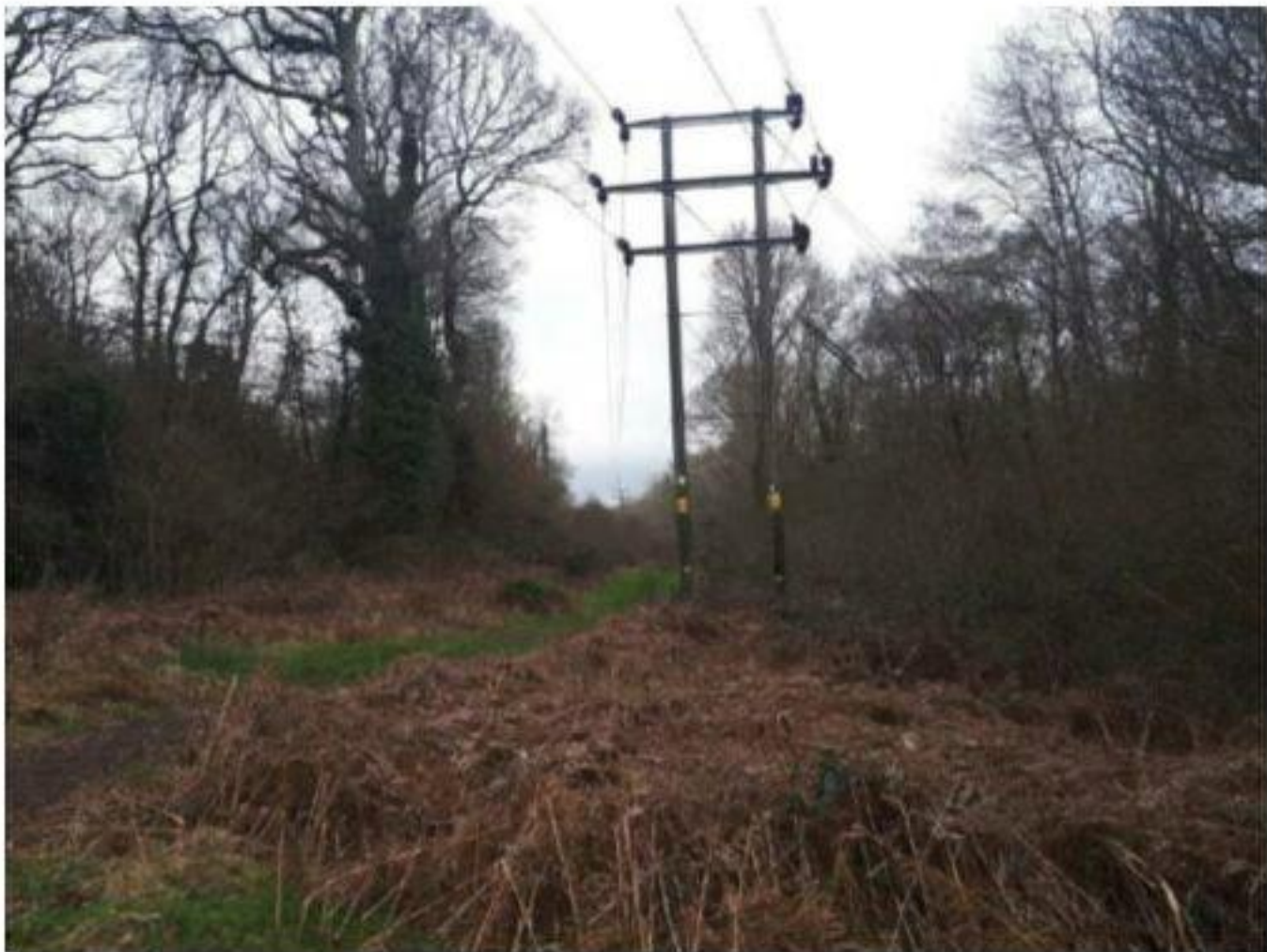
Plate 22: Looking at electric pylon located west of the site.
