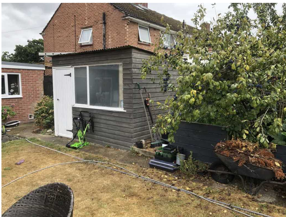
The existing shed by the west boundary is proposed to be demolished.
