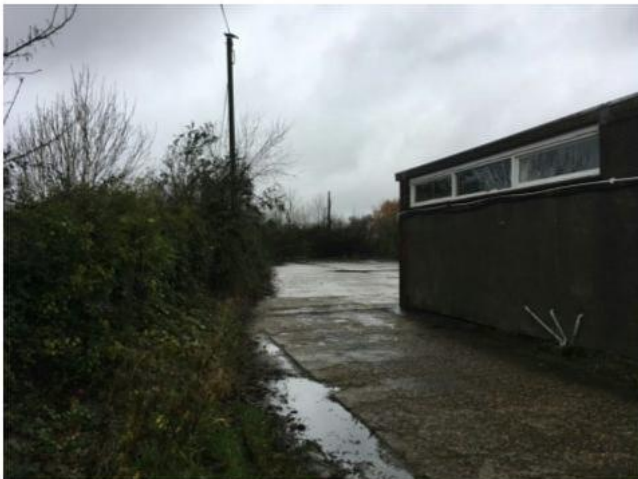
Side of existing structure looking towards concrete hard standing-formerly railway goods yard
