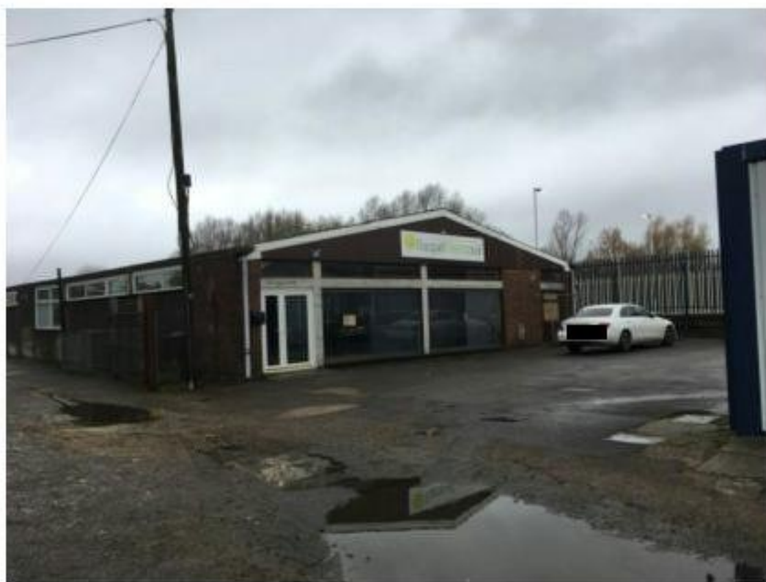
Front elevation of existing building showing main entrance
