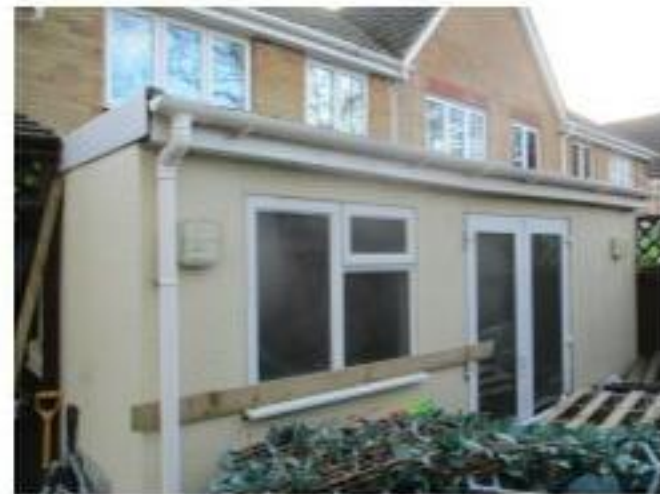
Fig 2. View of the existing single storey rear structure
