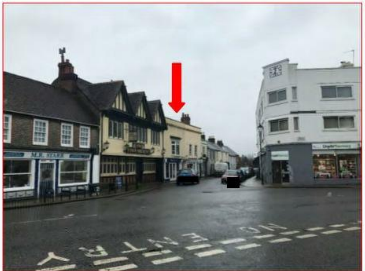
Plate 11 View looking west along West Street. Note nos. 6, 8 & 10 West Street (arrowed), which are identified as buildings of local interest that make a positive contribution to the Conservation Area.
