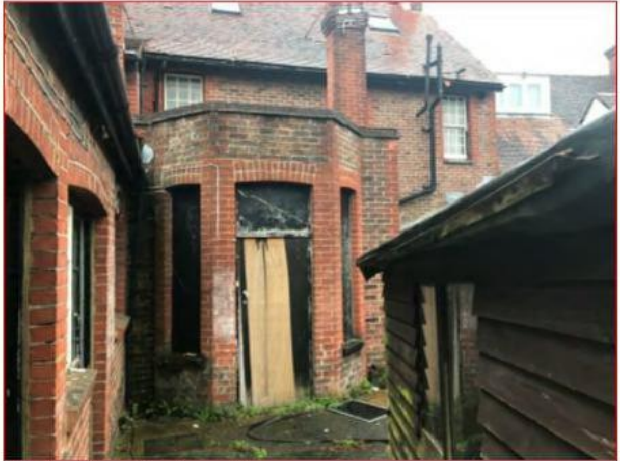
Plate 5 View of 'bay' rear addition.
