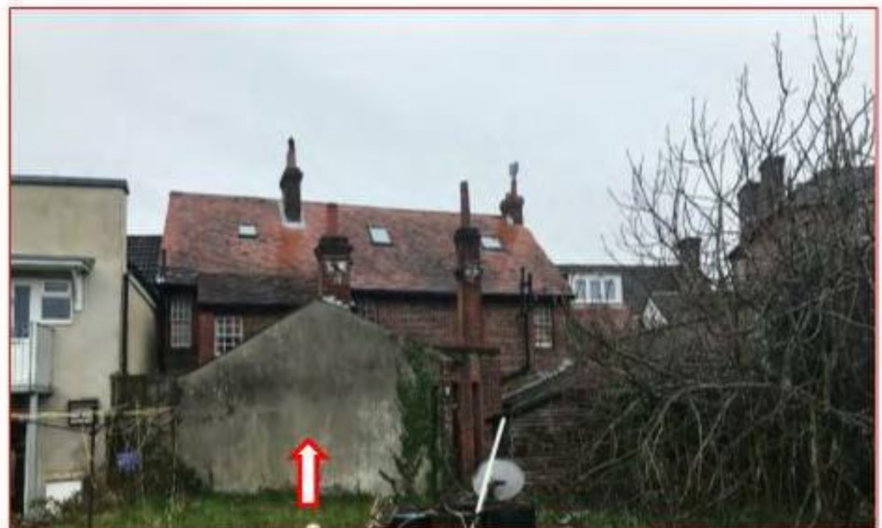
Plate 2 View of rear elevation (south facing) to subject building. Note the rendered face to the larger of the two existing rear historic wings (arrowed).
