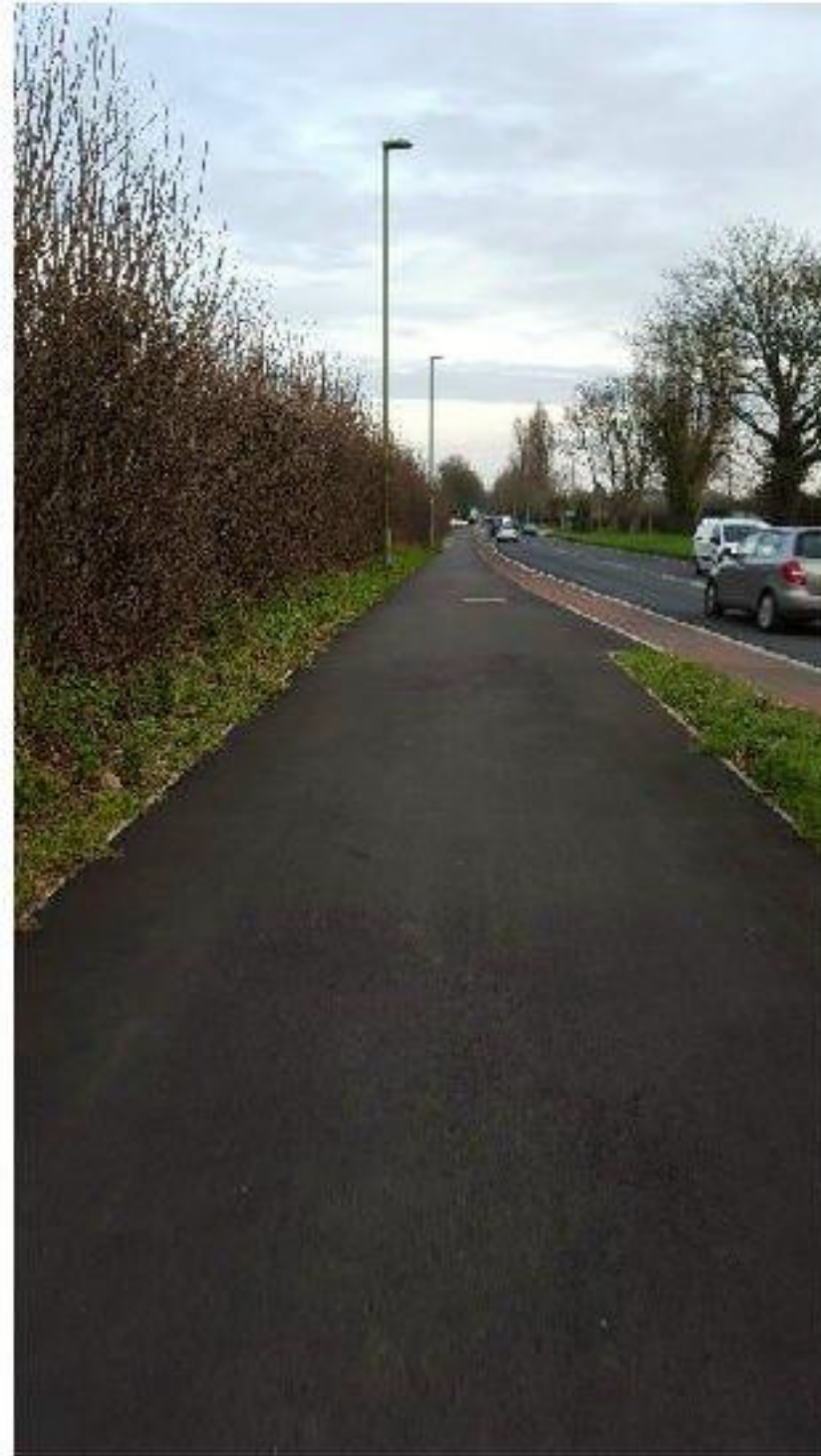
Photograph 3: Recently Improved Footway/ Cycle provision on Havant Road
