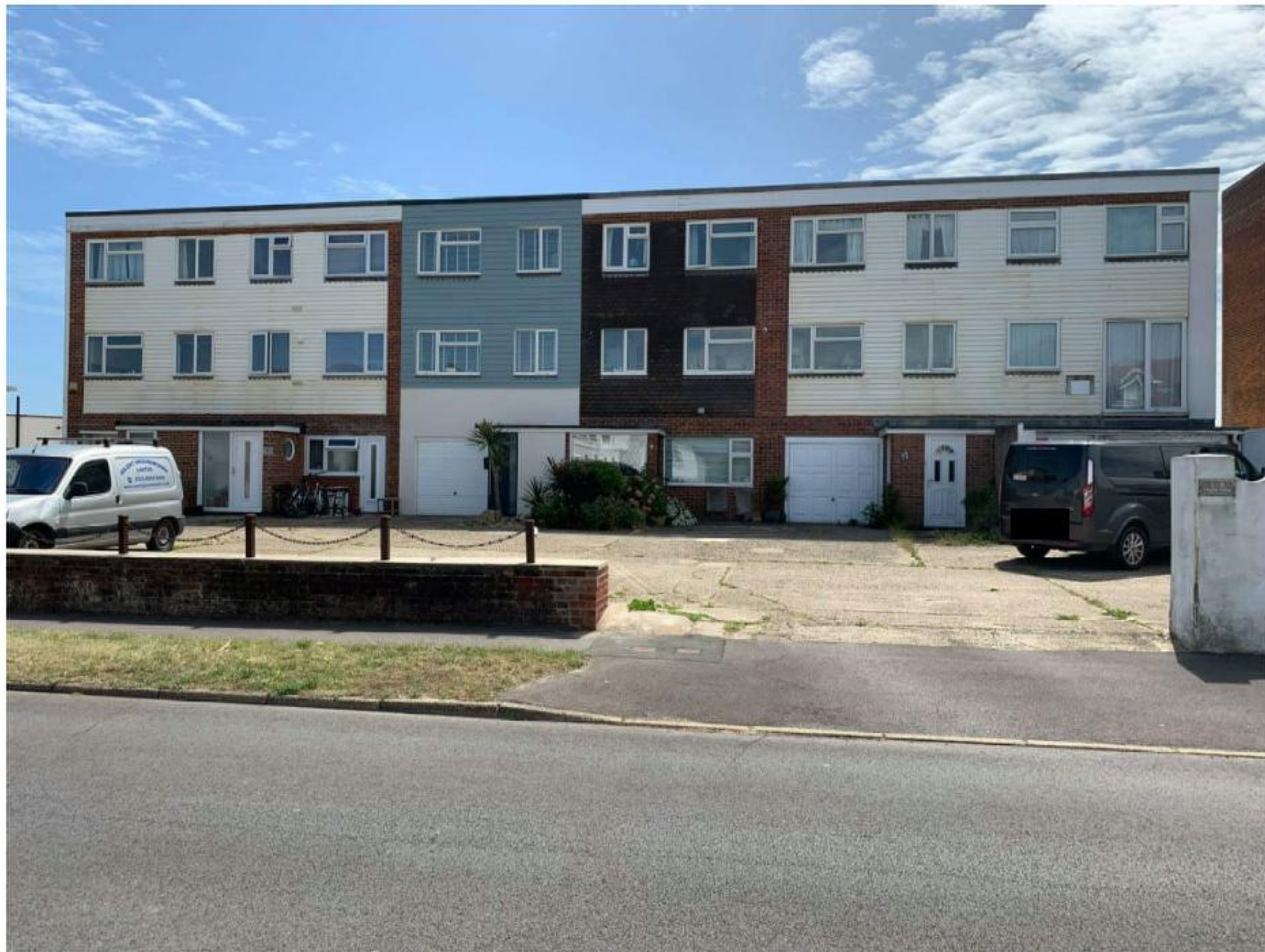
Town Houses Opposite.jpg
