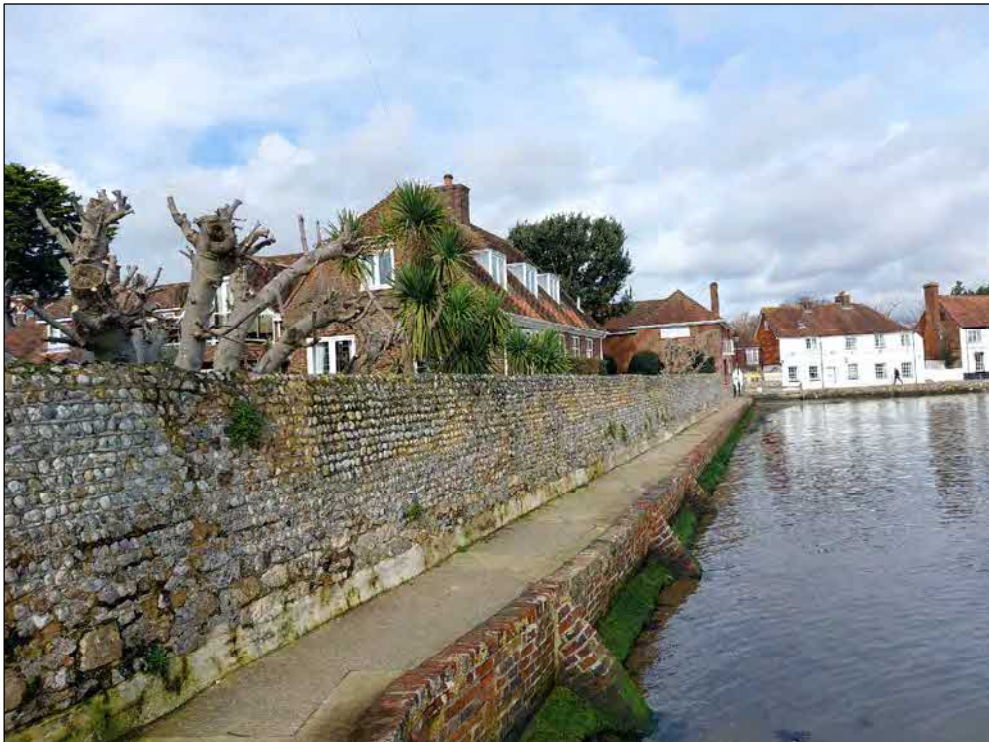
Photo 9) View looking north-east along the northern portion of the Frontage 4 harbour front
