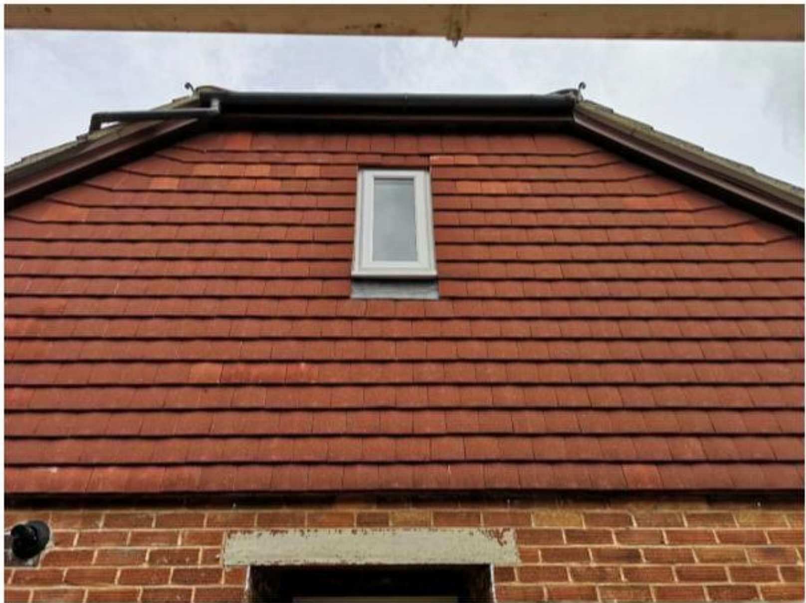
Photo 4: Side wall of No.17 Yew Tree Avenue
