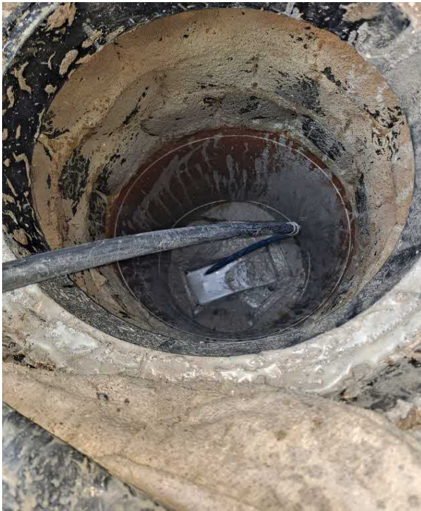
MH1 jetting in progress
