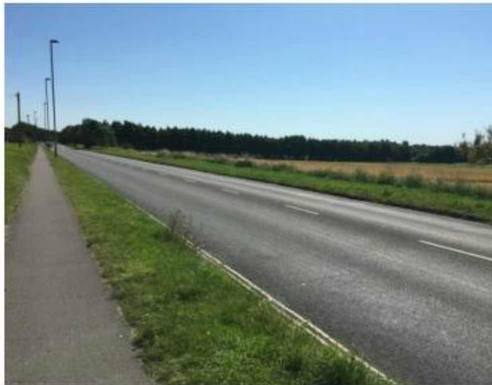
Photograph 16: Havant Road (A2030) Environment
