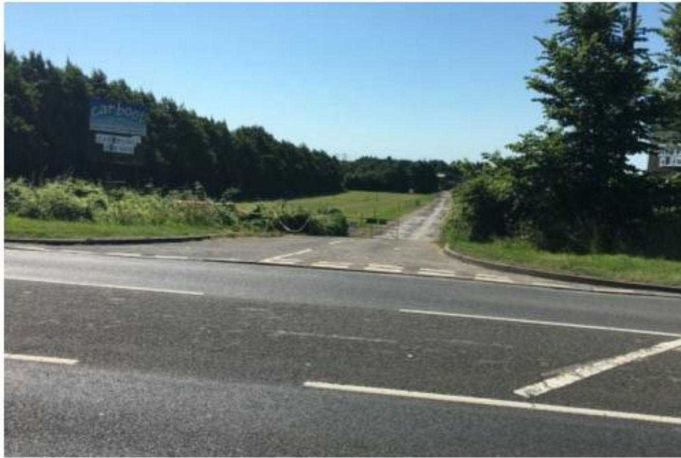
Photograph 1: Existing Site Access
