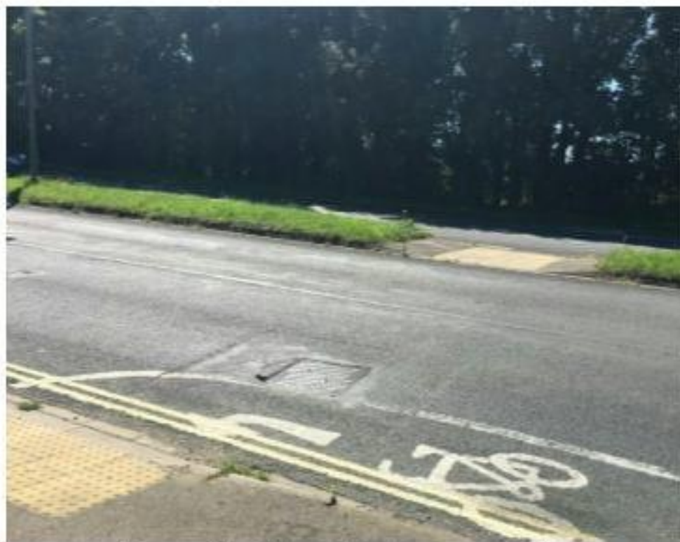
Photograph 9: Existing Pedestrian Crossing facilities
