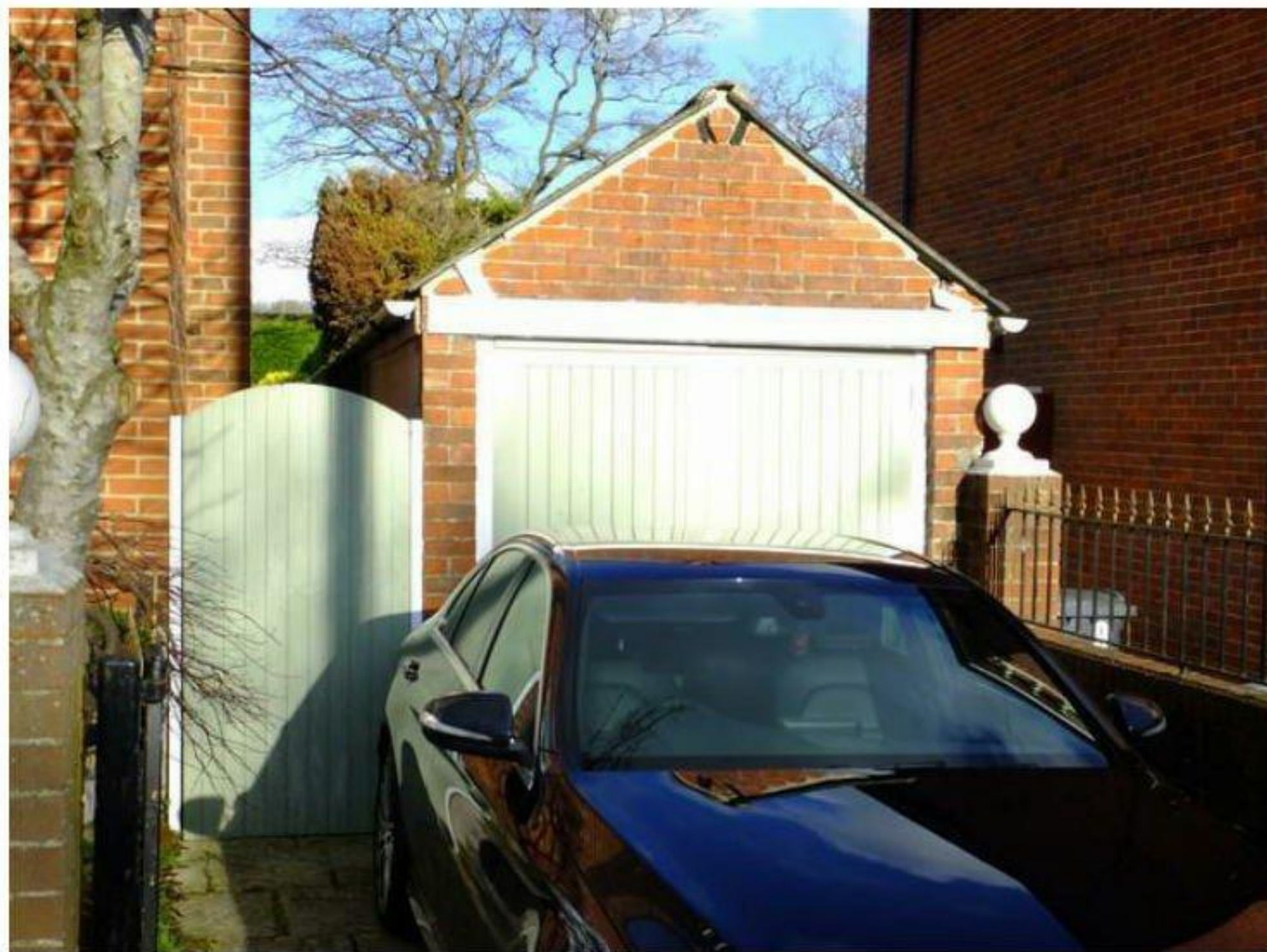
Image 8 Existing garage building that may be demolished for site access, then rebuilt
