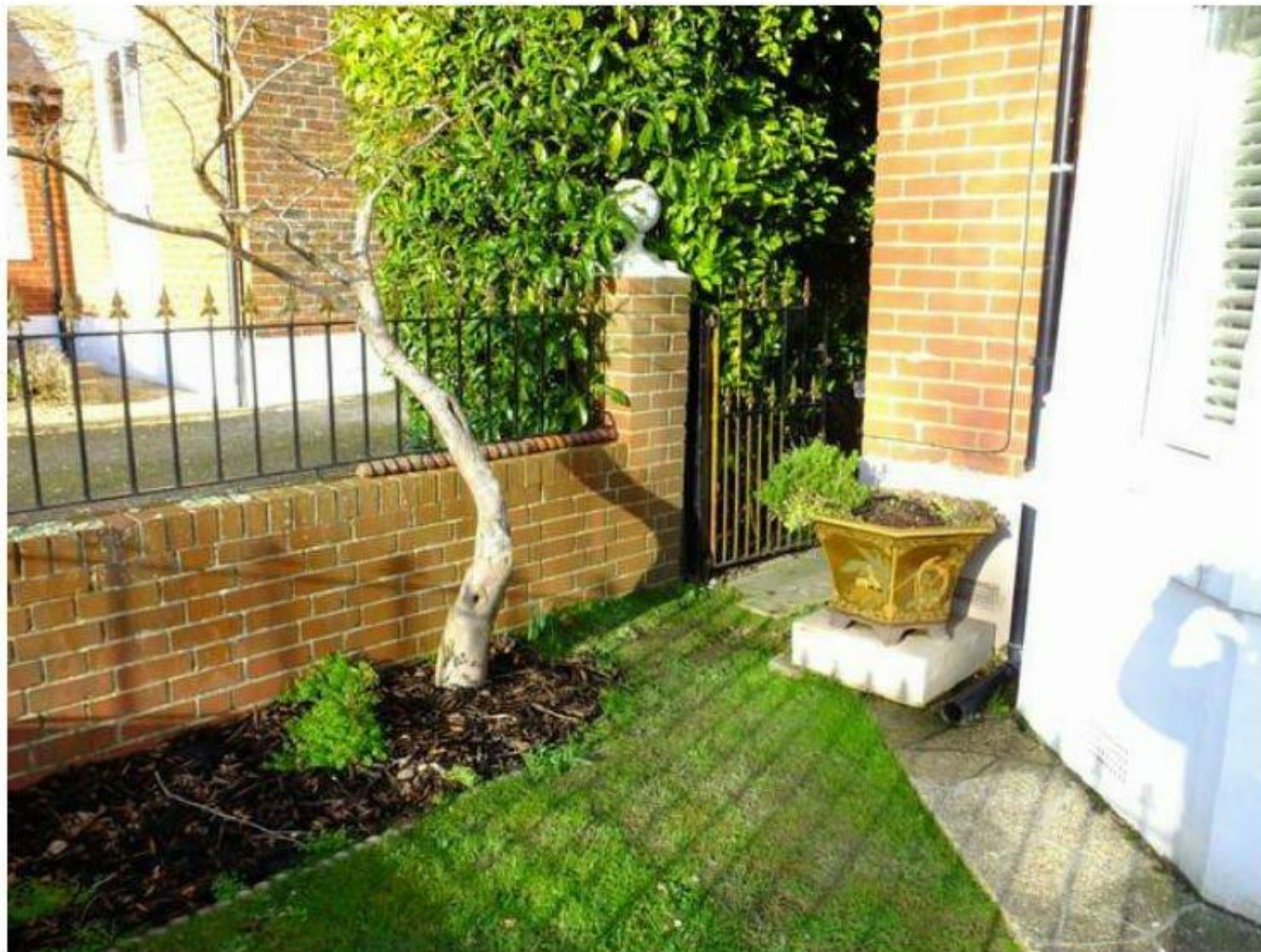
Image 7 T11 with existing stem damage that is to be removed for site access
