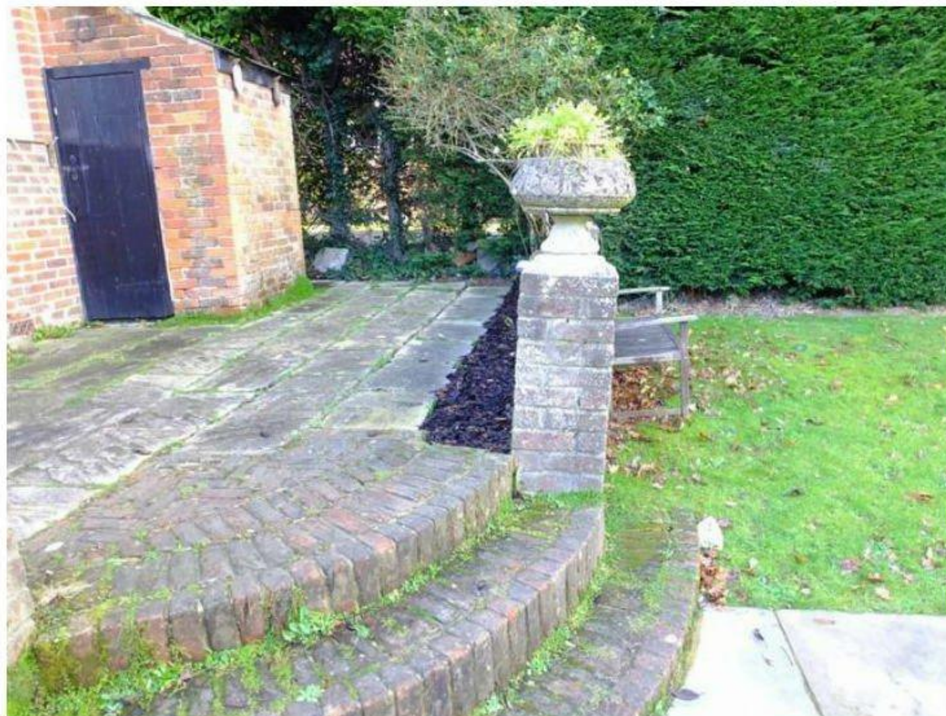
Image 4 Existing wall on west side that is going to be match on east side
