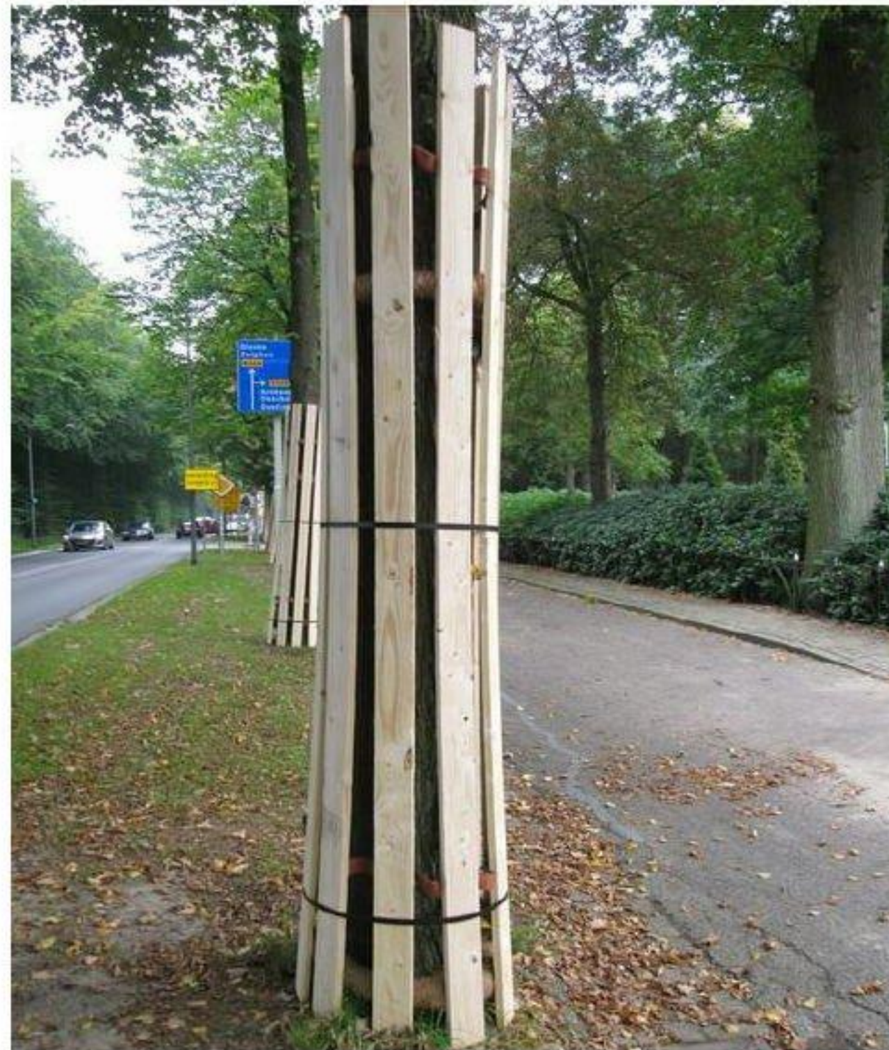
Figure 5 Tree Trunk Protection Measures
