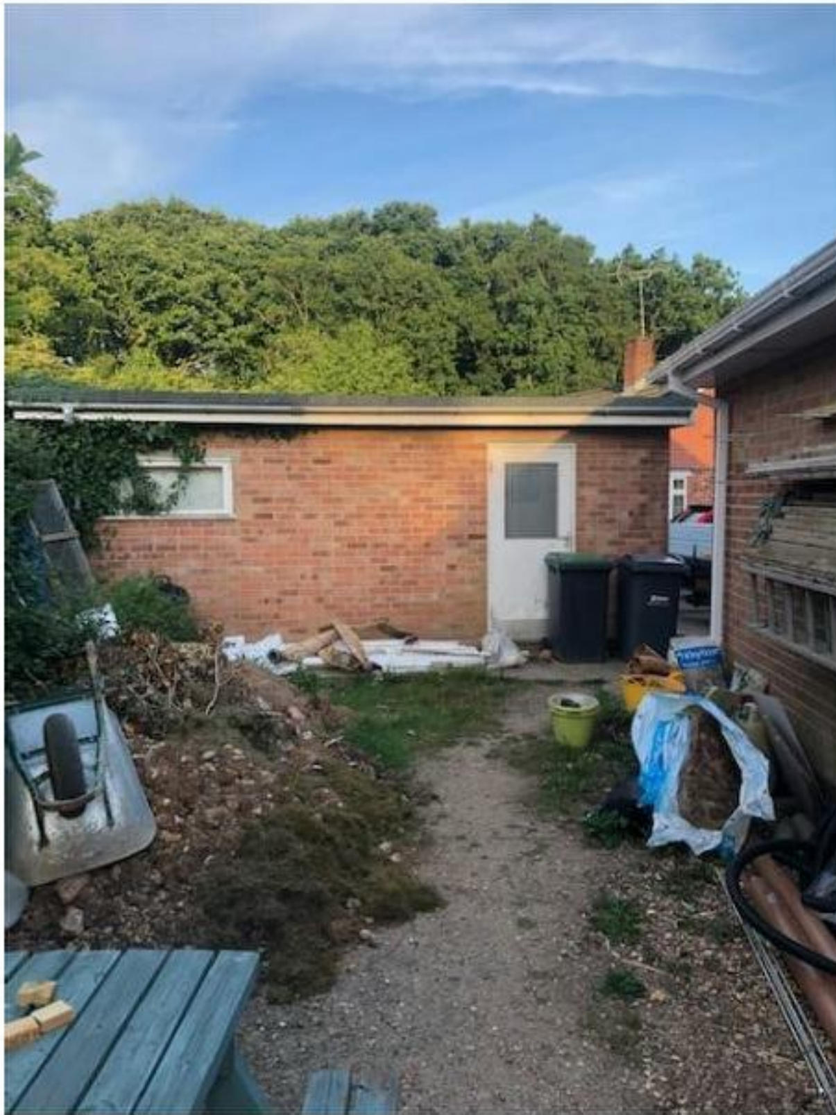
Photo 5: Side view of existing garage
