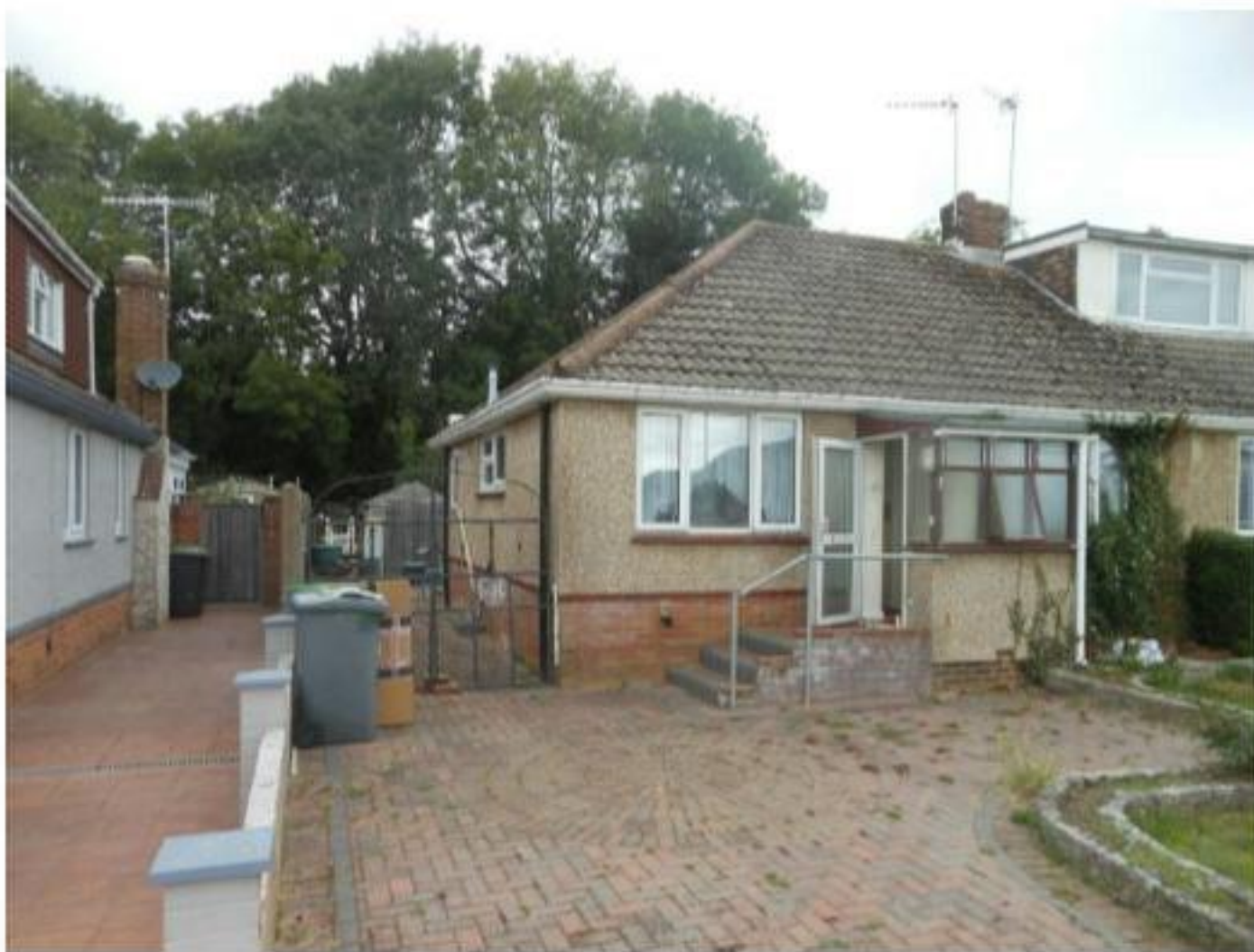
Photo 4: Front of property
