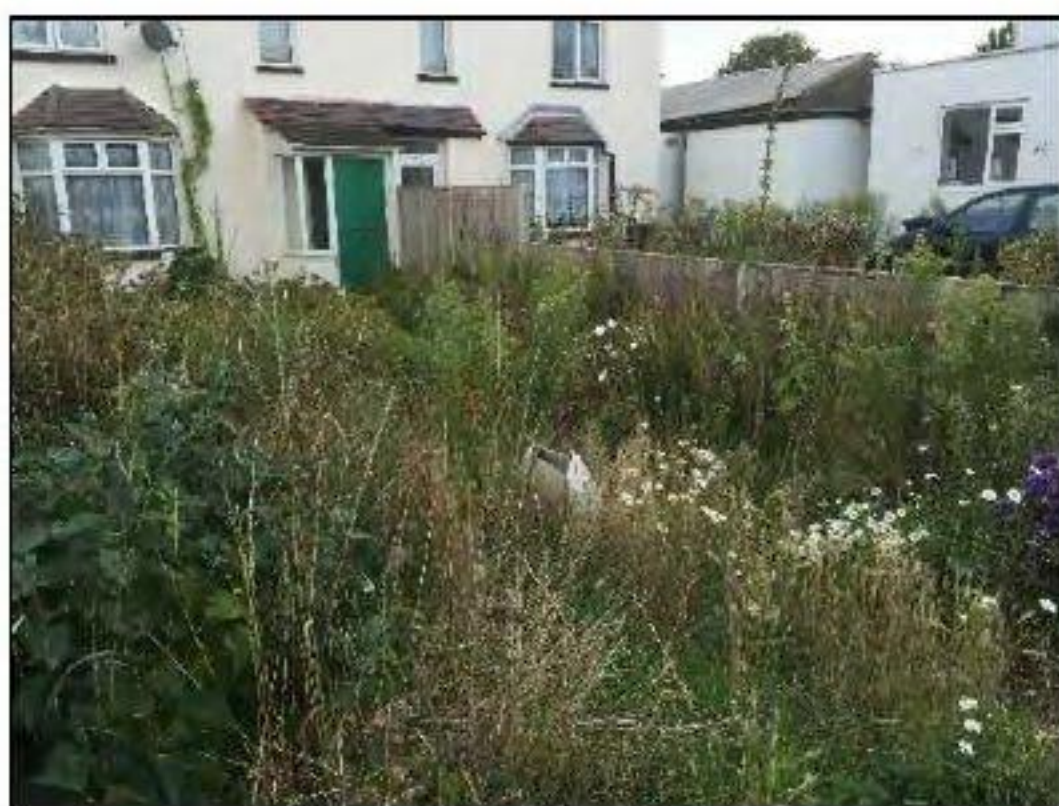
Figure 3: Disused gardens on southern elevation of former dwellings
