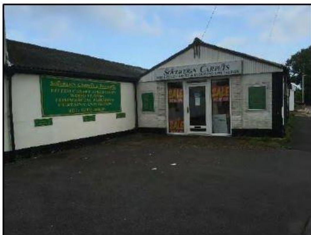
Figure 7: Eastern elevation of commercial unit on West Lane looking north
