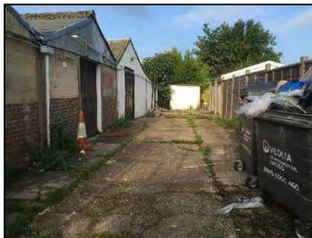
Figure 8: Rear northern elevation of commercial unit looking west
