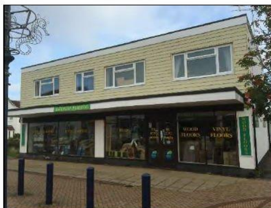
Figure 6: Southern elevation of commercial unit on Station Road
