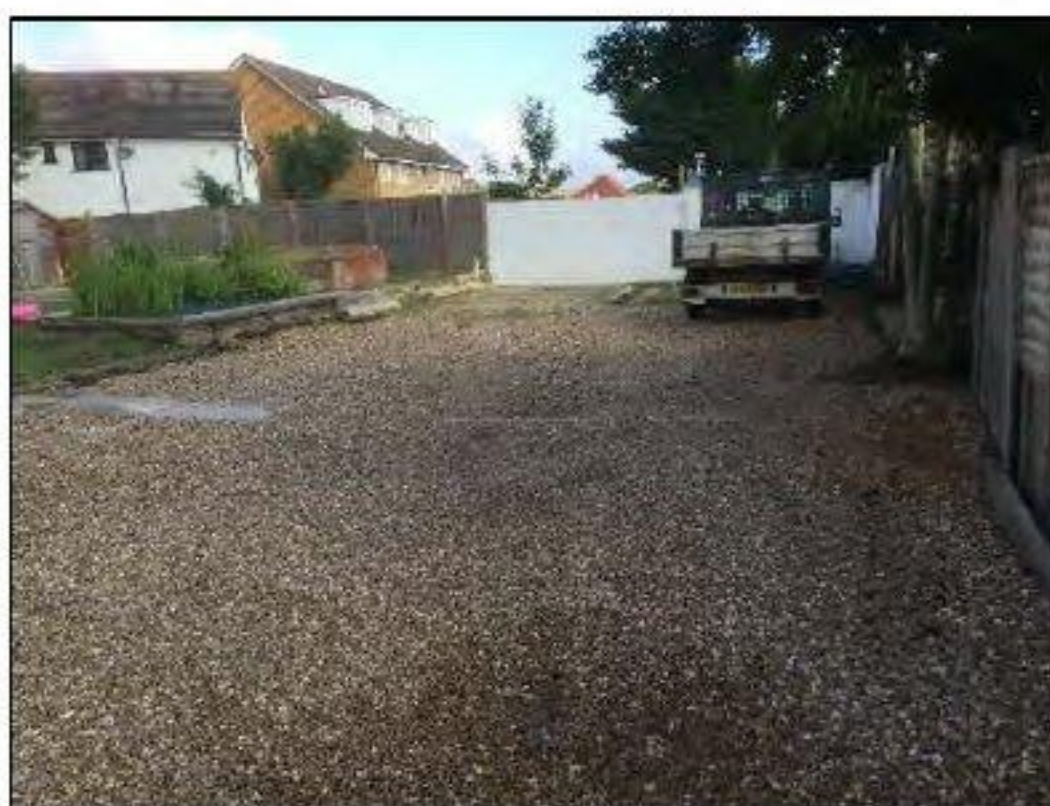
Figure 9: Gravelled hardstanding in northern area of the site
