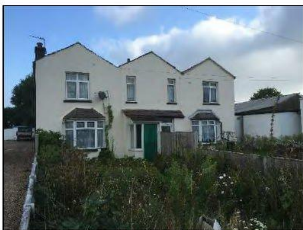
Figure 5: Southern elevation of former dwellings
