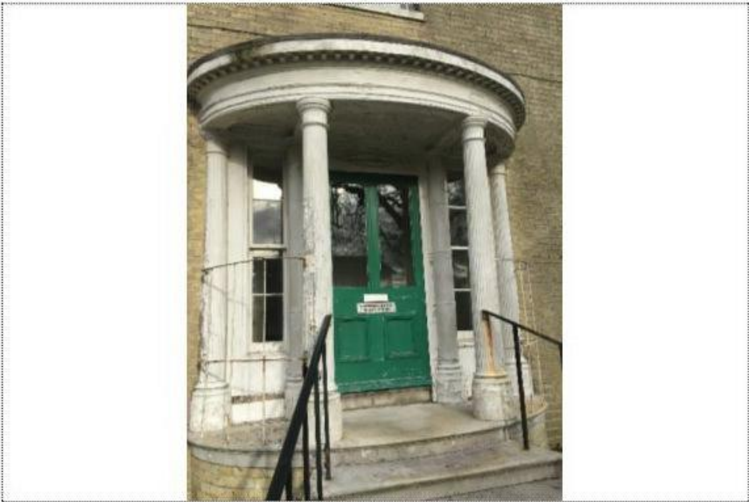
Photograph 8 - South Elevation Entrance Porch
