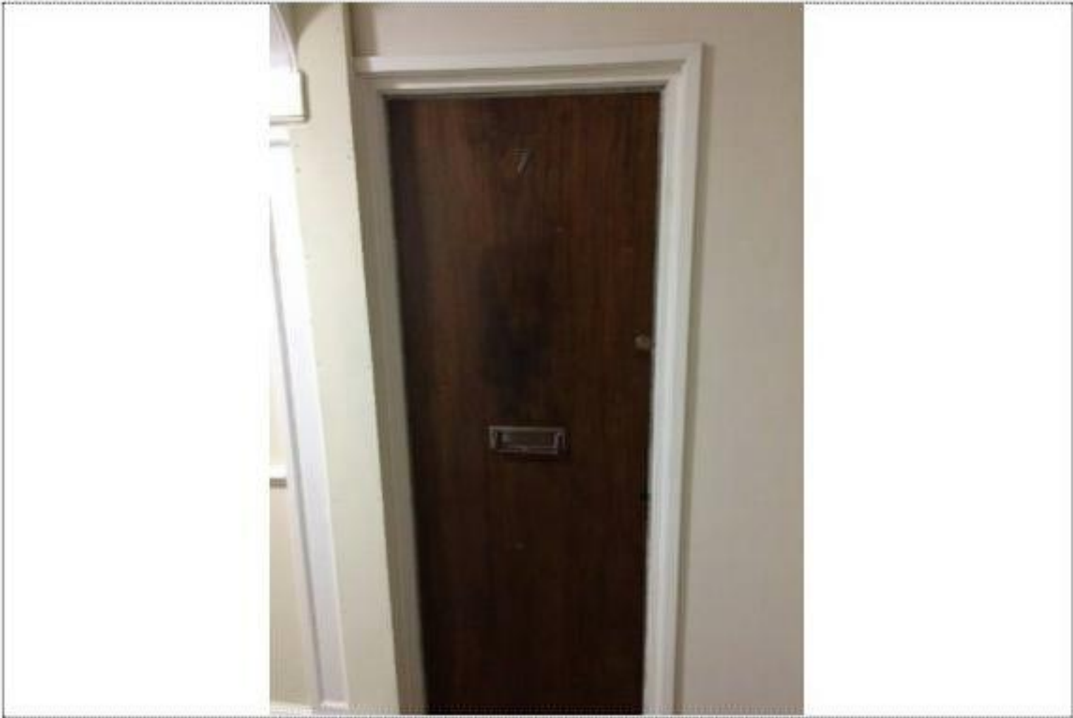
Photograph 33 - Flat 7 Entrance Door
