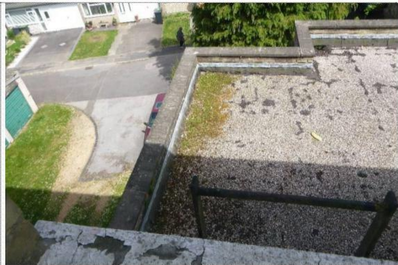
Photograph 24 – Single Storey Extension Flat Roof
