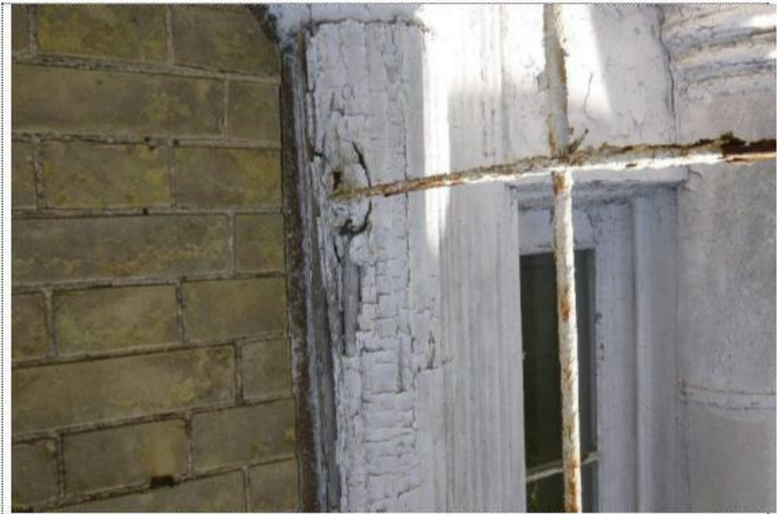
Photograph 10 - South Elevation Railing
