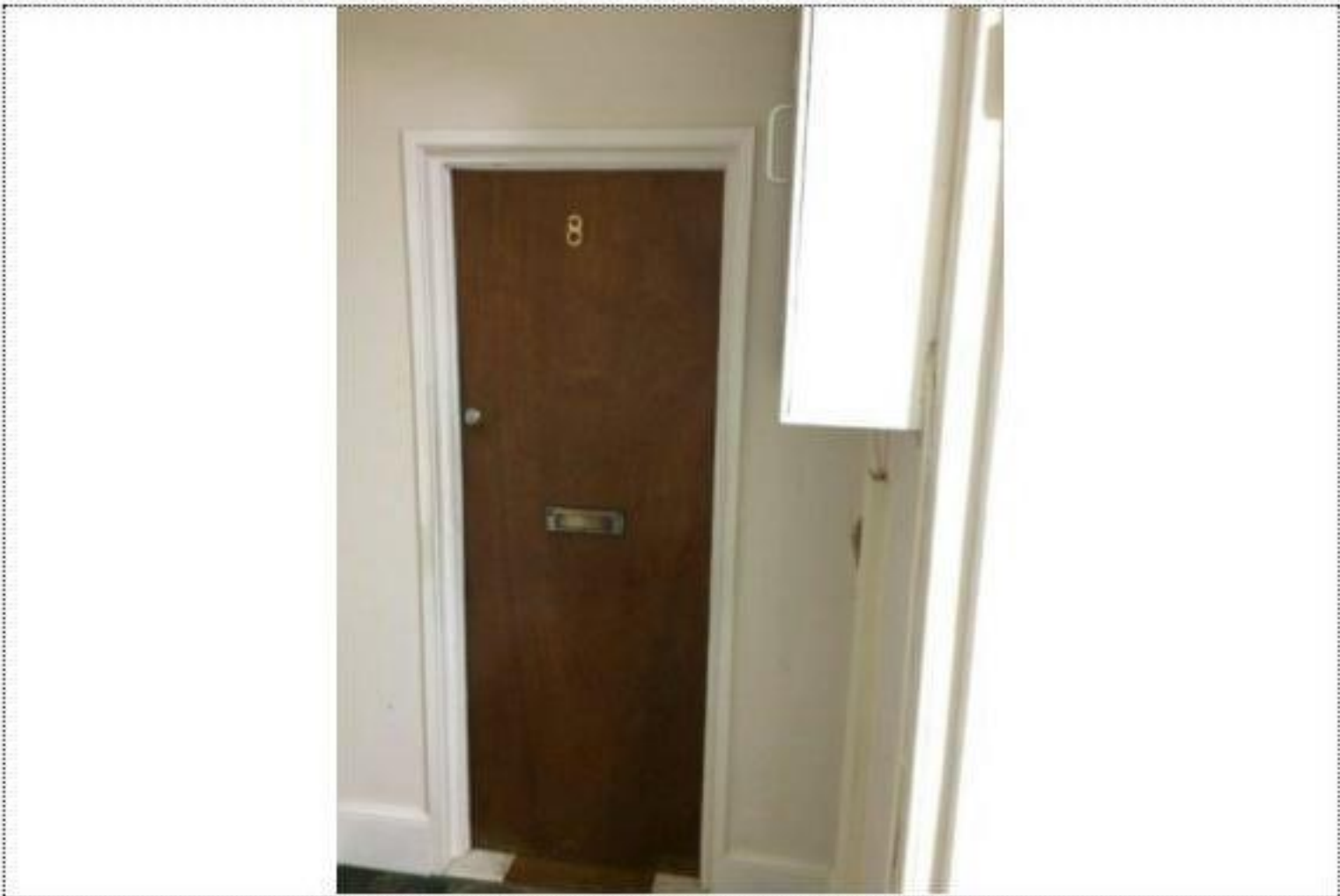
Photograph 34 - Flat 8 Entrance Door
