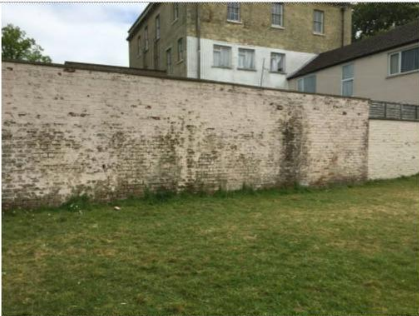
Photograph 14 - West Elevation – Rear of Garage Block
