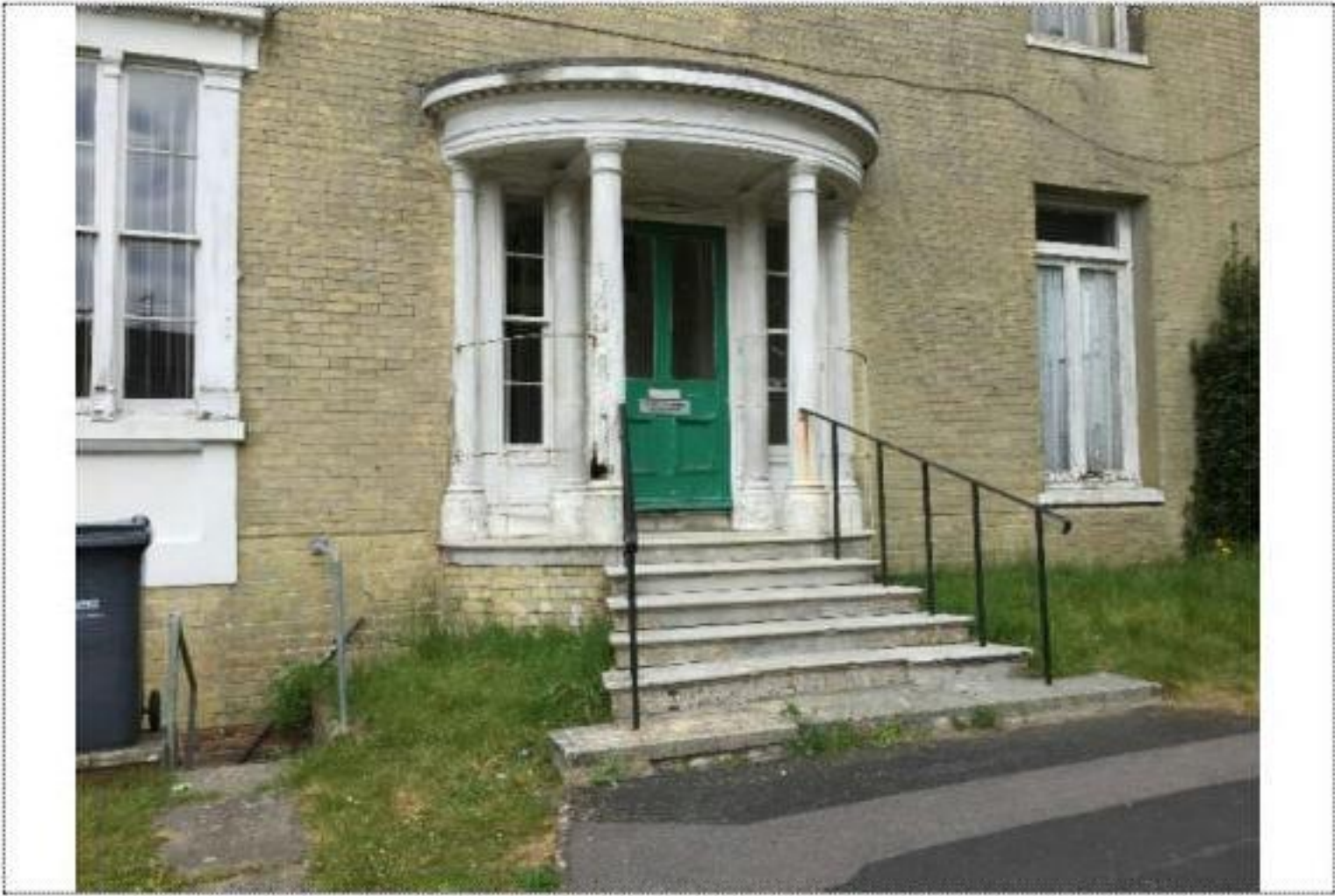
Photograph 7 - South Elevation Entrance
