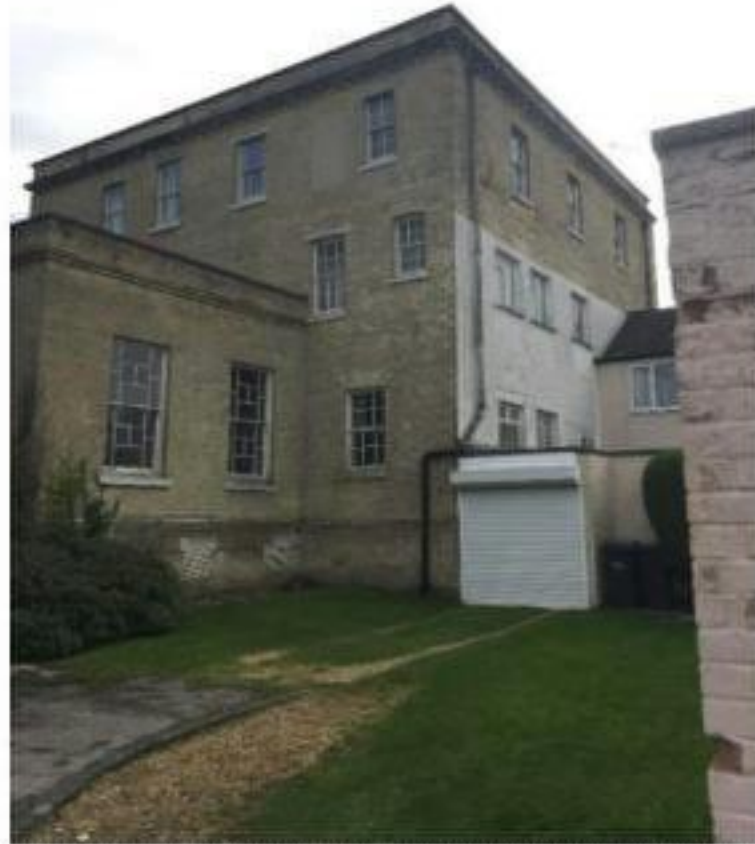
Photograph 13 - South and West Elevations
