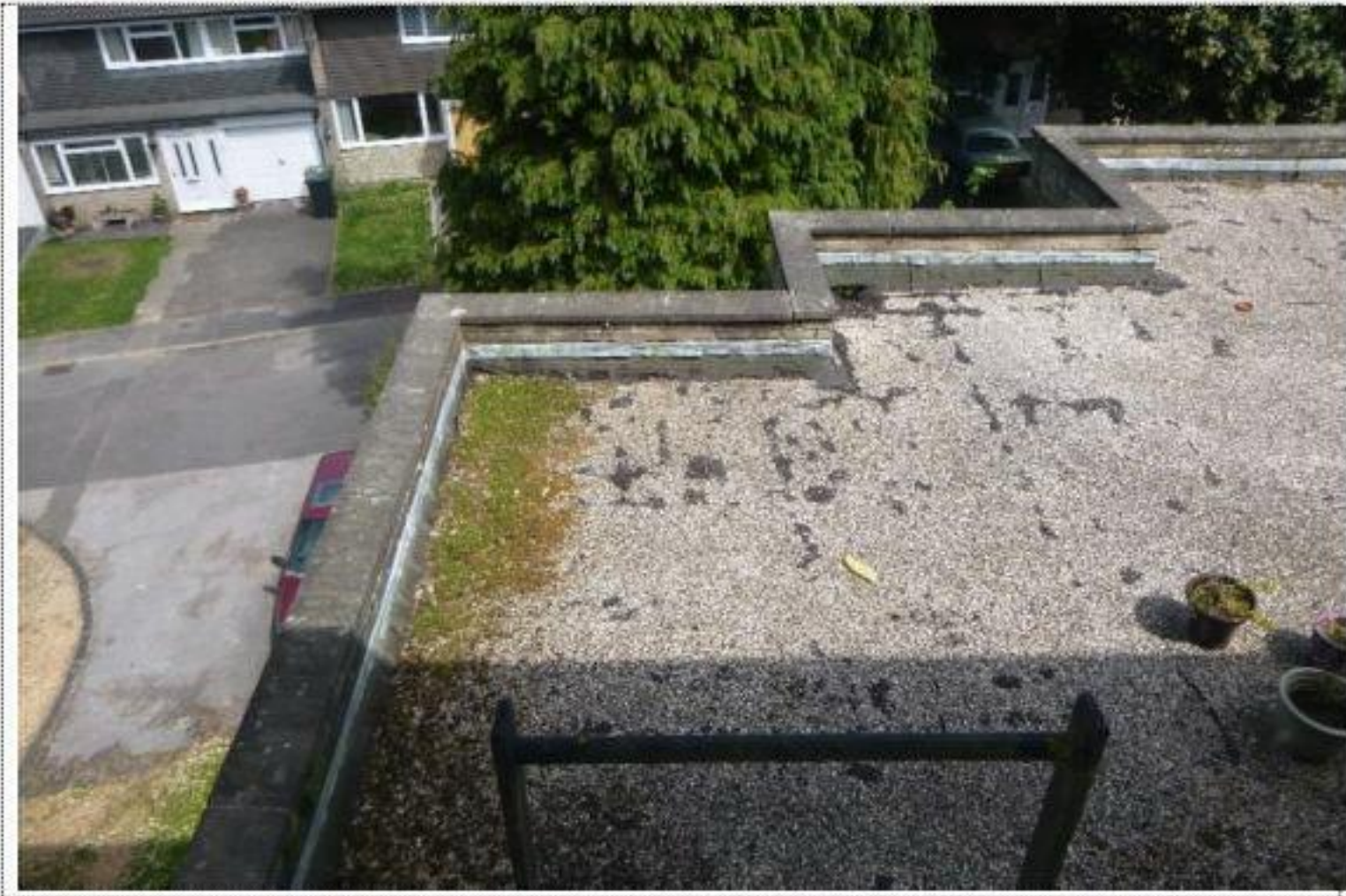
Photograph 23 – Single Storey Extension Flat Roof
