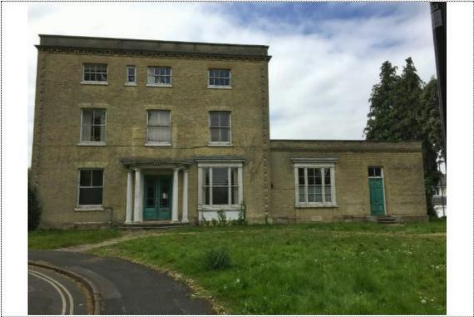
Photograph 1 - Front (East) Elevation
