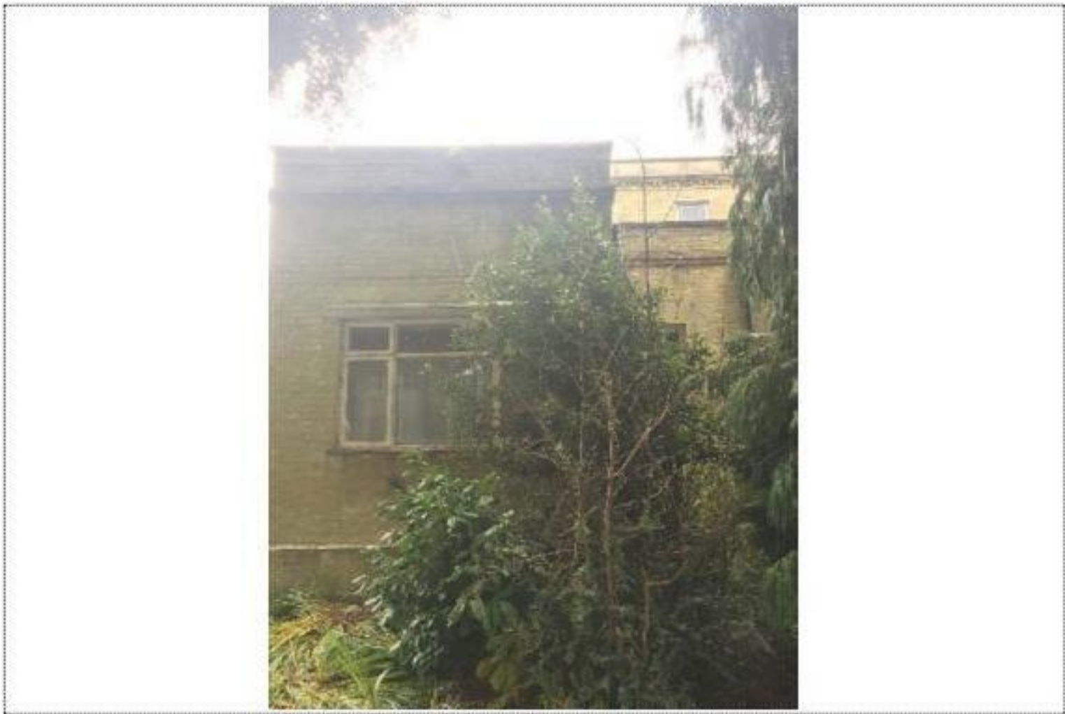
Photograph 19 - North Elevation of Single Storey Extension
