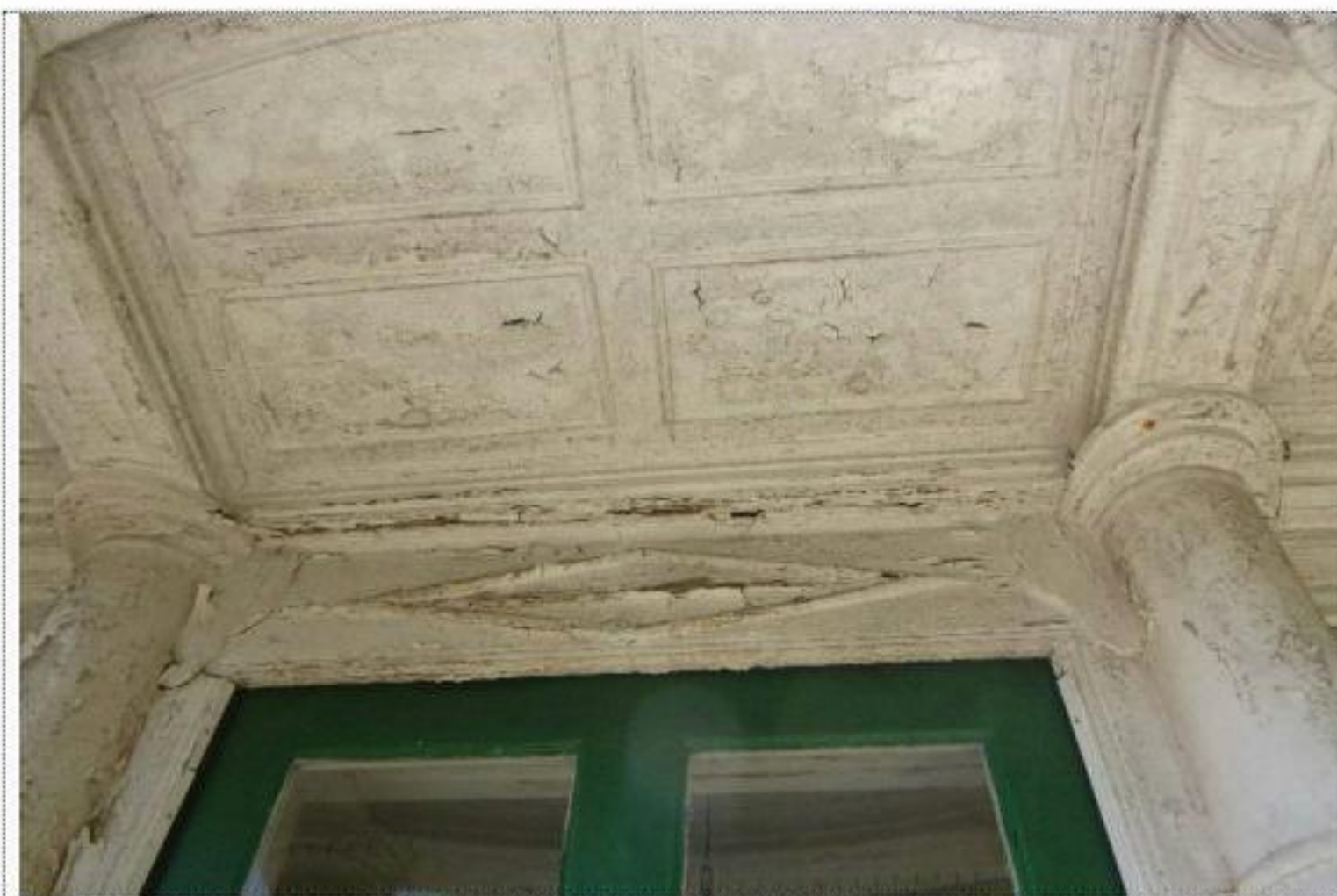
Photograph 11 - South Elevation Canopy Soffit
