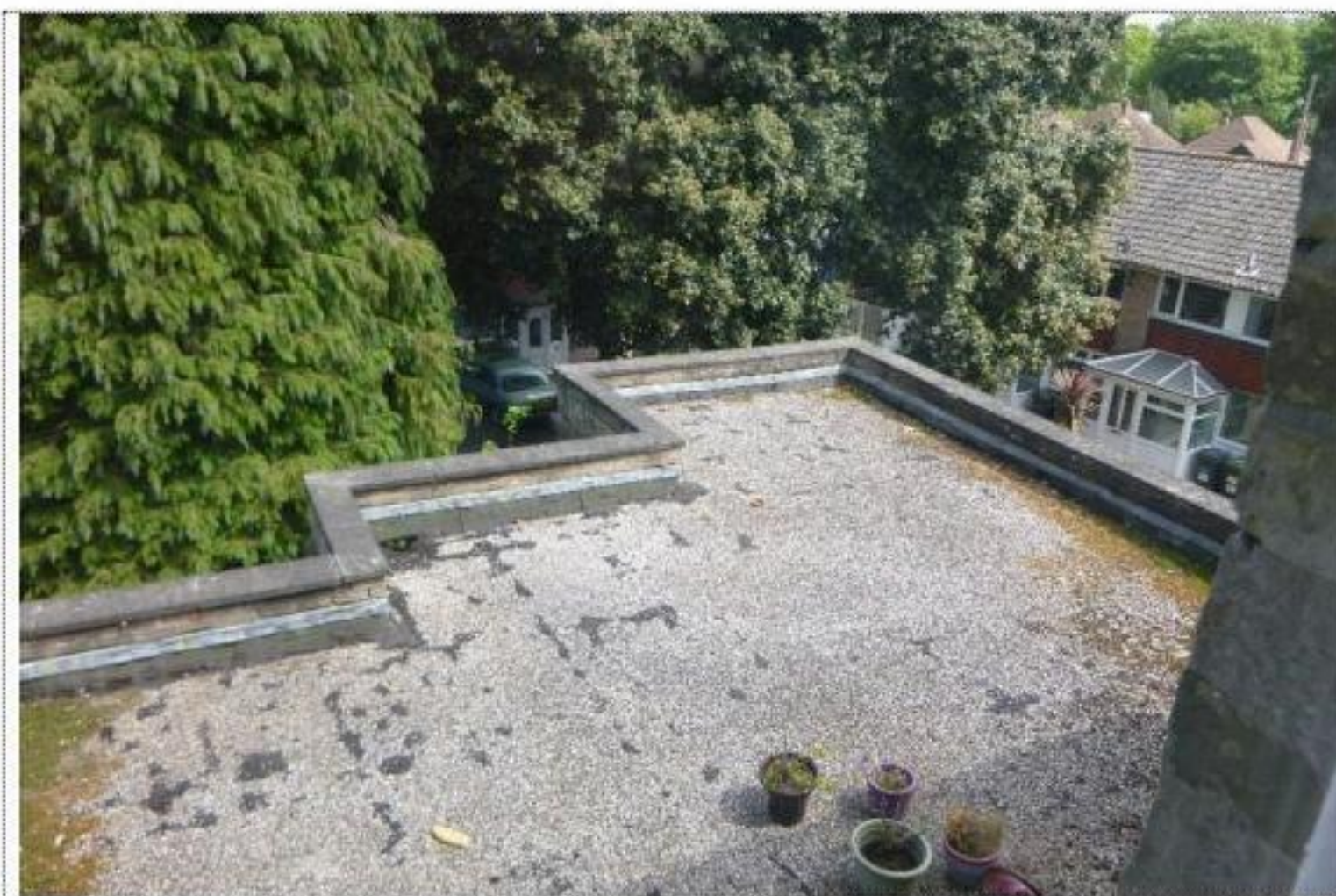
Photograph 21 – Single Storey Extension Flat Roof
