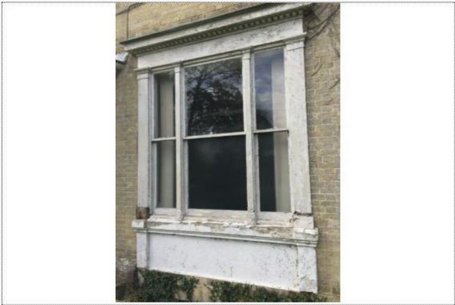
Photograph 3 - Front (East) Elevation Sash Window
