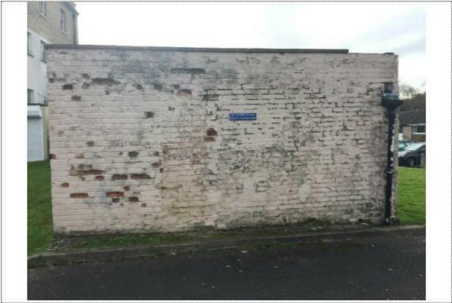
Photograph 15 - North Elevation of Garage Block
