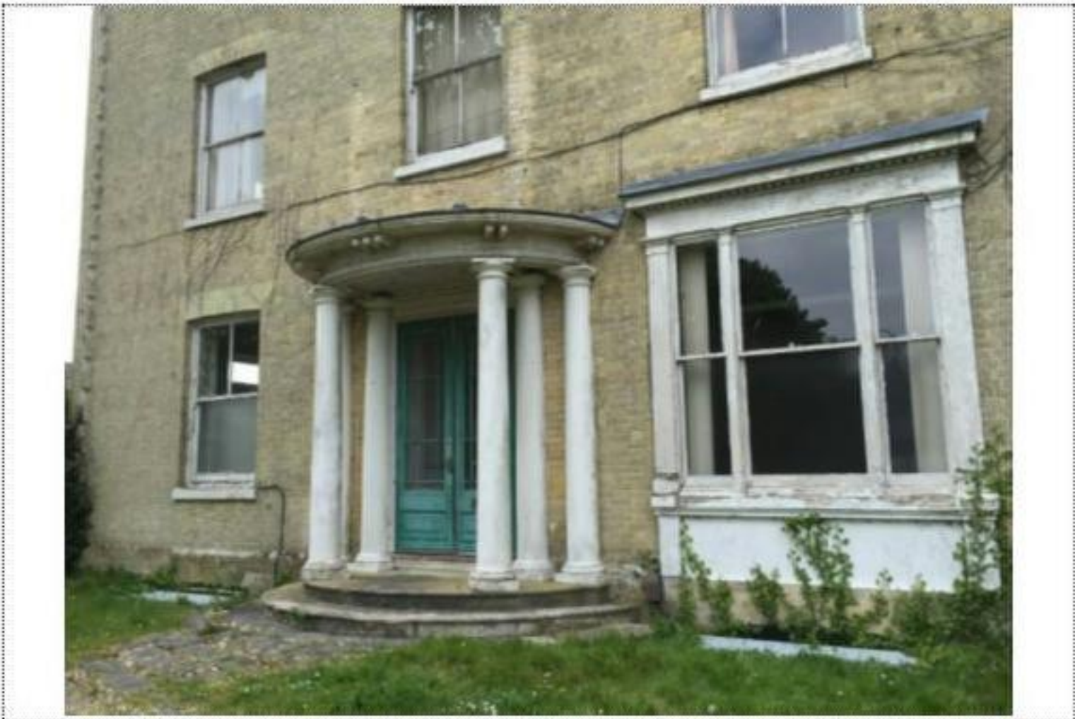
Photograph 2 - Front (East) Elevation
