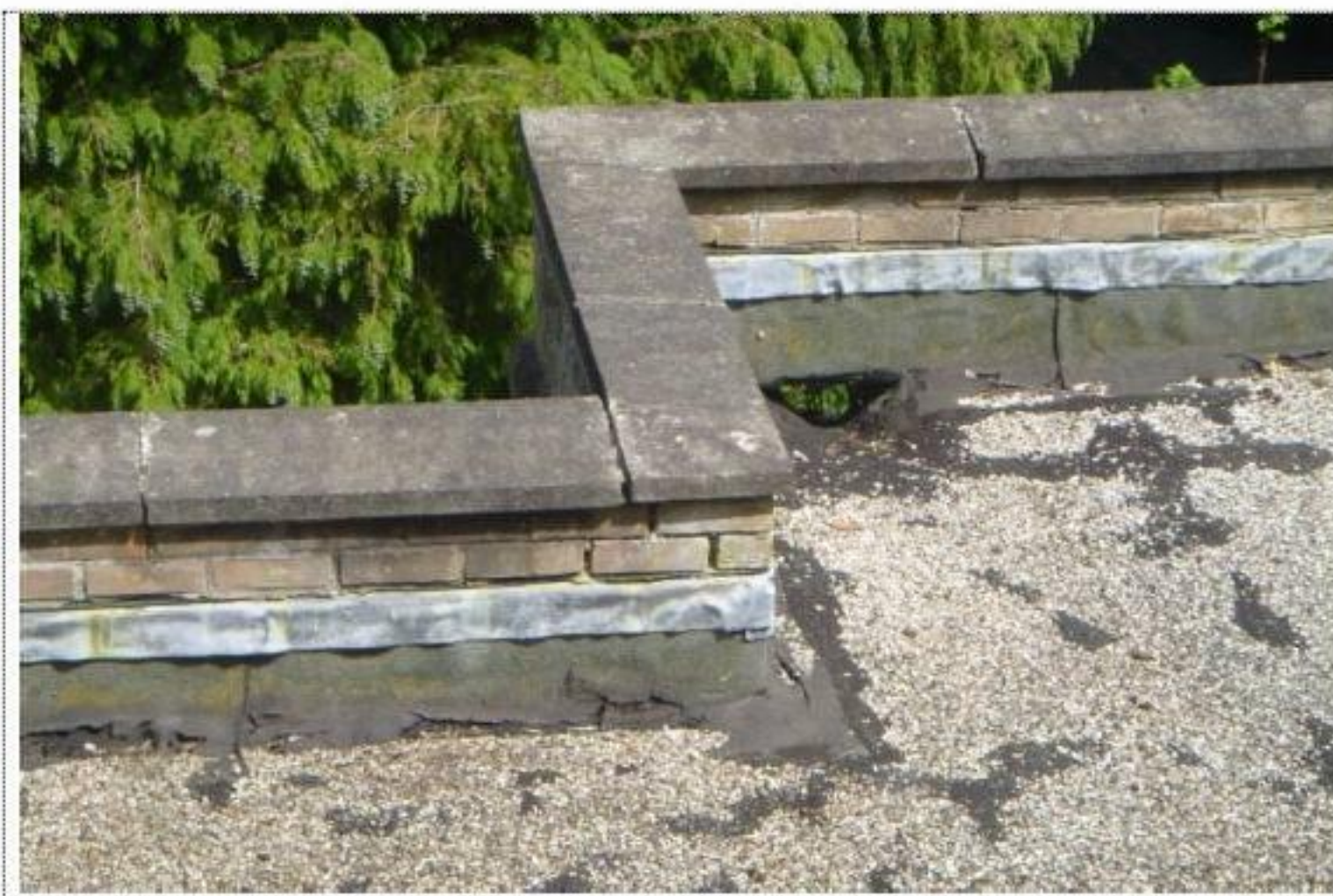
Photograph 25 – Single Storey Extension Flat Roof Upstands
