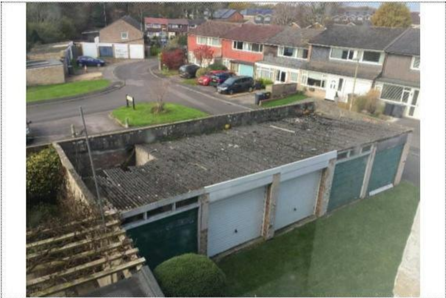
Photograph 18 - Garage Block Roof
