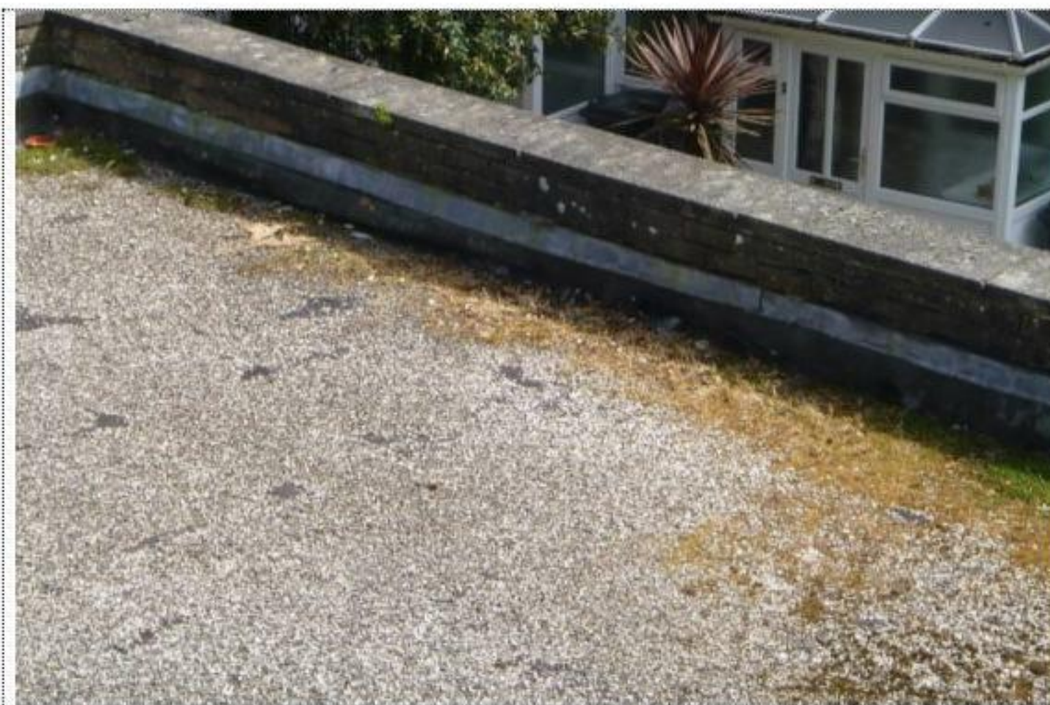
Photograph 26 – Single Storey Extension Flat Roof
