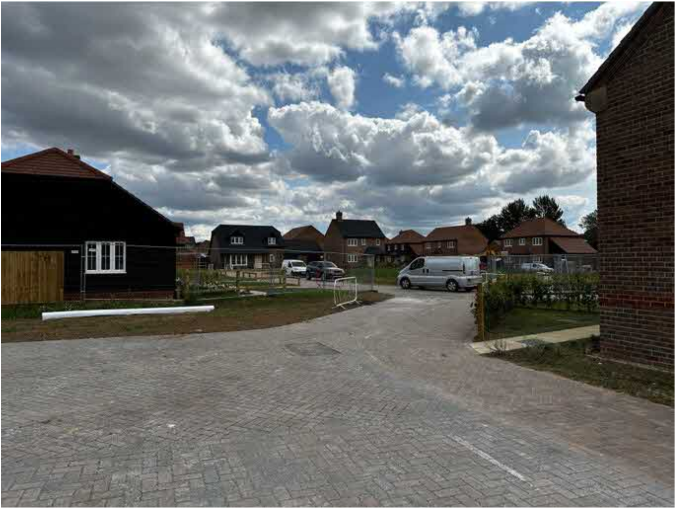
Parking area built out in north-western part of Phase 1.
