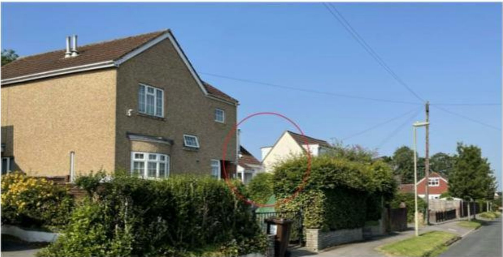
West facing – circle indicating where extension would be
