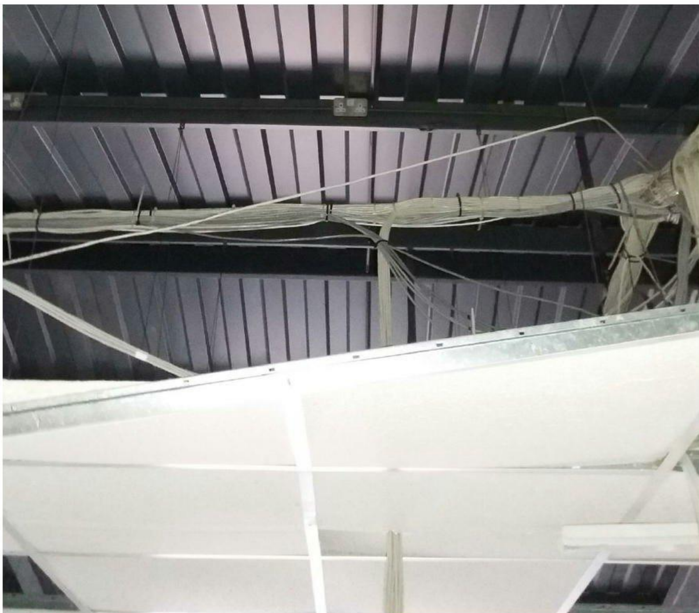
Photo 5 Roof cavity of the building above the suspended ceiling
