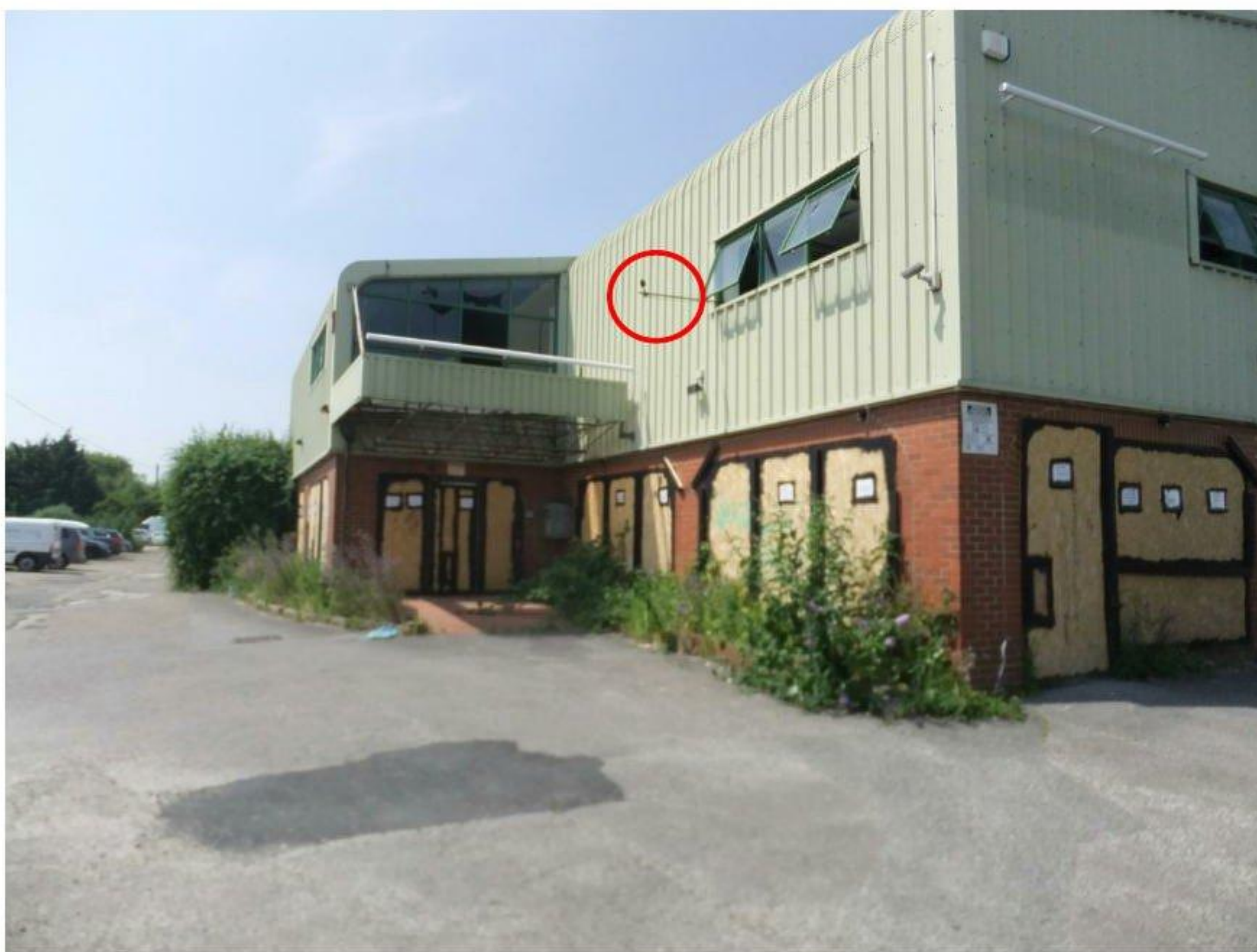
Photo 2 Long term measurement location – on façade facing access road
