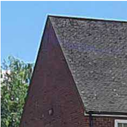
Front-Back Pitched roof with Grey Tiles
