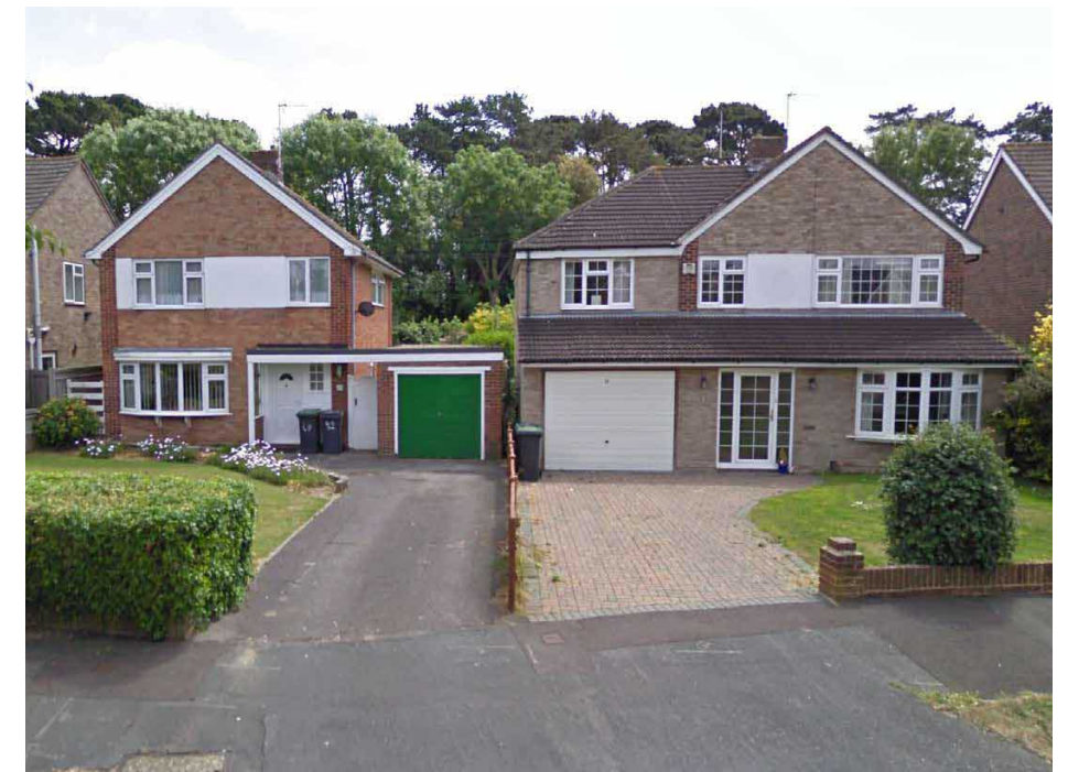
Detached Houses Southbrook Road, Havant
