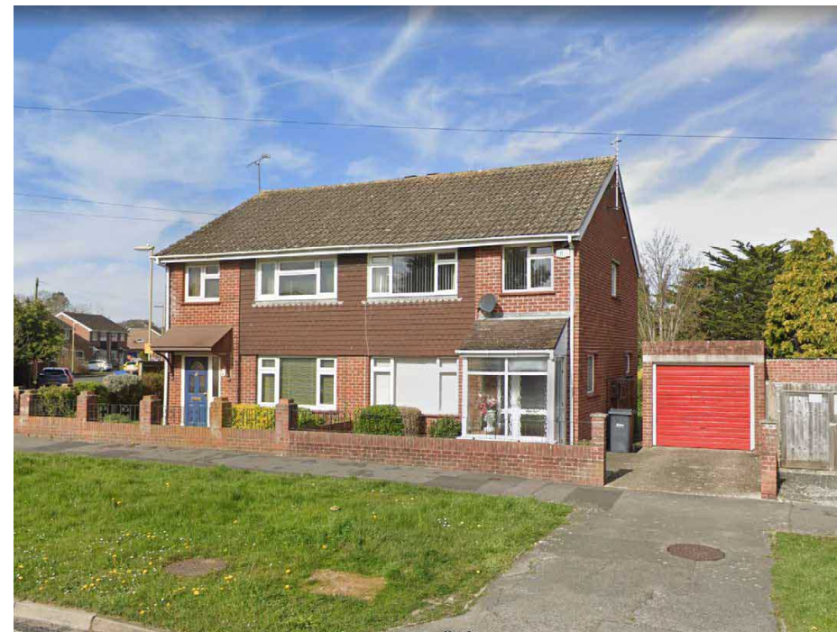
Semi-Detached Houses Park Lane, Havant
