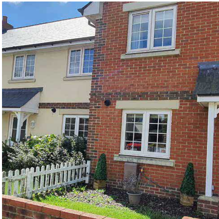
Feature Brick Detailing to Front
