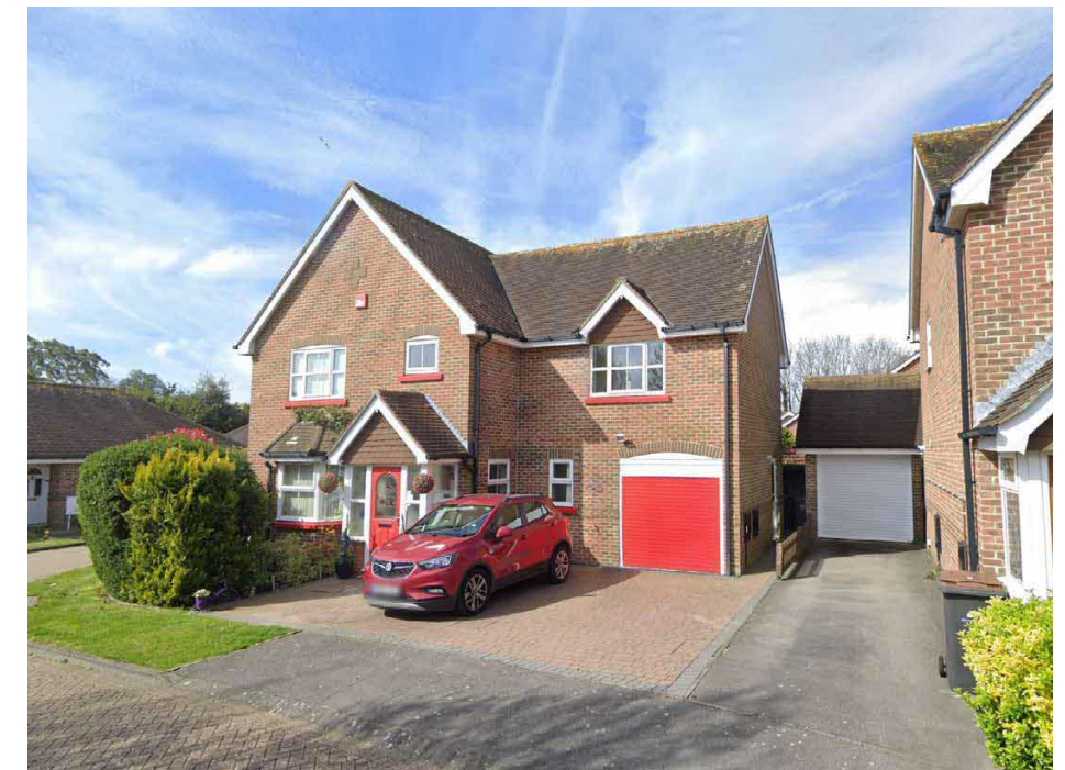
Detached House Tulip Gardens, Havant
