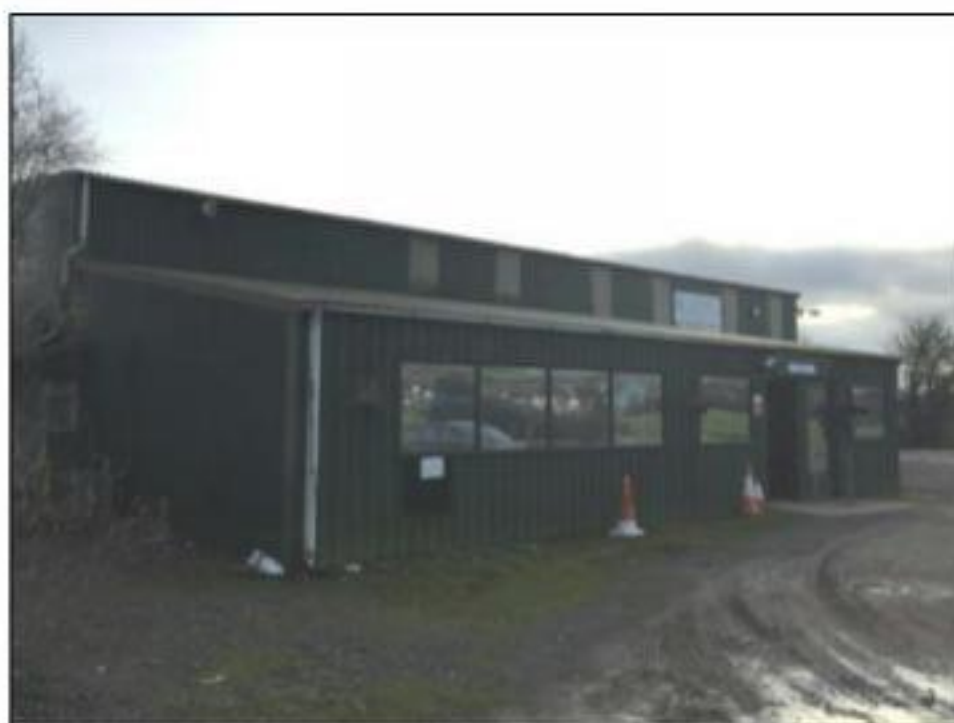
Photograph 24: Main commercial building (07) located in the industrial area.
