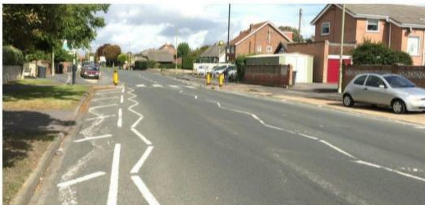
Figure 2.3: The A3023 Beach Road Looking North
