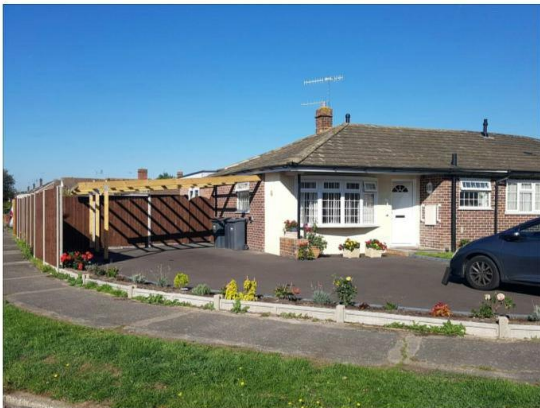
Front of 30 Inhurst Avenue
