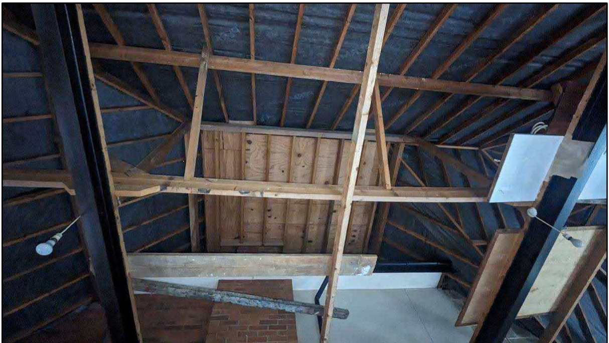
Photo 6 –The roof void in the boat garage,
