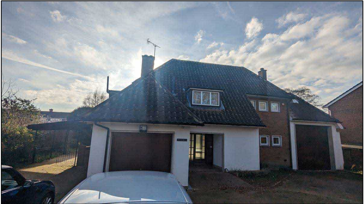
Photo 1 –View of the dwelling from the north looking from to the access point.
