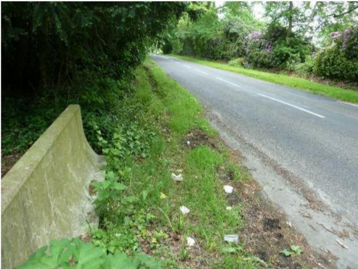
PHOTOGRAPH N: Eastleigh Road Drainage Ditch (eastern verge), looking south from the southern vehicle access
