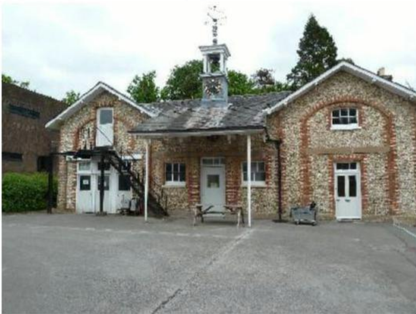
PHOTOGRAPH L: The Stables Building, looking east
