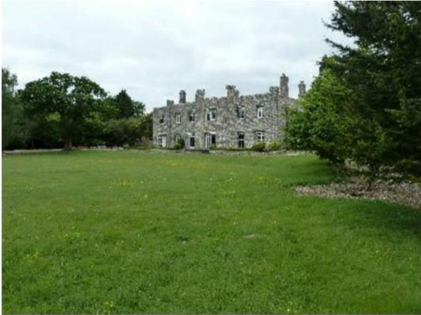
PHOTOGRAPH G: Southleigh Park House, looking northwest from the south-eastern corner of the site
