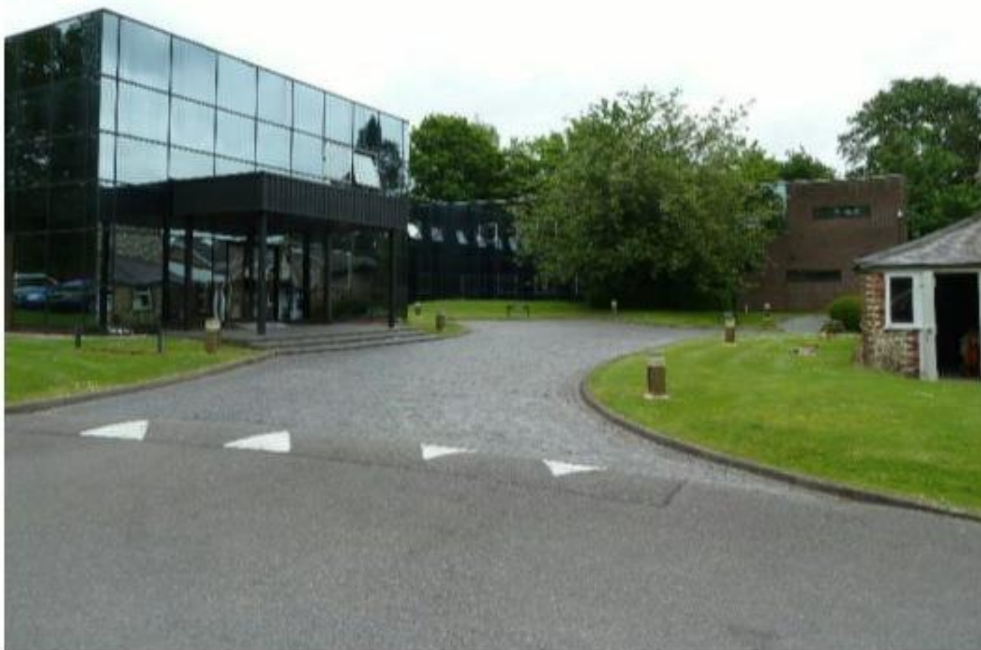
PHOTOGRAPH A: Main Office Building Entrance, looking northeast from the Eastleigh Road vehicle access
