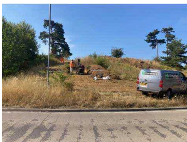
Slope levelled to enable window sampler at WS5. A ramp was formed to the right of WS5 to enable access to exploratory positions at the top of the fill.
