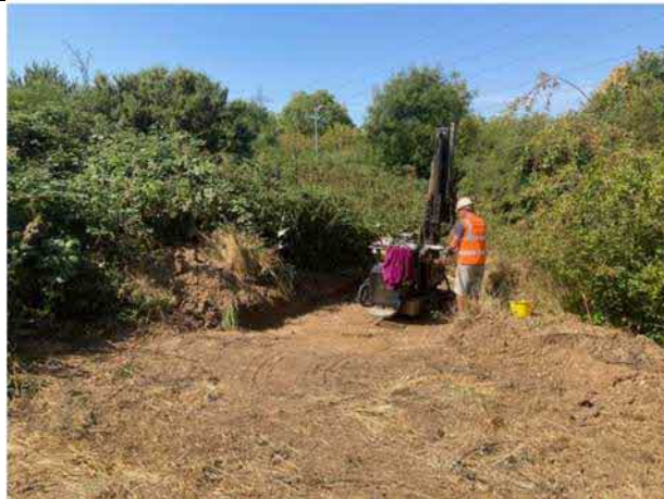
Vegetation clearance to give access to WS2
