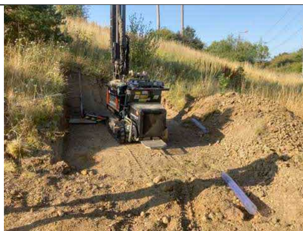
Slope levelled to enable window sampler at WS1. The ground level at the window sample position was reduced by approximately 1m.
