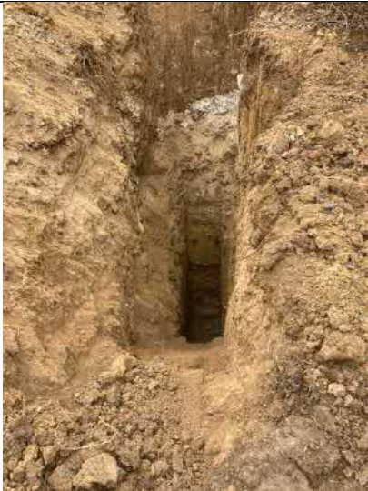
Location of CP3 following excavation of concrete obstruction
