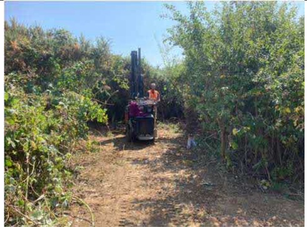
Vegetation cleared to give access to WS3
