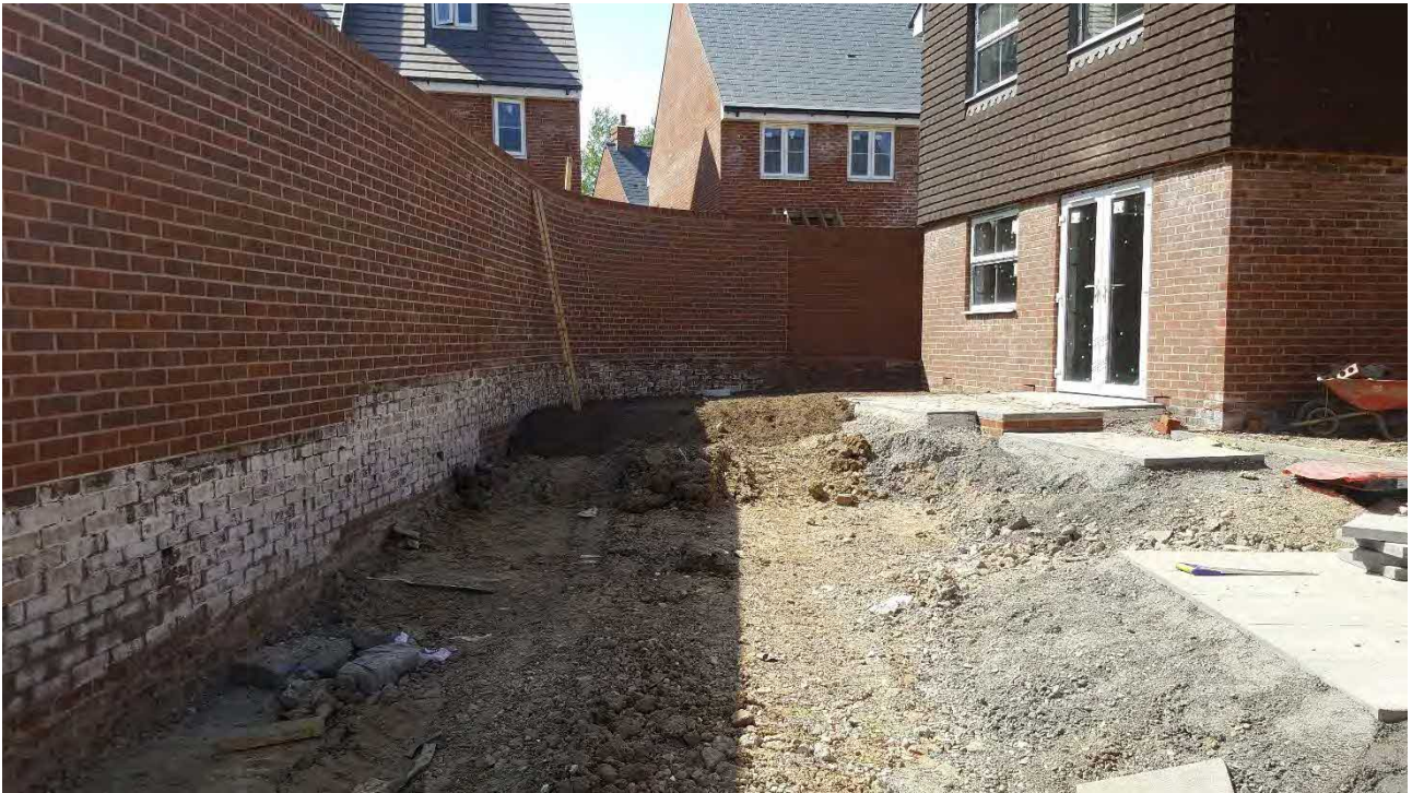
Plate 21 Reduced dig undertaken across Plots 24-27
