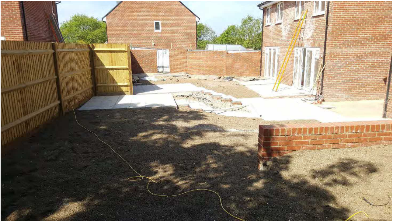
Plate 19 Completed rear garden areas of Plots 20-23
