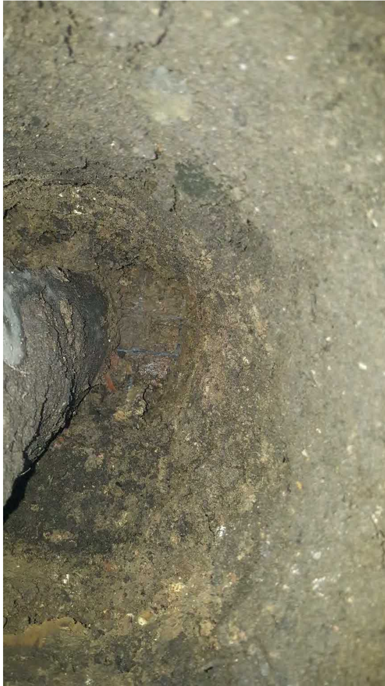
Plate 7 Plot 18 Geogrid beneath Subsoil and Topsoil
