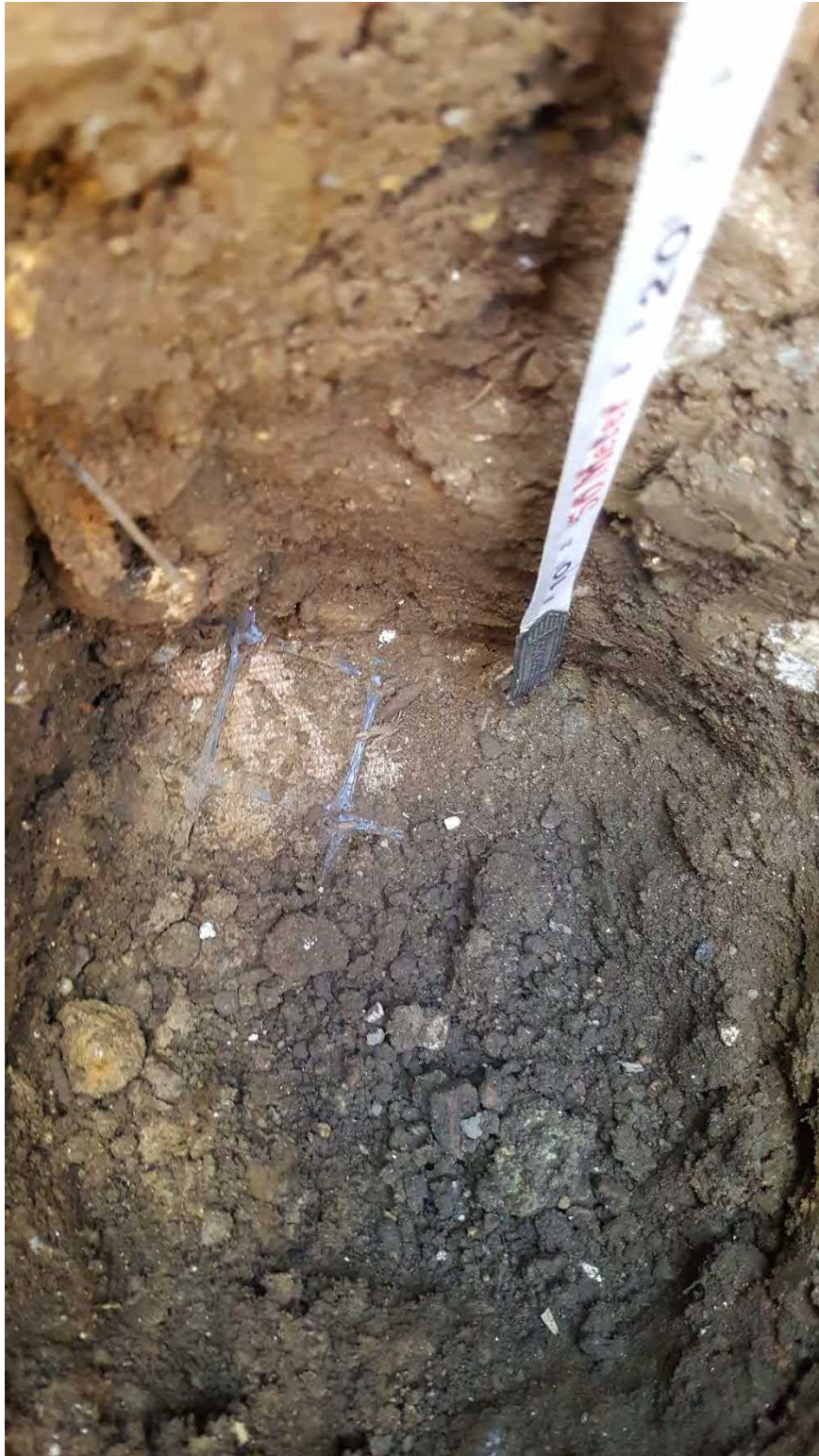
Plate 5 Plot 10 geo-grid and membrane beneath subsoil
