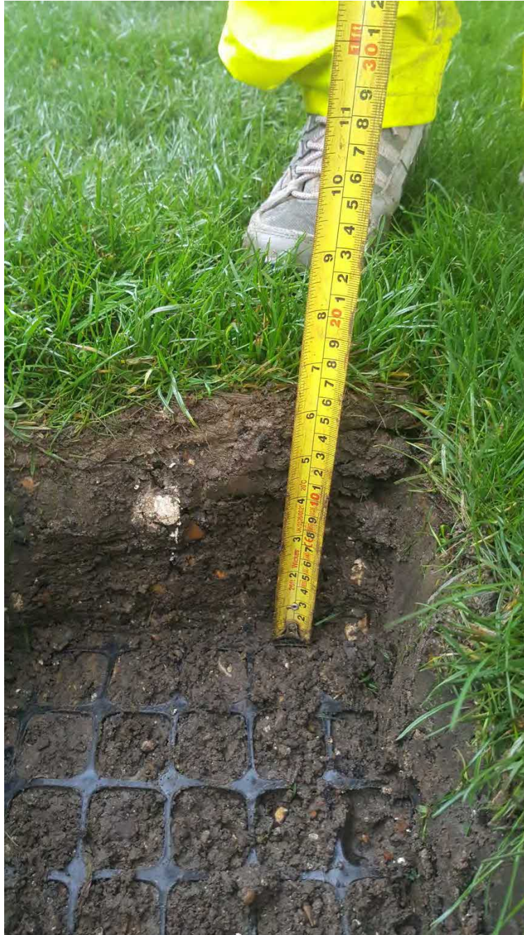
Plate 2 Plot 1-6 Pit between flats and railway cutting boundary
