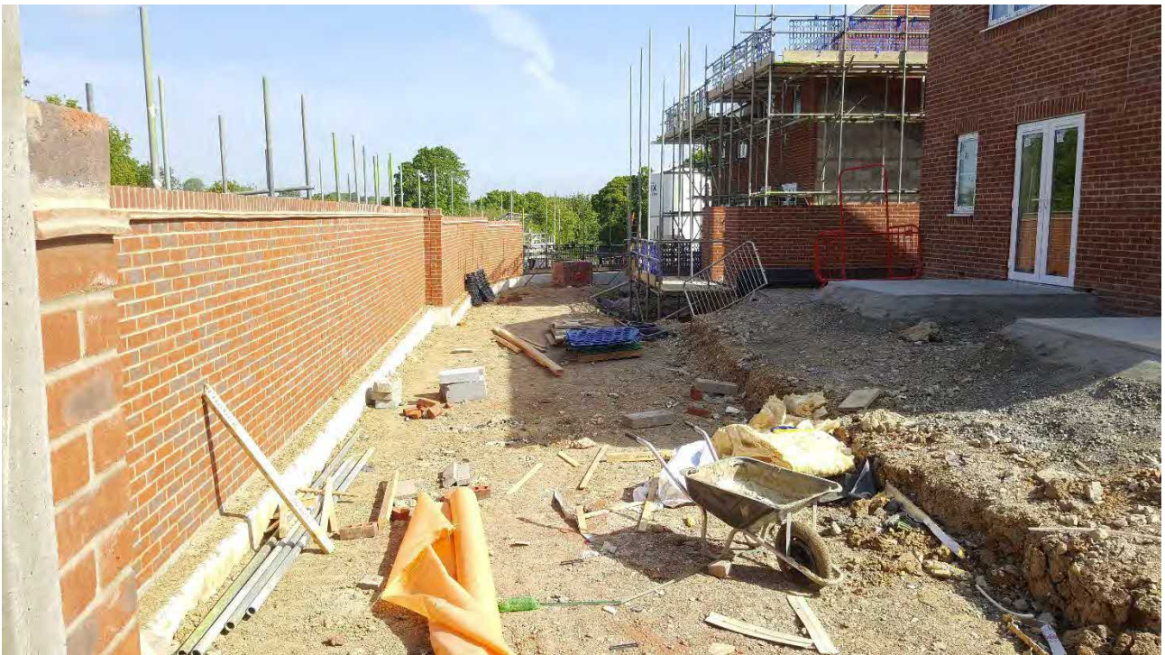
Plate 18 Reduced dig undertaken across Plots 13-16
