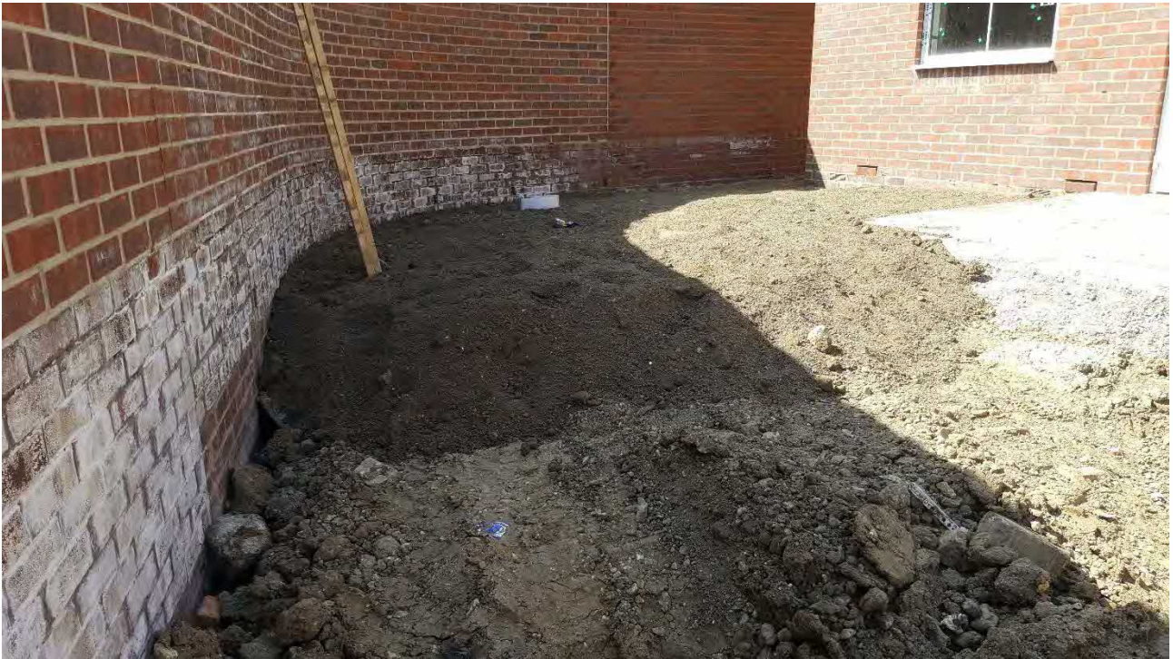
Plate 17 Plot 24 reduce dig and installation of Topsoil
