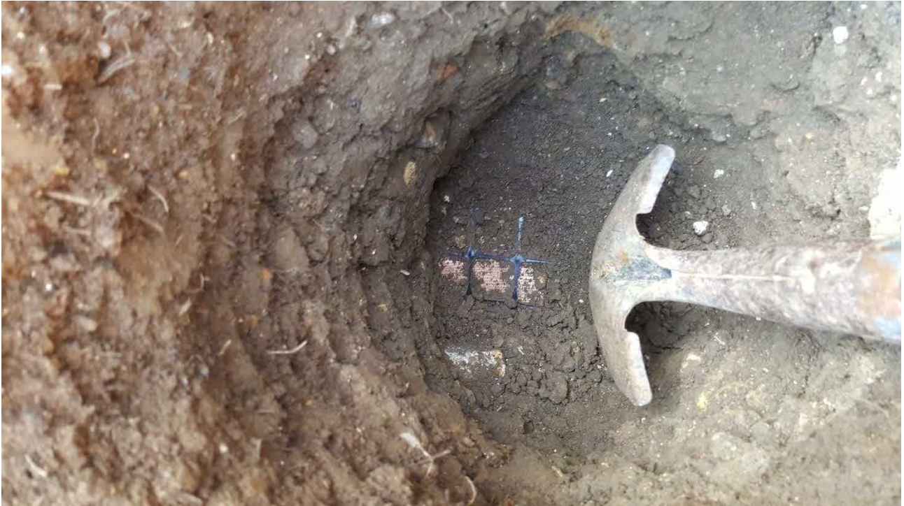
Plate 1 Plot 7 geo-grid and membrane beneath subsoil
