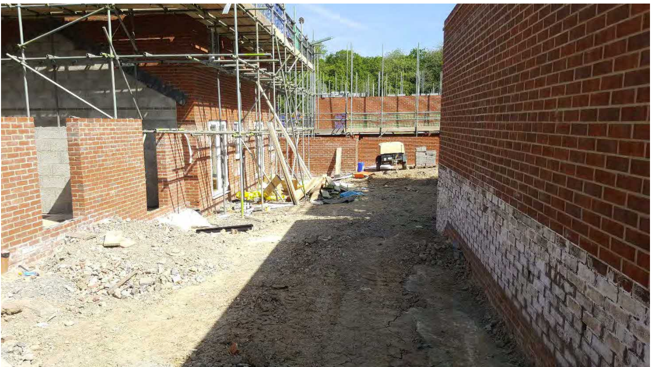
Plate 22 Reduced dig undertaken across Plots 24-27
