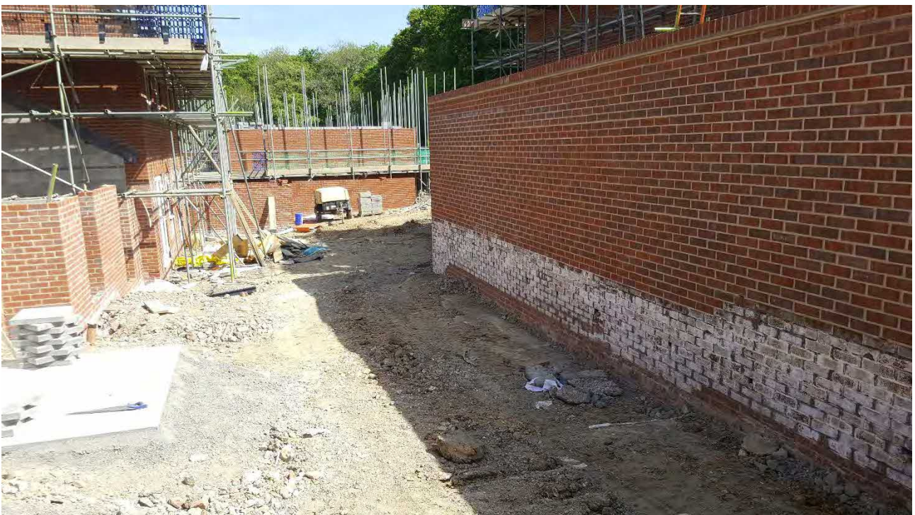
Plate 20 Reduced dig undertaken across Plots 24-27
