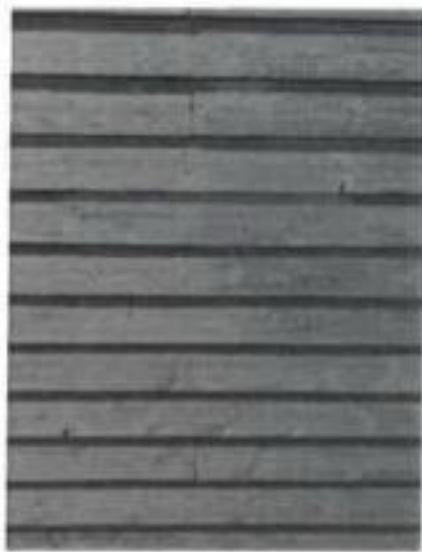
Black Timber Cladding
