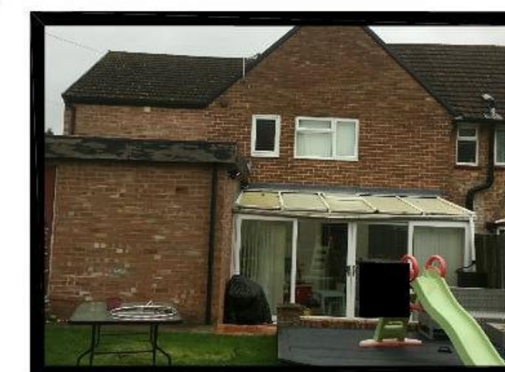
Photo - West Elevation
