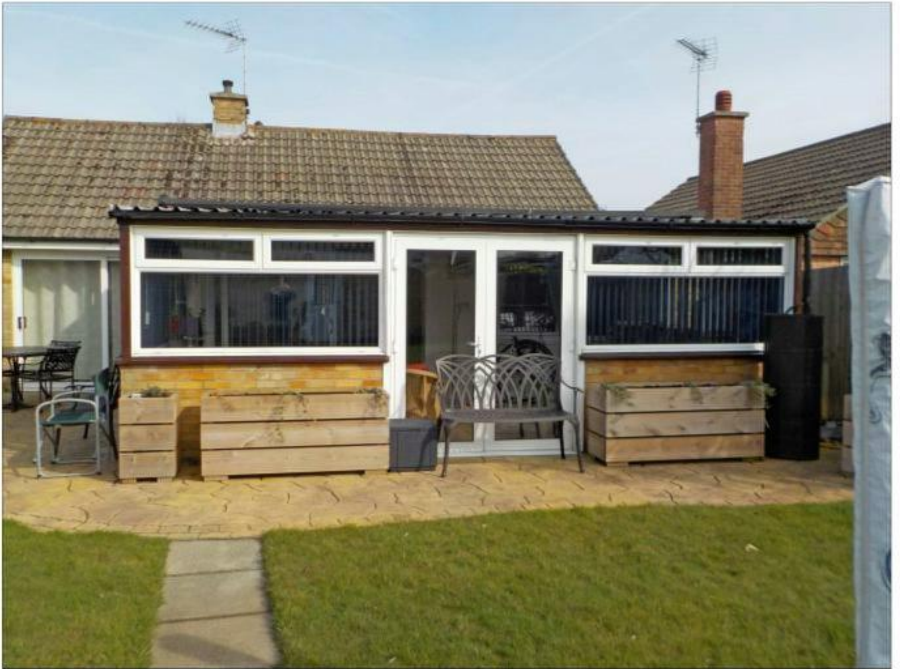
Rear of No. 48 Charlesworth Drive
