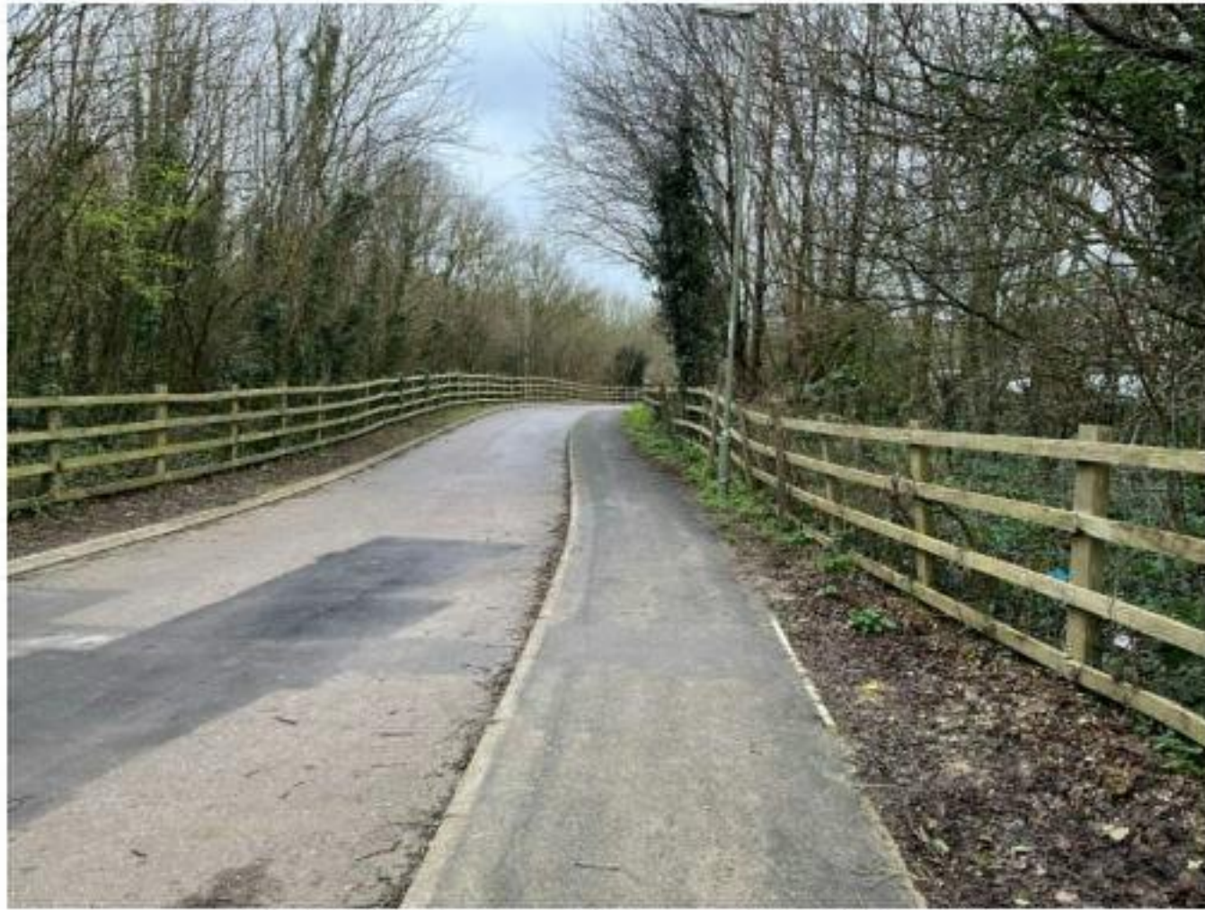
Photograph 2: Carriageway and footway conditions of Emsworth Rd
