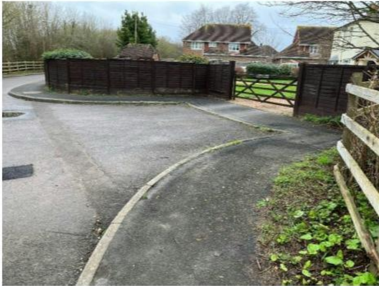
Photograph 3: Carriageway and footway conditions of Emsworth Rd
