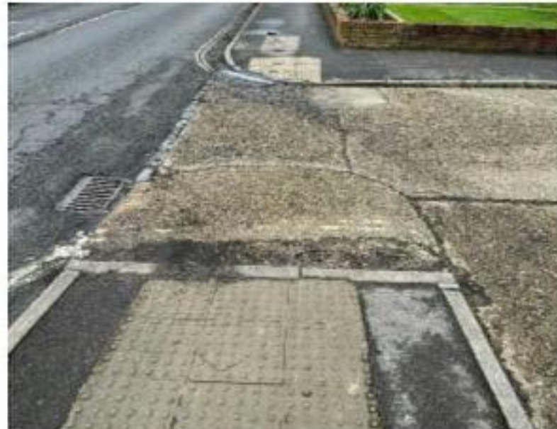
Photograph 11: Dropped kerbs and tactile paving at parking layby on Emsworth Rd
