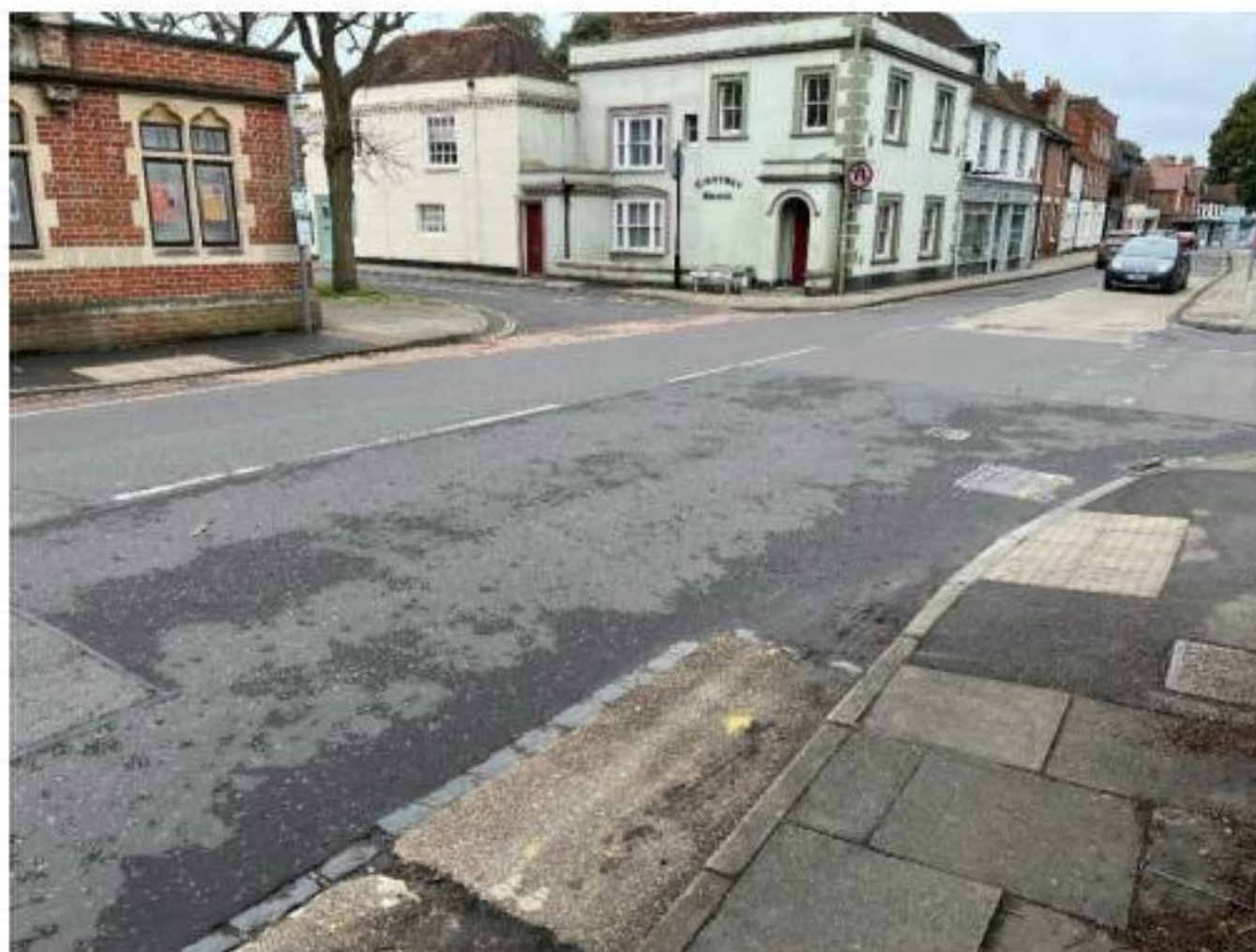
Photograph 12: East St tactile paving and dropped kerb crossing
