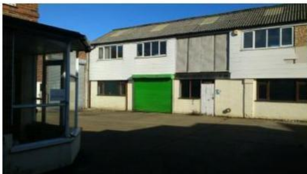
Two storey building looking east
