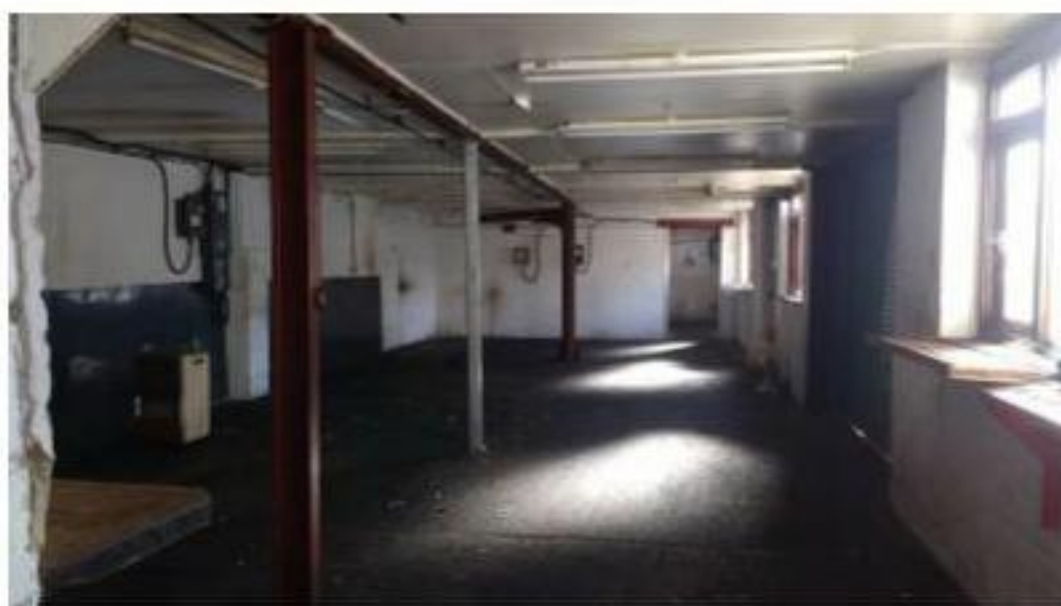
Internal ground floor two storey building looking south
