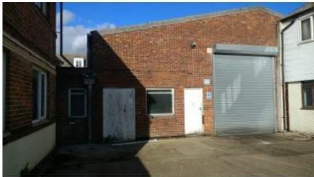
Full height building looking north
