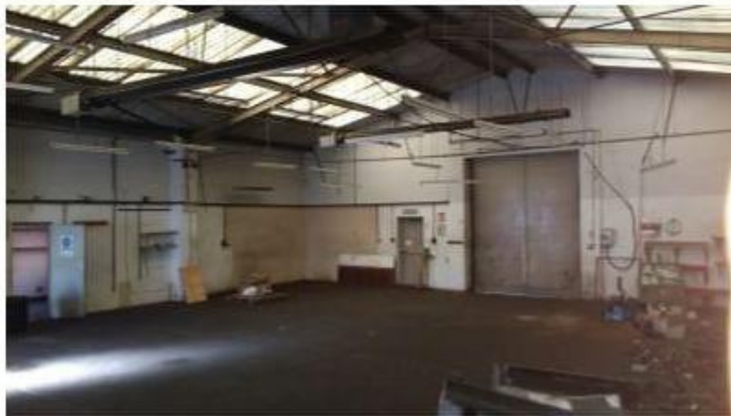
Internal parts full height building looking north
