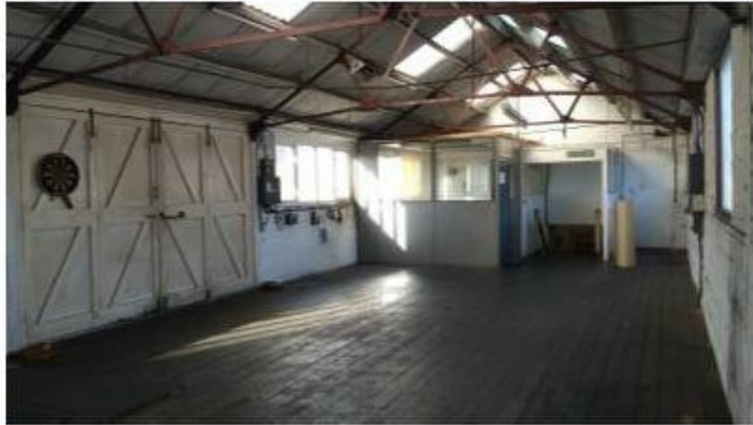
Internal first floor two storey building looking north
