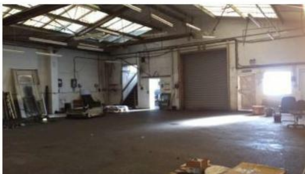
Internal parts full height building looking south
