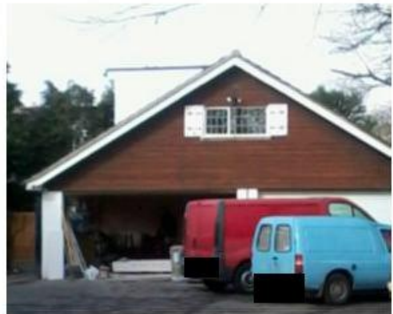
View of existing dormer from south
