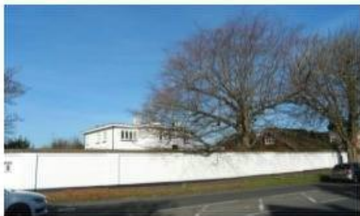
View of property boundary wall to the 'White House' in winter obscuring the ground floor of the garage with its roof seen above the wall.
